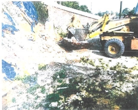
Figure 3.1 : Site clearing works (Source: Courtesy of JKRKT)
