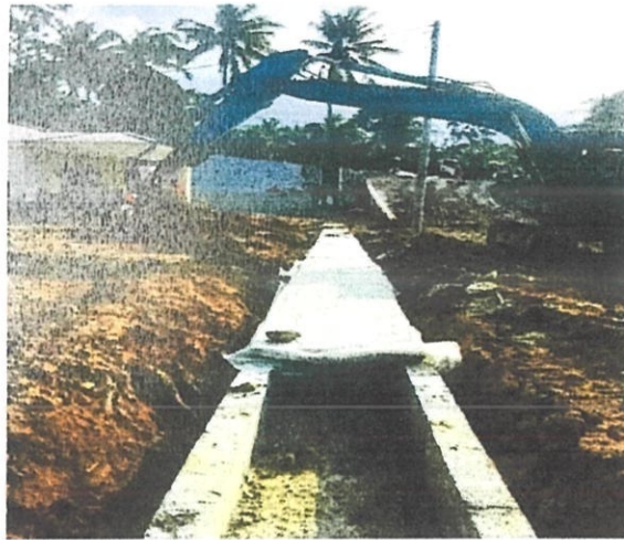
Figure 3.14 : Installation of toe drain (Source: Courtesy of JKRRKT)
