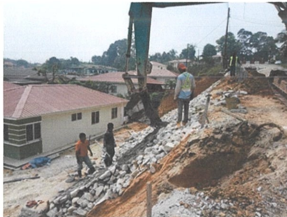
Figure 3.10 : Stone pitching works in progress
