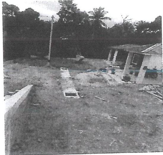
Backfilling works in progress
