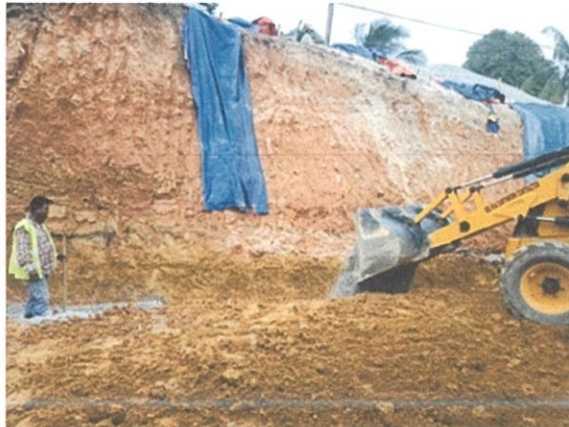
Figure 3.6 : Hardcore with the thickness of 300mm being poured
