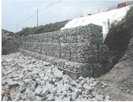
Figure 1.2 : Gabion Wall at Jln Felda Tenggara
