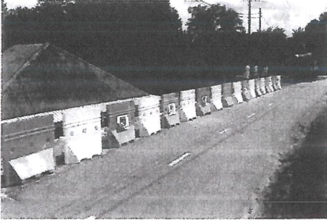
Plastic barrier and signage installation
