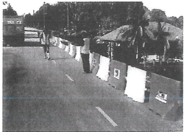
Plastic barrier and signage installation
