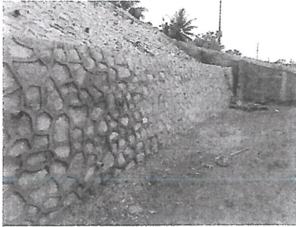
Stone Pitching works in progress
