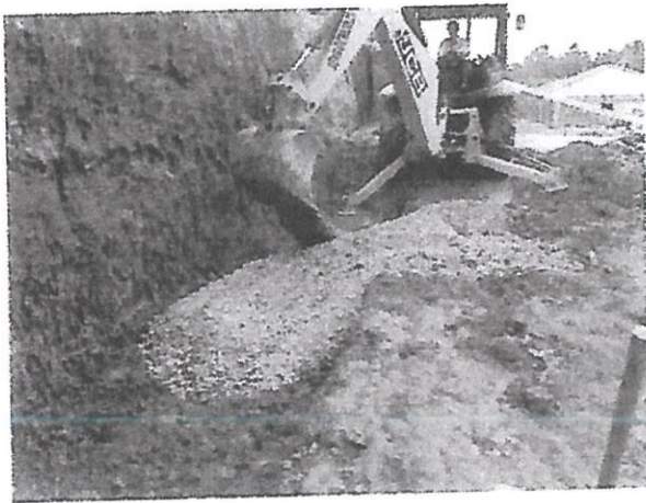
Base slab in progress
