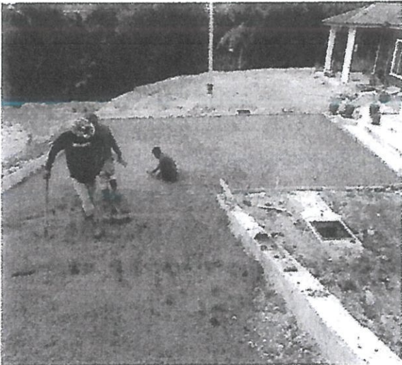
Base slab under progress
