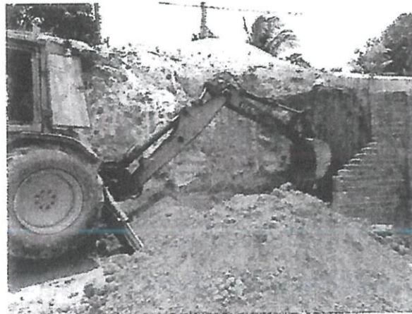
Site condition before start work
