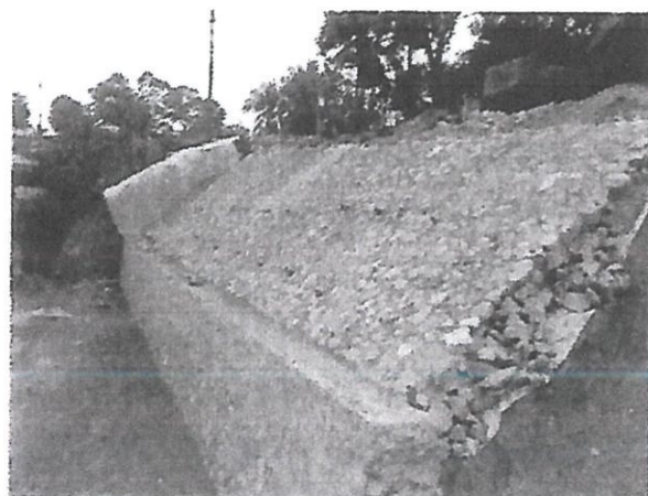
Stone Pitching works in progress
