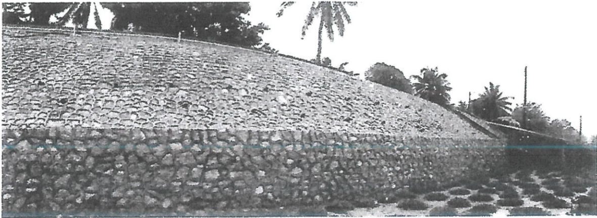
Stone Pitching and Rubble Wall 100% complete
