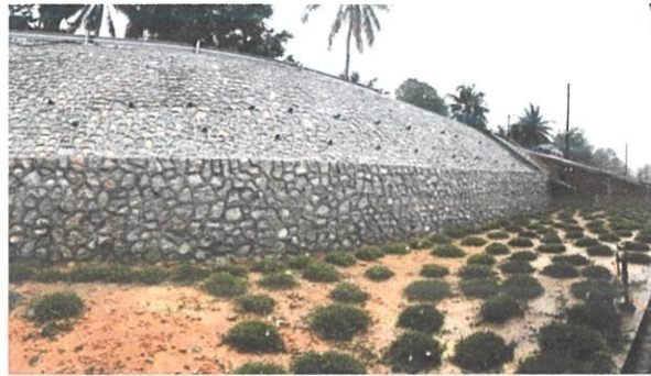
Figure 1.1 : Rubble Wall and Stone Pitching
