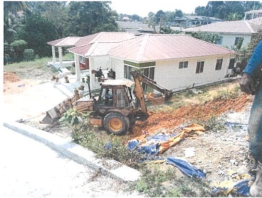
Figure 3.5 : Trench excavation for footing
