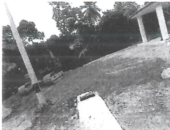
Toe drainage works completed
