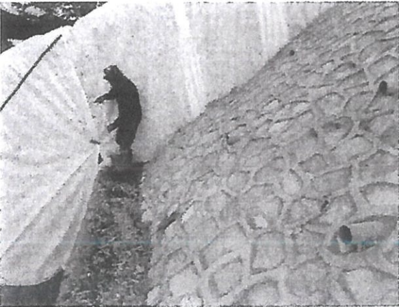
Stone Pitching works in progress
