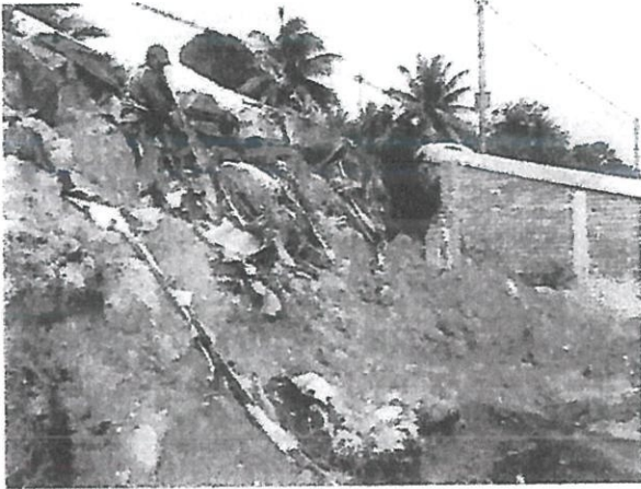
Site condition before start work
