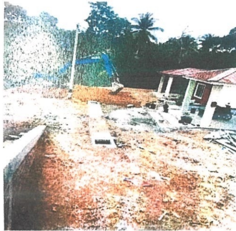
Figure 3.16 : Backfilling soil onto covered drains (Source: Courtesy of JKRKT)
