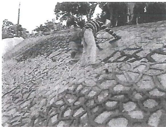
Stone Pitching works in progress
