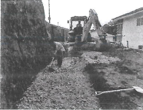
Crusher run backfill ongoing progress
