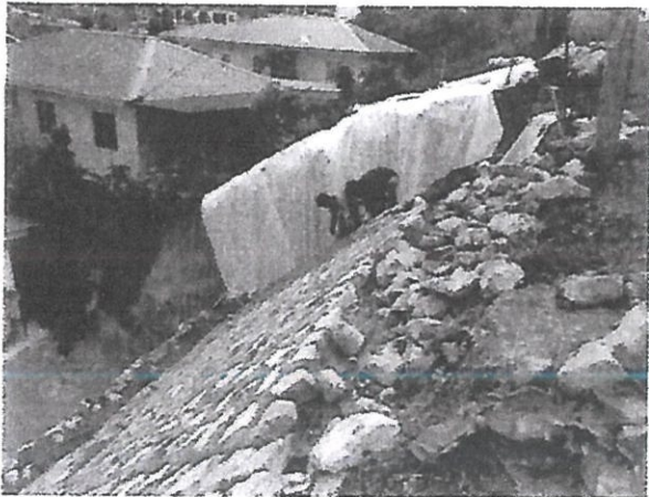
Stone Pitching works in progress
