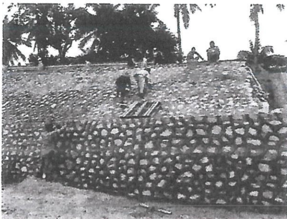
Stone Pitching works in progress
