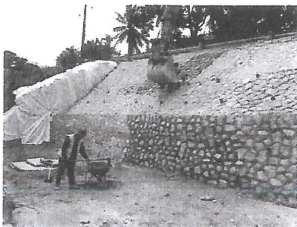
Stone Pitching works in progress
