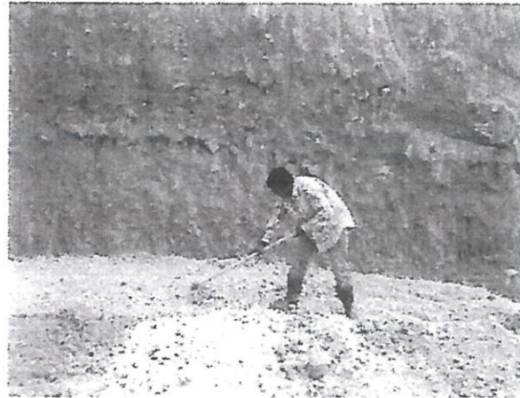
Crusher run backfill ongoing progress
