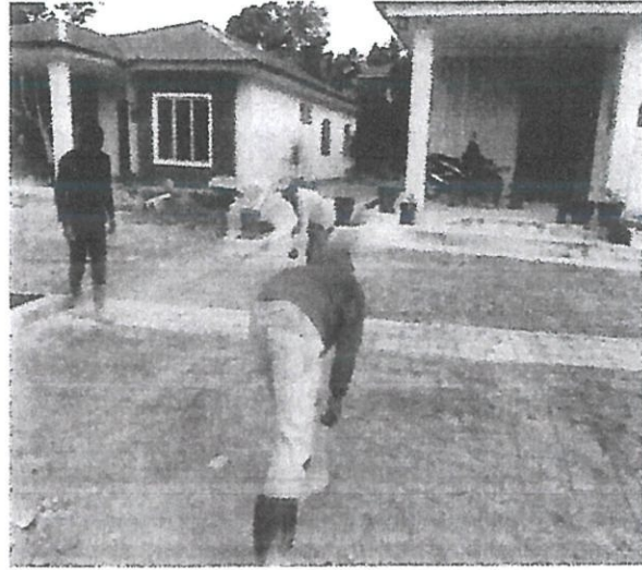
Base slab under progress
