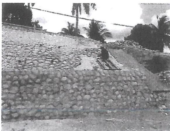
Stone Pitching works in progress
