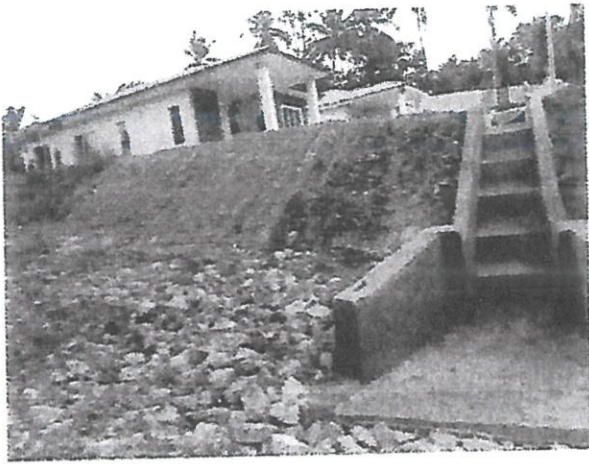
Cascade Drain and wingwall works in progress
