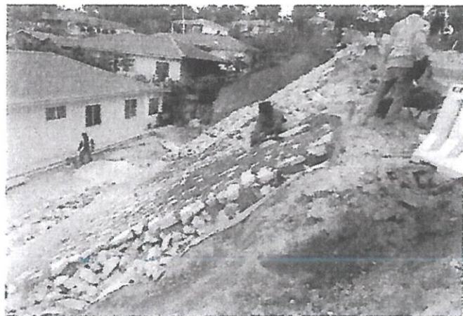
Stone Pitching works in progress
