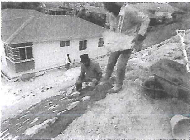
Stone Pitching works in progress
