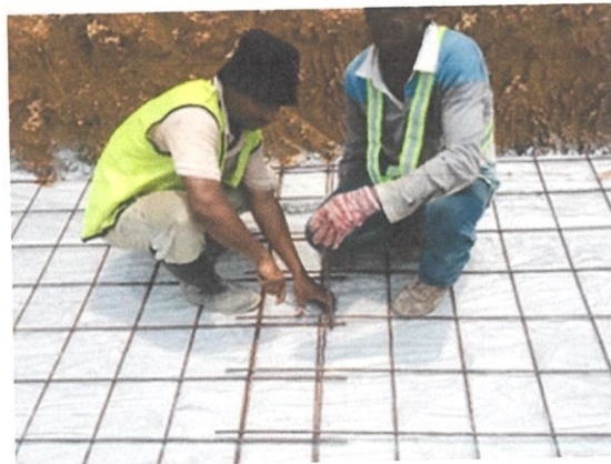
Figure 3.8 : Dowel bars being installed
