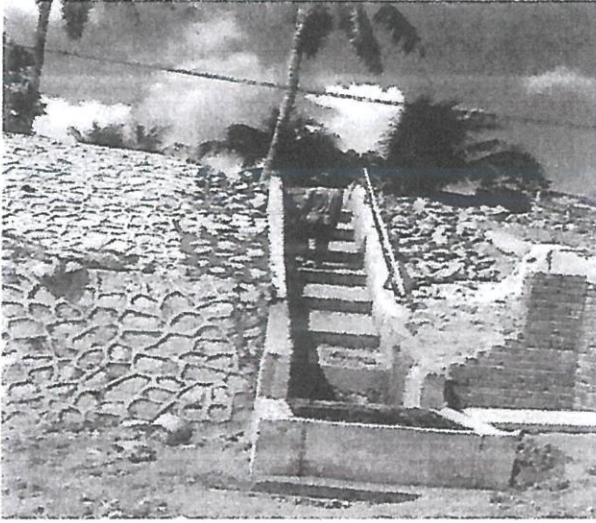
Stone Pitching works in progress
