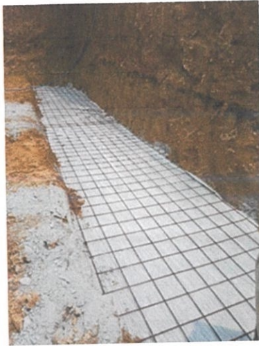
Figure 3.7 : BRC wire mesh steel
