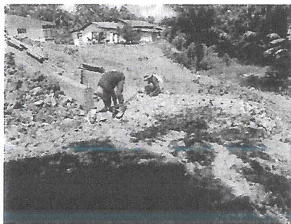
Gabion mattress installation
