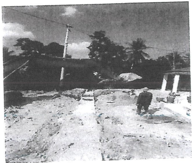
Backfilling works for toe drain
