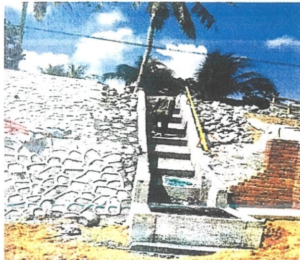
Figure 3.13 : Cascade drain construction in progress (Source: Courtesy of JKRKT)
