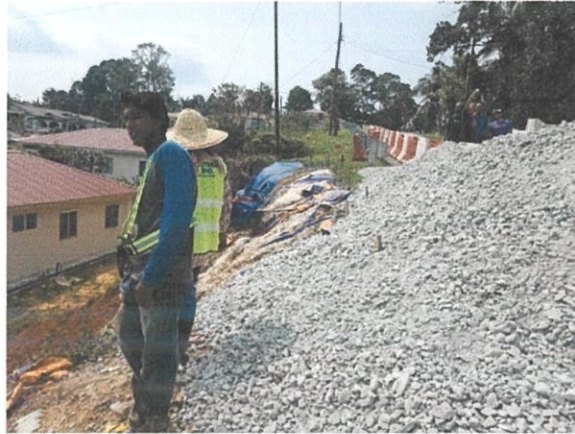
Figure 3.18 : Road above the slope
