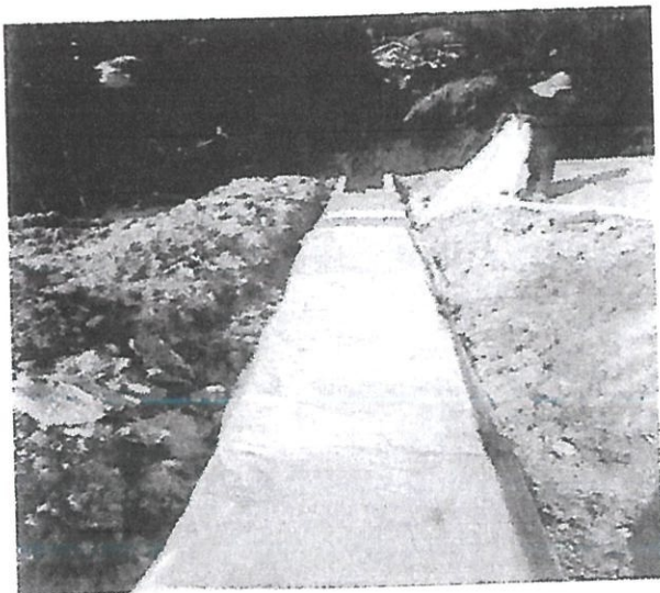
Geotextile installation works in progress
