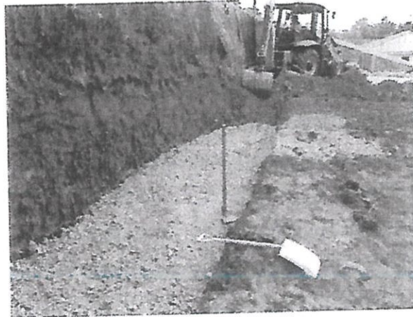
Base slab in progress
