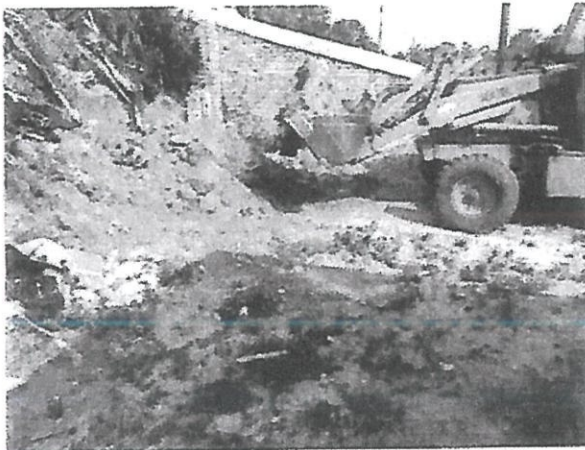
Site condition before start work
