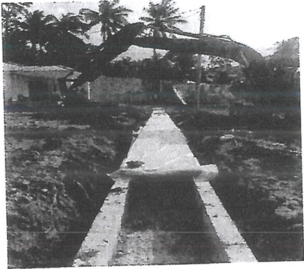
Toe drain works in progress, geotextile installation
