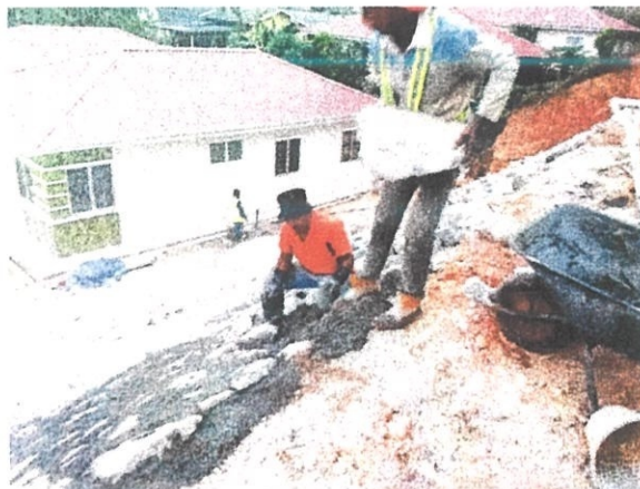
Figure 3.11 : Stone pitching works in process (Source: Courtesy of JKRKT)
