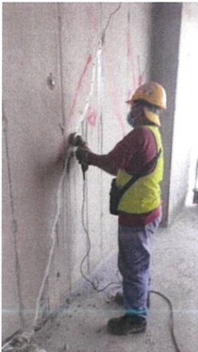
Figure 3.4.2 h) Remove Packer and Seal
