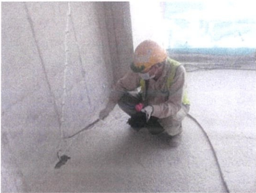
Figure 3.4.2 g) Injection work
