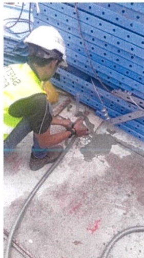
Figure 3.4.2 d) Injection work
