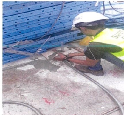
Figure 3.4.1 b): pressure grout process
