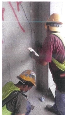
Figure 3.4.2 b) Patch up work using sika grout 215
