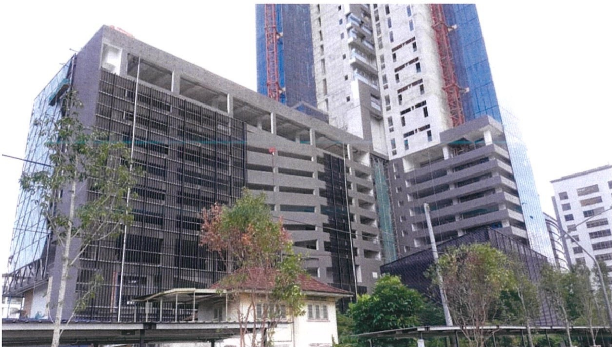
Figure 3.1.2: View of podium
