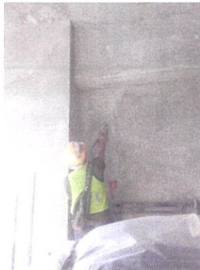
Figure 3.4.2 a) Cutting V-Cut using grinder
