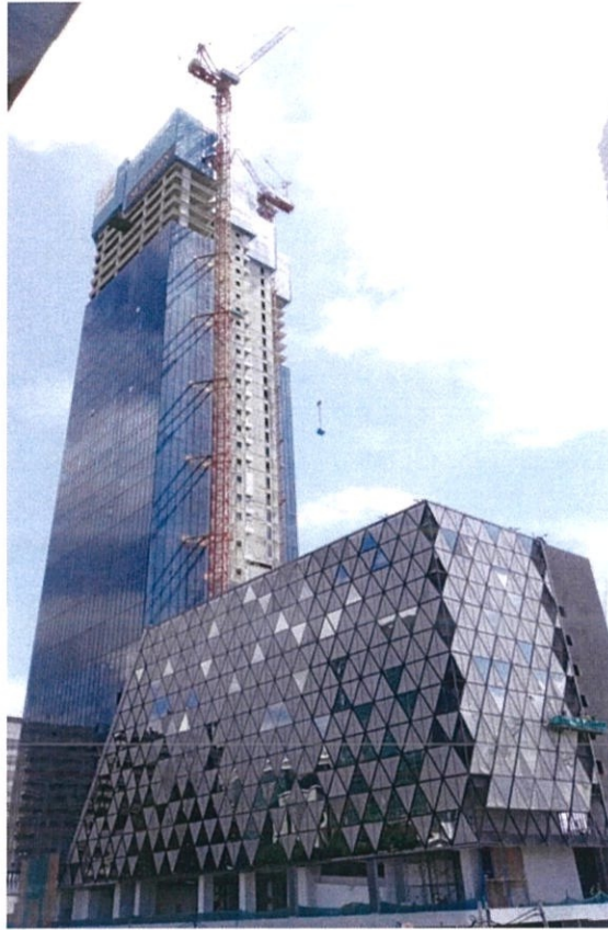
Figure 3.1.1: View of the building construction
