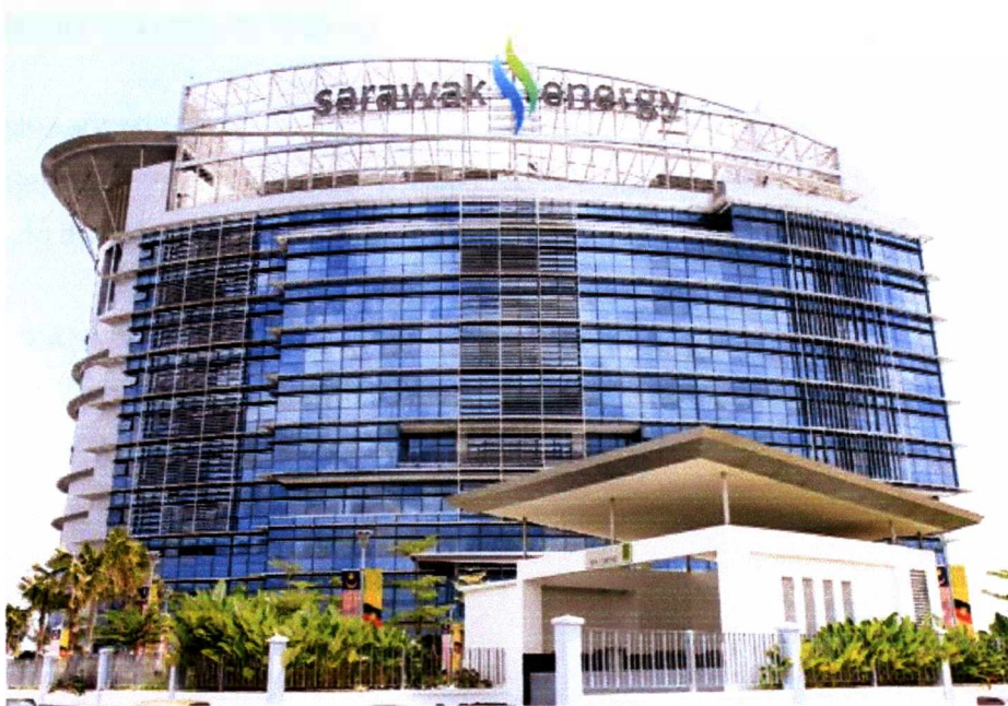
Figure 1.1 Sarawak Energy Berhad headquarters in Kuching (Source: https://www.theborneopost.com )
