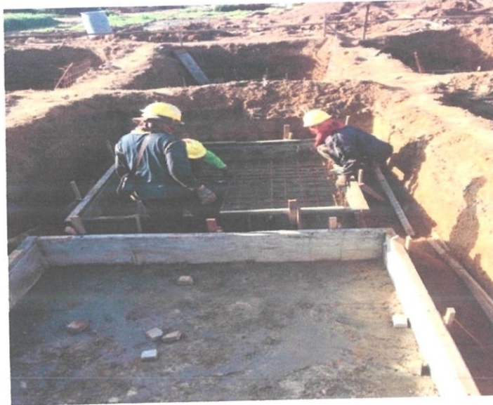
Photo 1.7 The Installaion of Formwork For Footing
