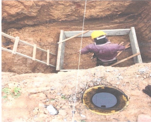
Photo 1.5 Set up the location of formwork
