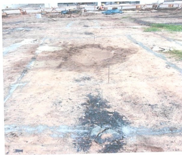
Photo 1.2 The Marking and Pegging Process
