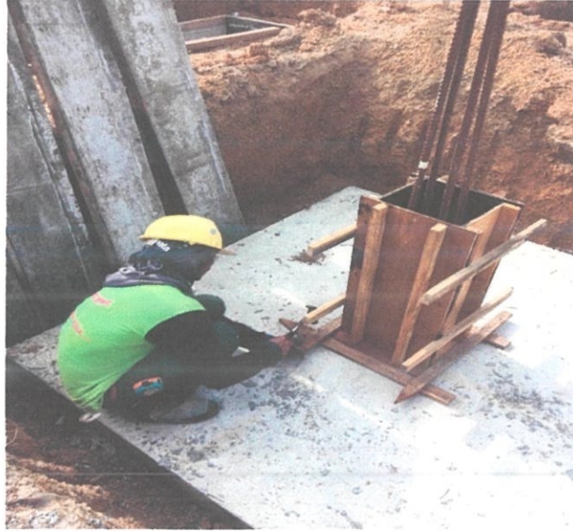
Photo 1.11 The installation formwork for stump
