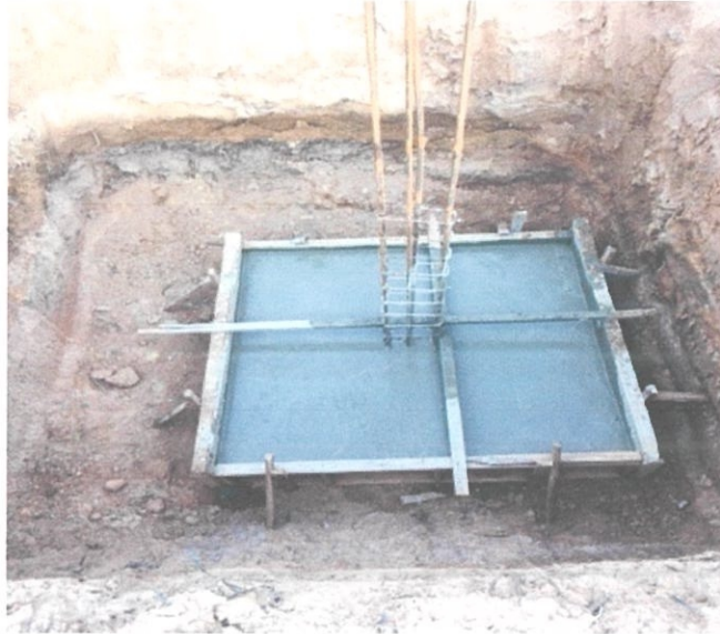
Photo 1.10 The concreting of pad footing
