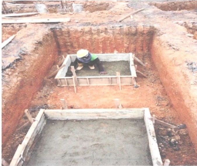
Photo 1.6 Laid a Cement Plus Sand as Lean Concrete.
