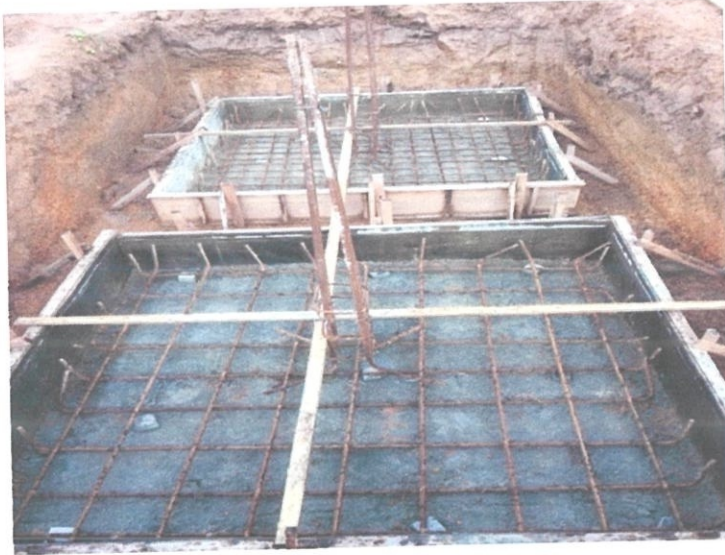
Photo 1.9 The installation of reinforcement
