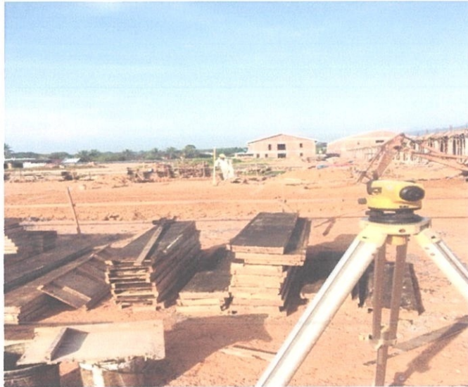
Photo 1.4 Levelling the Excavated Hole
