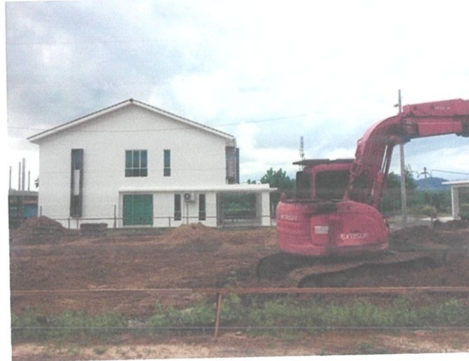
Photo 1.3 The Excavation of Soil
