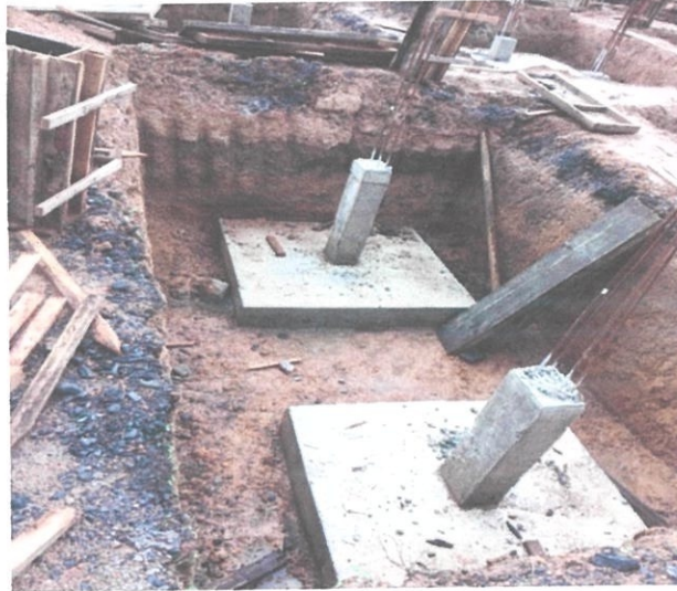
Photo 1.13 The dismantle of formwork.
