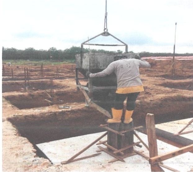
Photo 1.12 The concreting of stump.
