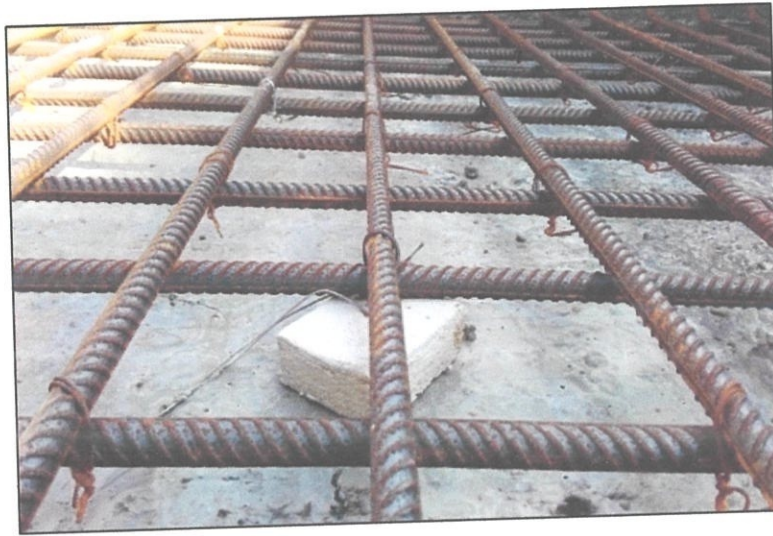
Photo 1.8 The Installation of Spacer Block.
