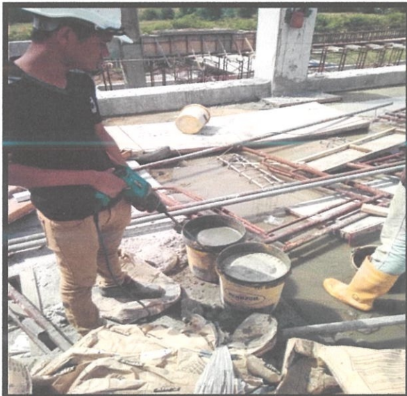
Picture 3.3.1(vi) Prepare NSG cement
