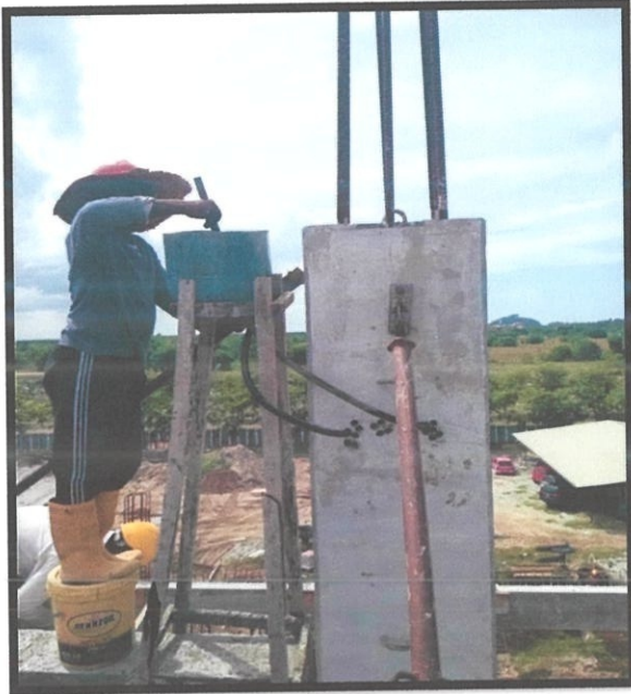
Picture 3.3.1(vi) Grouting process
