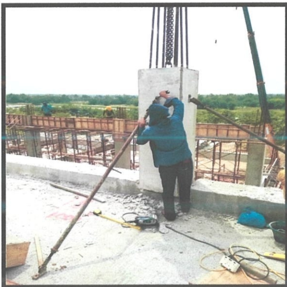
Picture 3.3.1(iv) Installation of prop
