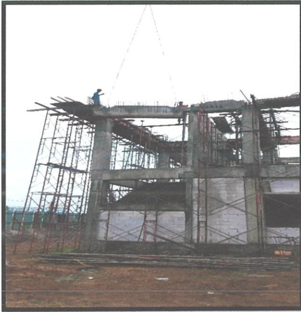
Picture 3.3.2(ii) Lift and install work beam
