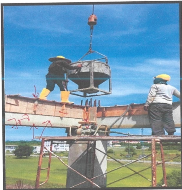
Picture 3.3.2(v) Casting joints between beam and column
