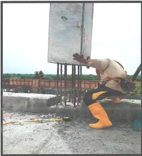
Picture 3.3.1(iii) Installation of precast column
