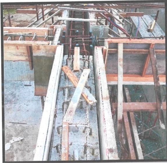
Picture 3.3.2(iv) Rebar the joints between beam and column
