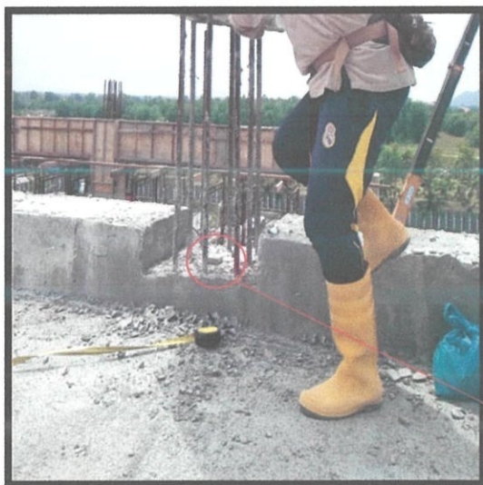
Picture 3.3.1(ii) Put shim pad on slab
