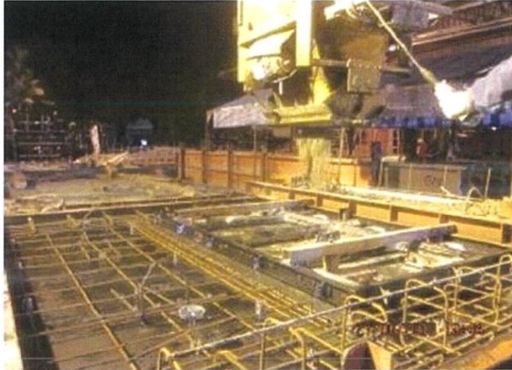
Figure 3.20: Pouring concrete Grade 30 into moulding.
