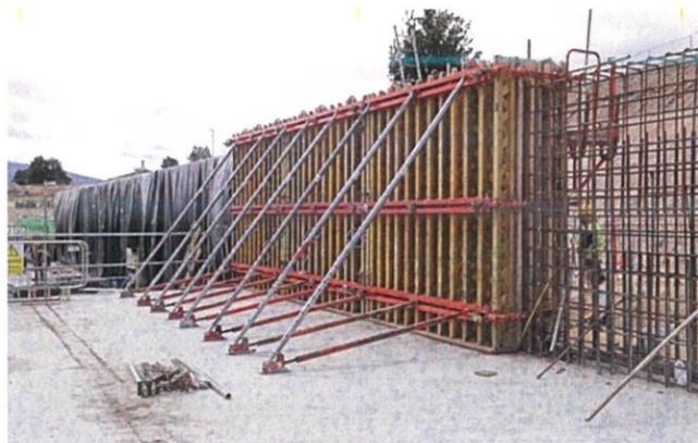
Figure 3.1 : Steel Formwork in use to cast concrete wall
