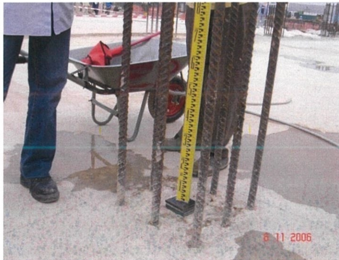
Figure 3.25: Installing shim plate.
