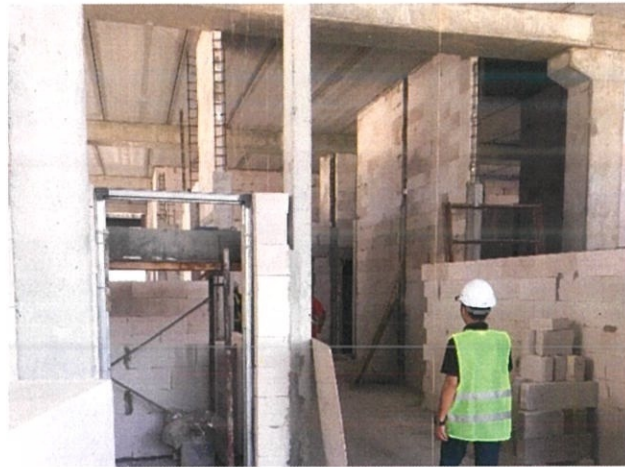
Figure 3.5: 100mm Block used for partition wall
