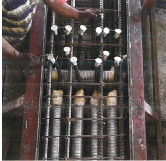
Figure 3.18: Workers inserting flexi hose in between the rebar.
