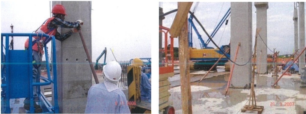
Figure 3.34: Minimum 2 props per each column are installed.
