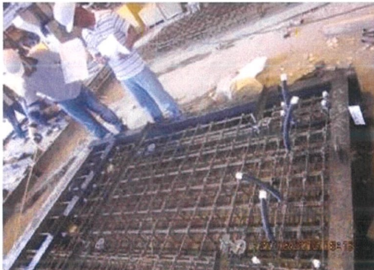
Figure 3.19: Engineers inspecting the rebar before concreting works.
