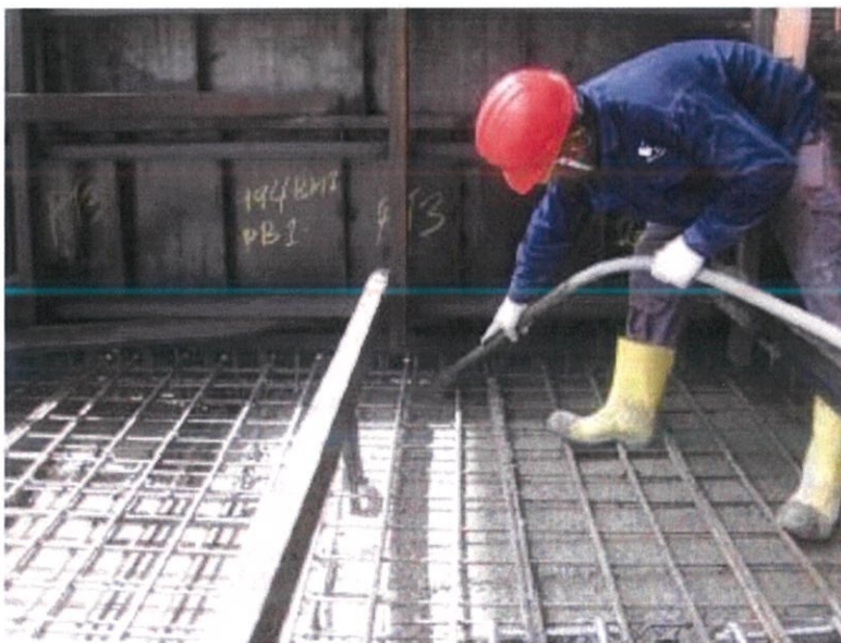
Figure 3.21: Vibrating to ensure a balance and evenly spread concrete.
