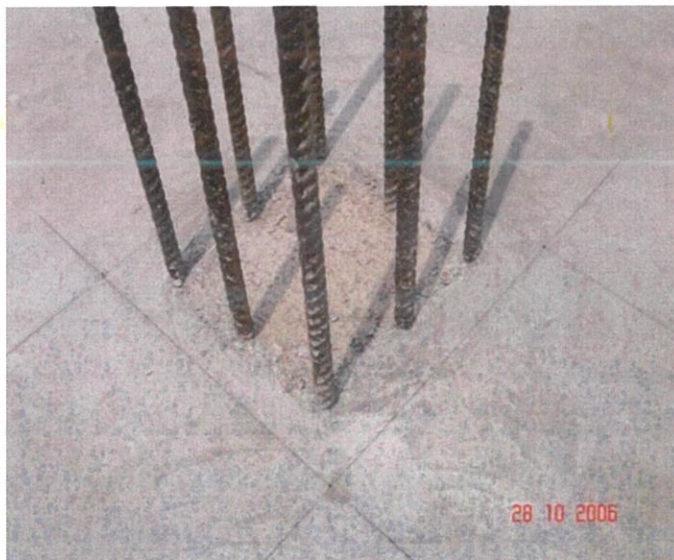
Figure 3.27: Column setting out.
