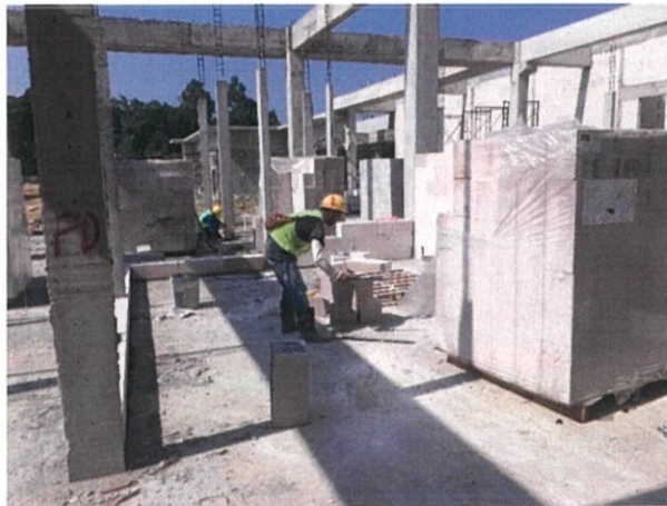
Figure 3.4: A workers handling Starken AAC Block
