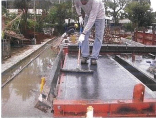
Figure 3.16: Applying lubricating oil onto the mould surface.
