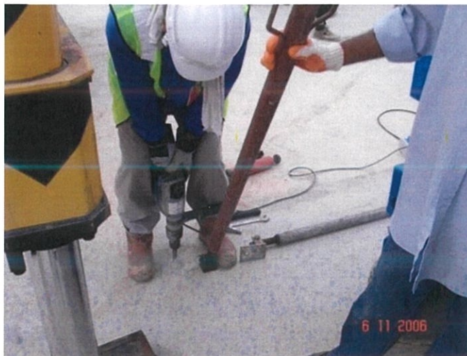
Figure 3.32: A workers drilling ole to fix the props.
