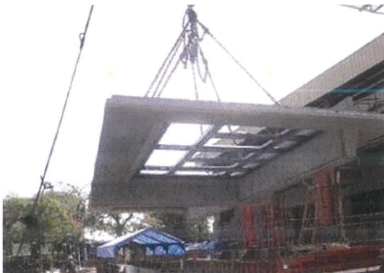
Figure 3.22: A finish panel can be raised up from the moulding to be stored before installation.
