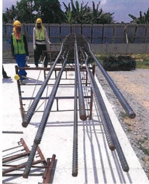
Figure 3.14: Rebar laid to be tied to engineer specification.
