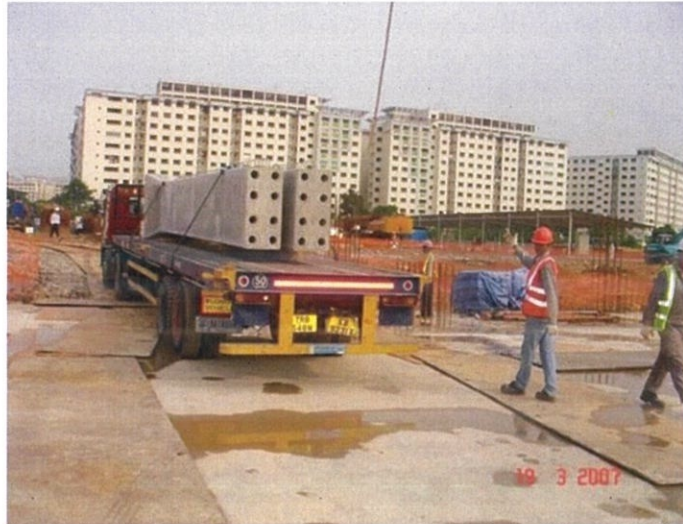
Figure 3.29: Column move closer to installation point.
