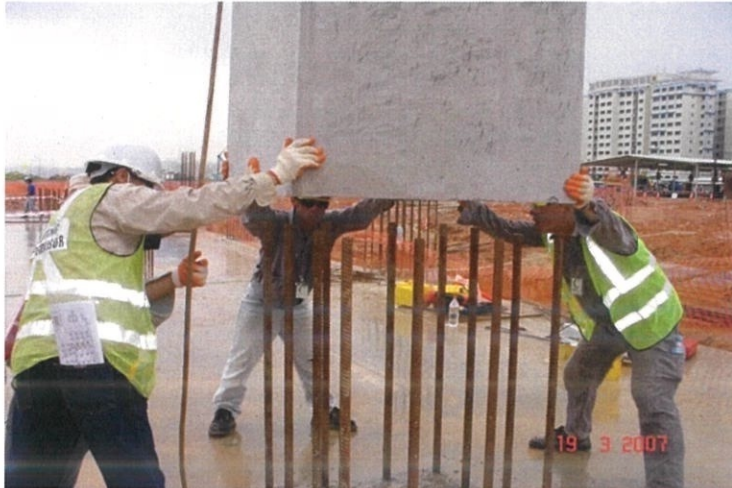
Figure 3.31: Three workers calibrating column onto starter bar.
