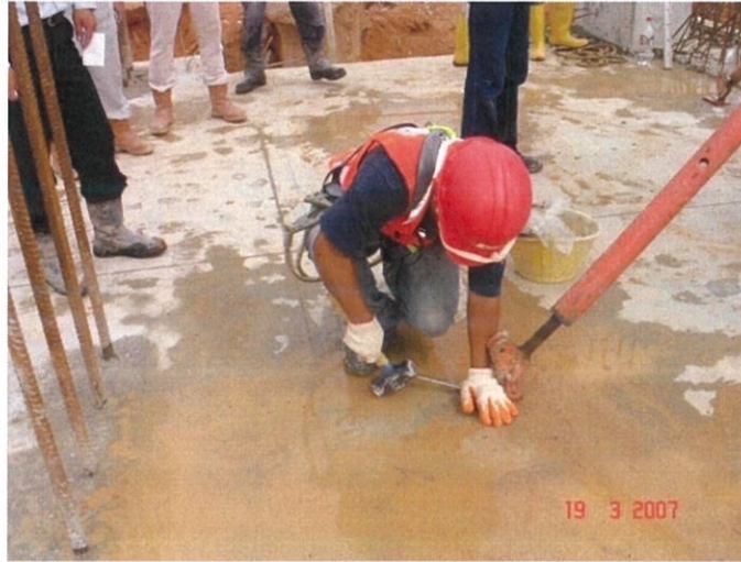
Figure 3.33: Props are tied to slab/base using bolts and nuts.
