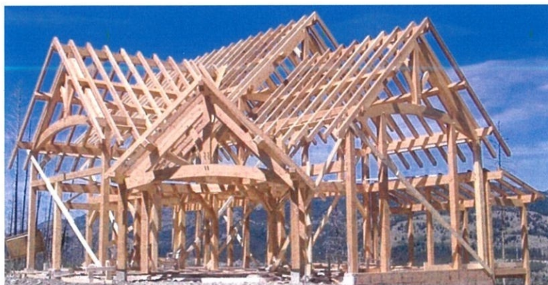
Figure 3.3: Single Storey house build by using timber framing system
