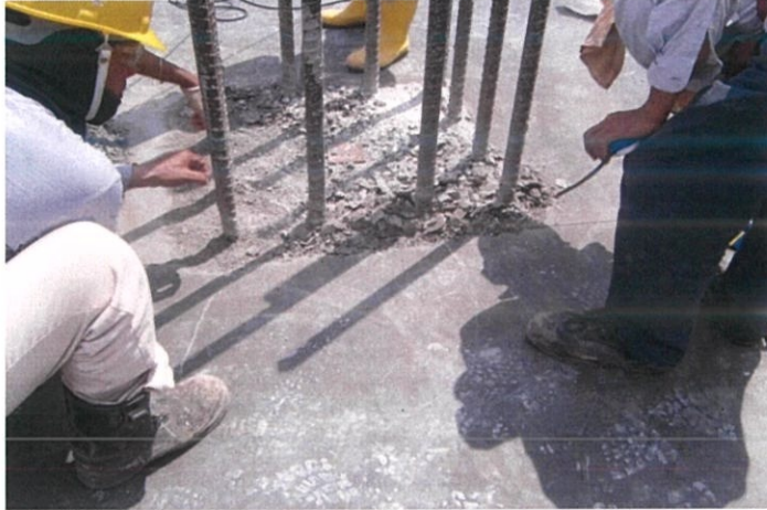
Figure 3.26: Exceeding concrete hacked to level base.
