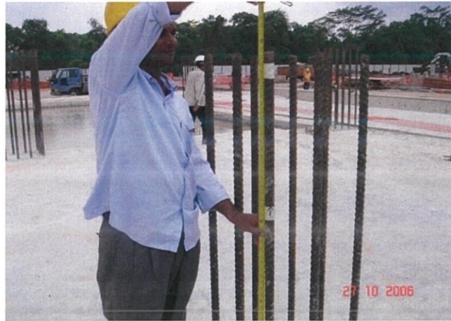
Figure 3.24: Measuring height using tape.
