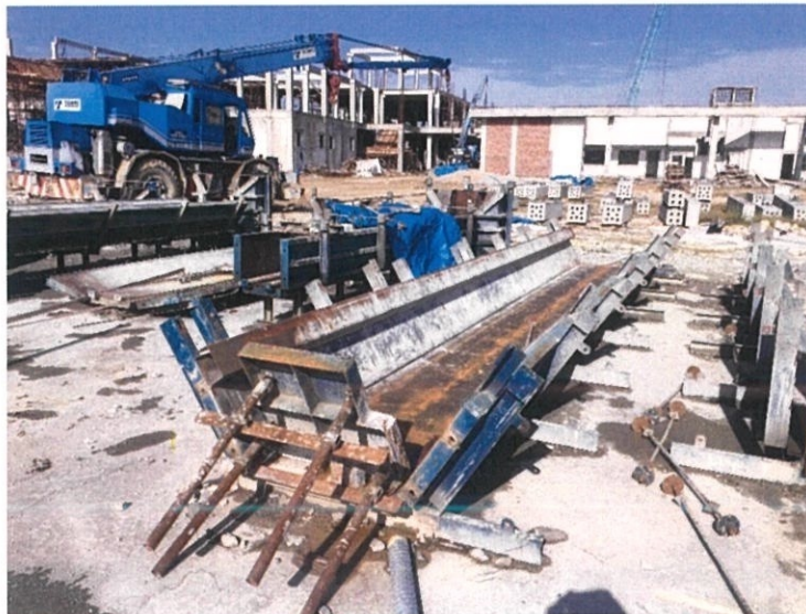
Figure 3.13: Precast Column Steel Moulding
