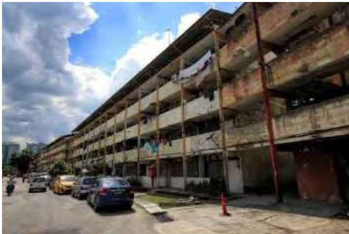
Figure 2: External condition of Waller Court
