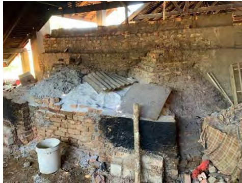
Figure 6: The Chamber Kiln used to do Firing Proses (Field Observation, 2021)
