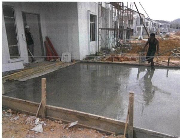
Figure 3.30: Concreting.
