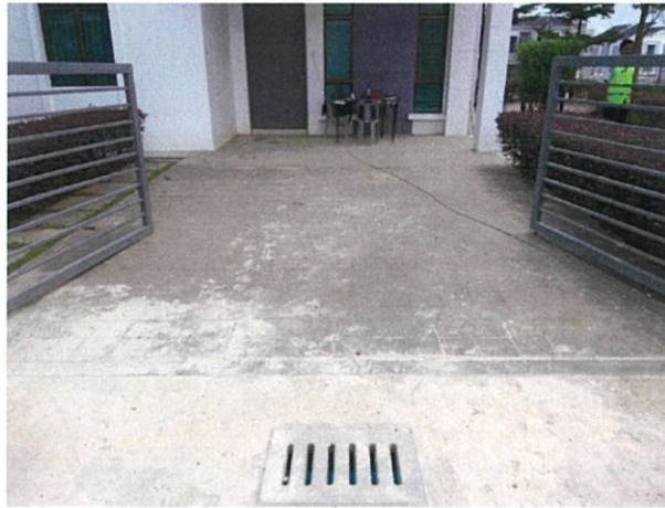
Figure 1.1: Finished Driveway from sample house.
