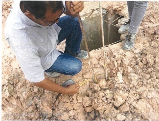
Figure 3.9: Setting out pegs.
