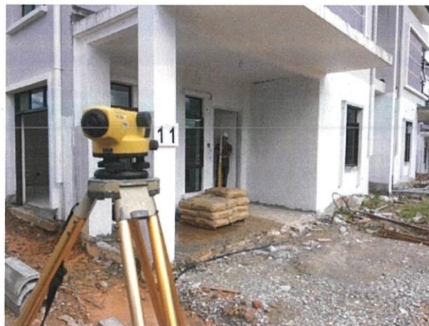
Figure 3.10: Levelling Floor level.
