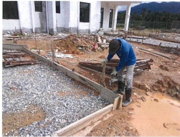
Figure 3.14: Installation of formwork.
