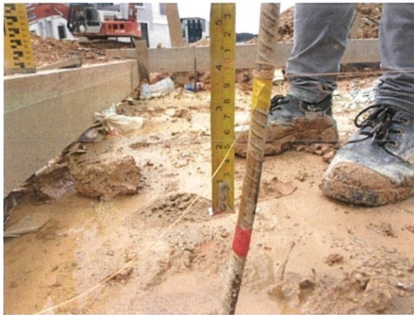
Figure 3.21: String tied to point "3b".
