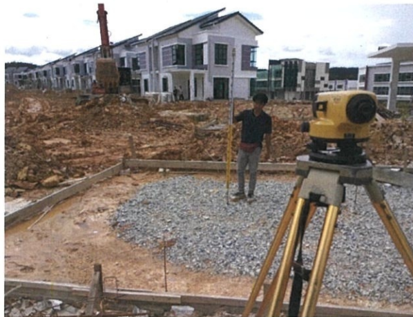
Figure 3.24: Levelling point "2b".
