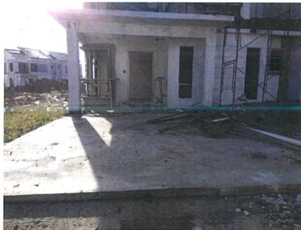
Figure 3.31: Cured concrete.
