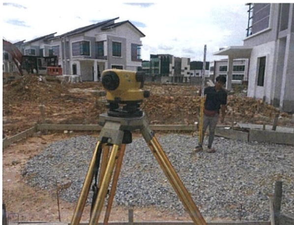
Figure 3.25: Levelling point "1b".
