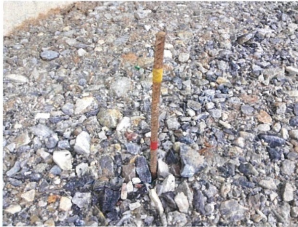
Figure 3.18: Yellow tape (Concrete) & Red tape (Crusher Run)
