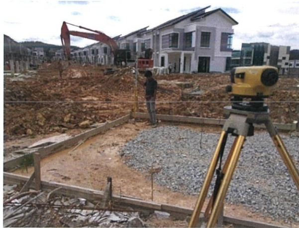
Figure 3.19: Transferring level data of point "3b" at point "3a" & "3c".
