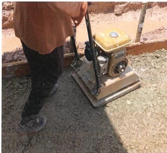
Figure 3.27: Plate Compaction.
