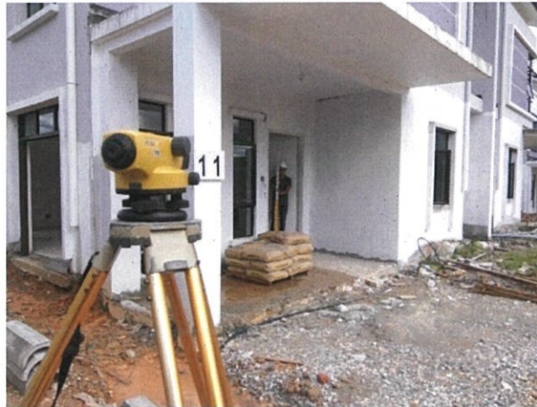
Figure 3.16: Levelling Floor level.
