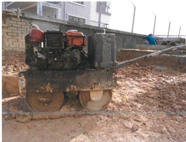
Figure 3.13: Mini Road Roller compaction.
