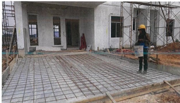
Figure 3.29: Waterproofing sheet and BRC wire mesh.
