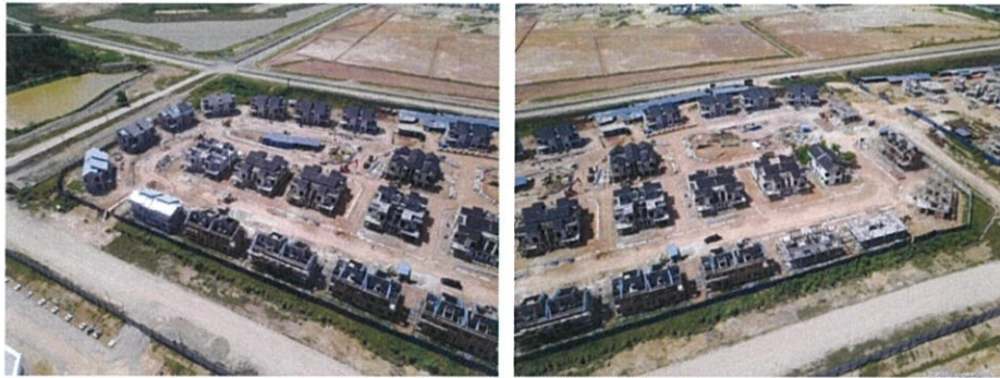
Figure 3.3 & 3.4: Sky view of site. (Source: Courtesy of IMSB)
