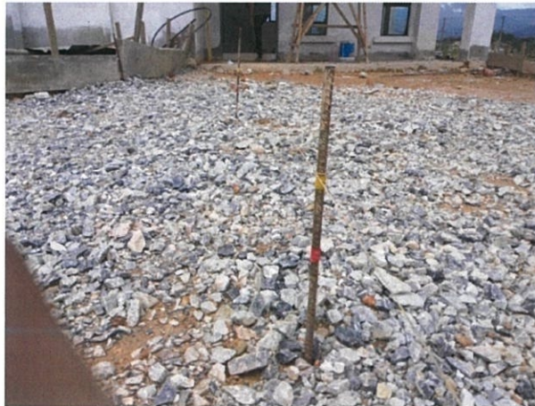
Figure 3.23: Markings for middle pegs, points "2b" & "1b".
