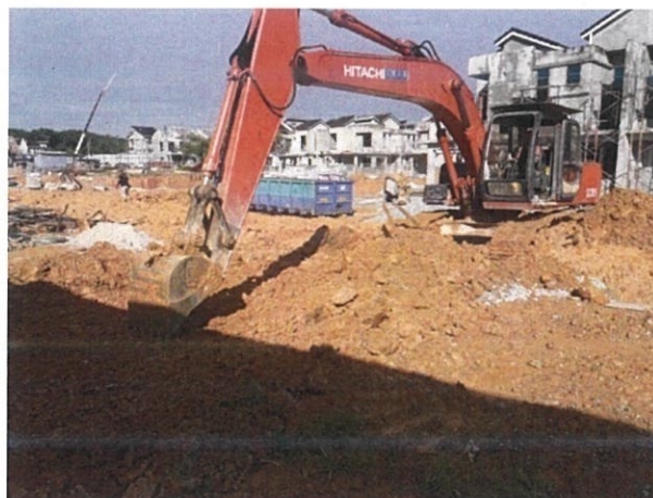
Figure 3.11: Excavating driveway.
