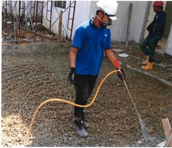
Figure 3.28: Spraying anti-termite.
