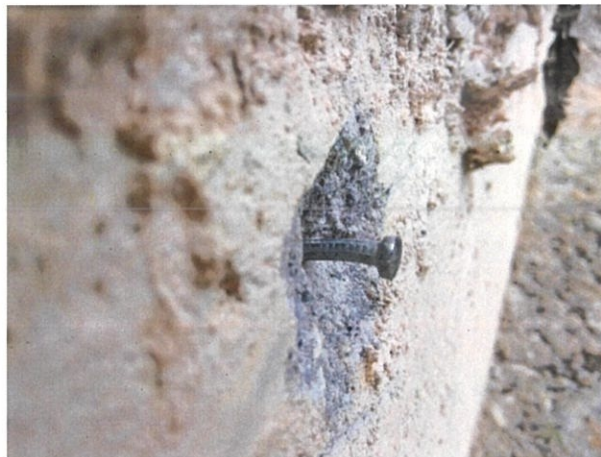
Figure 3.17: Marking drop level of Porch.
