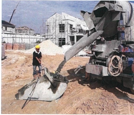
Figure 3.50: Grade 20 & Grade 15 Concrete.
