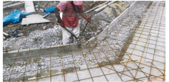
Figure 12: Cutting over reinforcements
