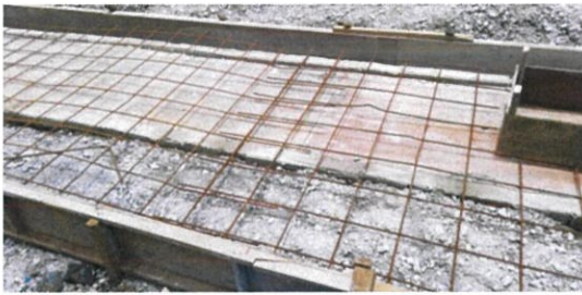
Figure 14: Overlapped reinforcements
