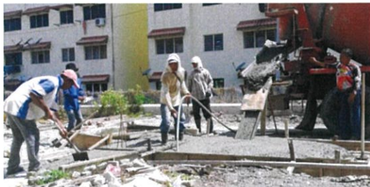
Figure 16: Concrete pouring and vibrating
