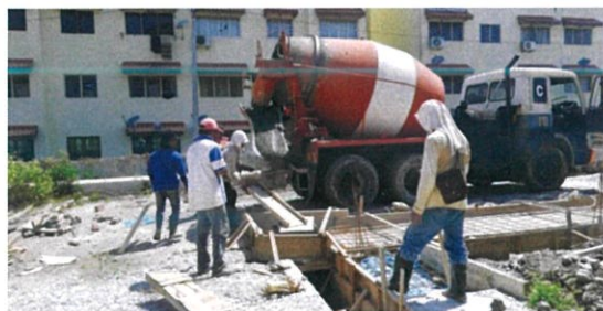
Figure 17: Concrete mixer truck
