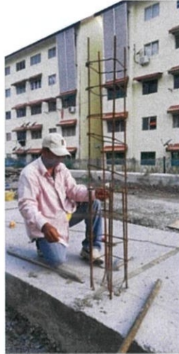
Figure 19: Installation of column reinforcement
