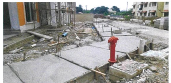
Figure 15: Curing process of concrete
