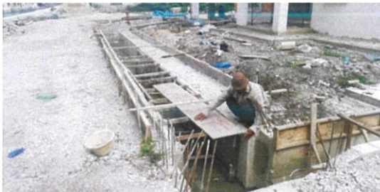
Figure 11: Formwork installation
