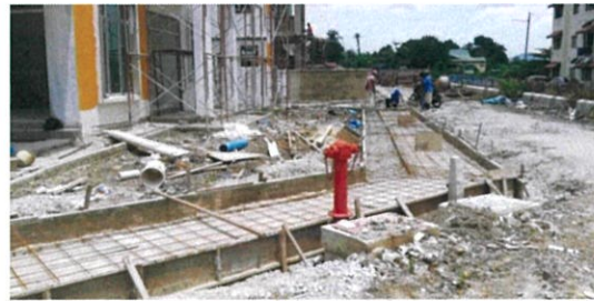
Figure 13: Reinforcements installation
