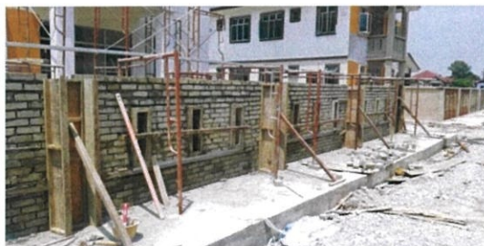
Figure 25: Column formworks
