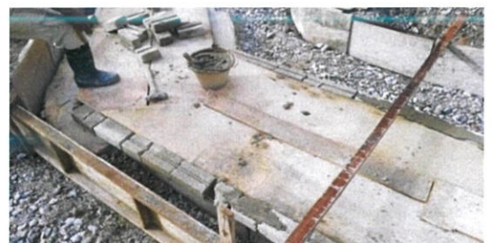
Figure 10: Formwork installation
