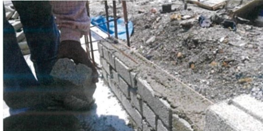
Figure 23: Reinforcement every 3 layers
