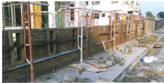
Figure 24: Laying of frames
