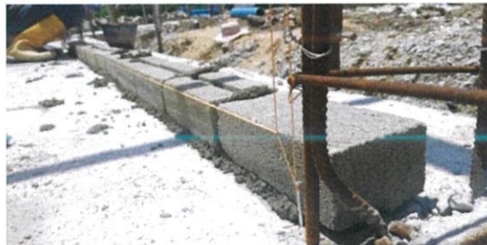
Figure 20: Thread as guideline
