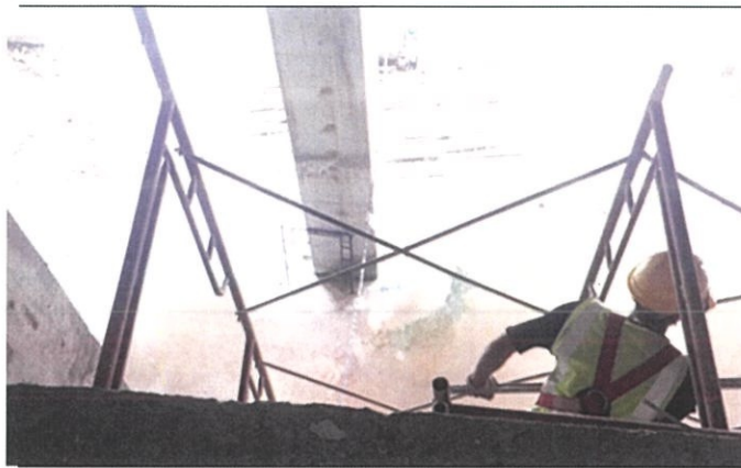
Figure 3.13: The installation of scaffold
