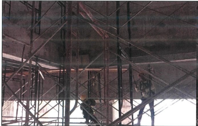
Figure 3.23: carpenter dismantled the formwork
