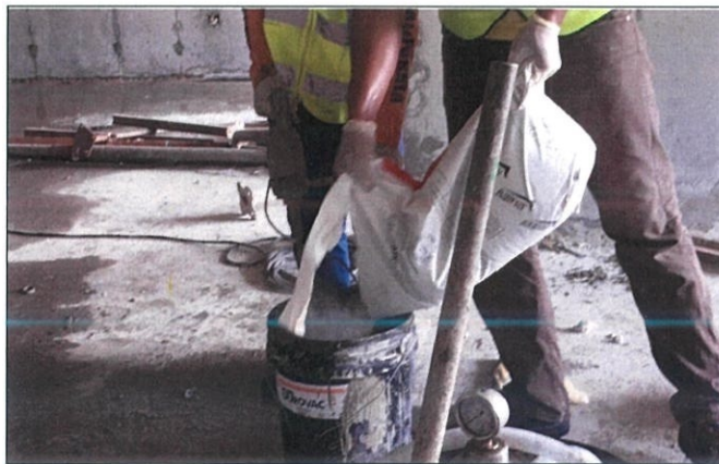
Figure 3.30: mixing the non-shrink grout
