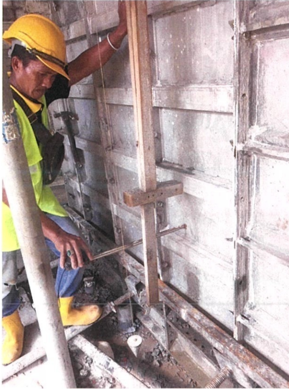
Figure 4.3: verticality inspection on formwork installation
