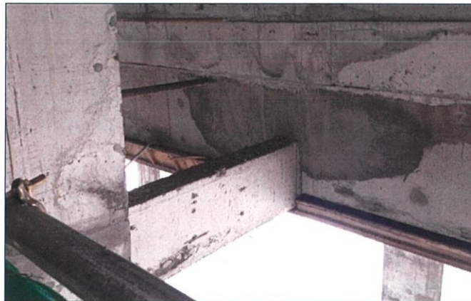
Figure 3.19: The installation of beam form
