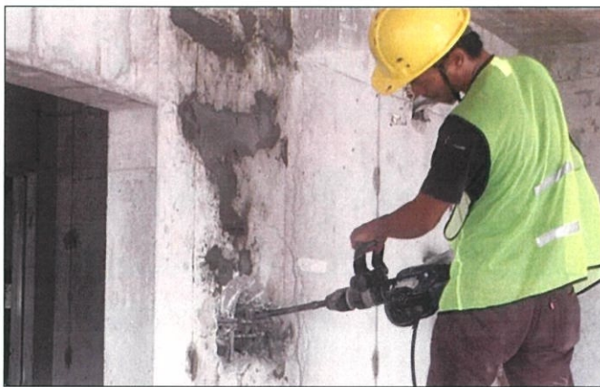
Figure 3.25: Hacking wall in process
