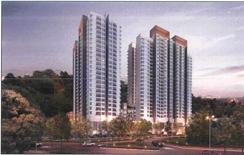
Figure 3.1 : Riana South at Cheras, Kuala Lumpur
