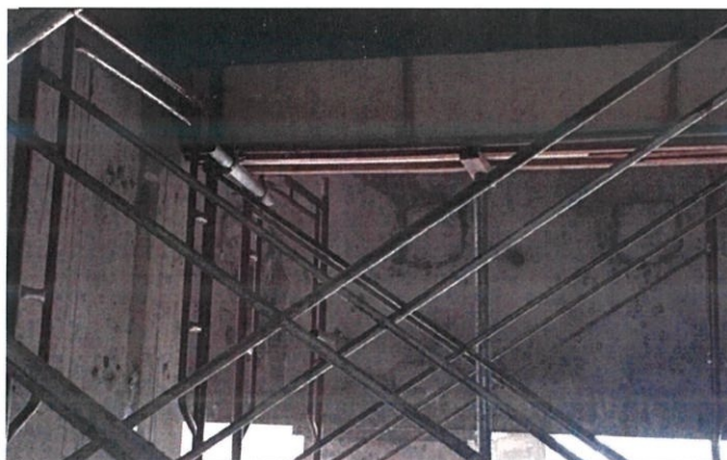
Figure 3.20: The installation of props and strut
