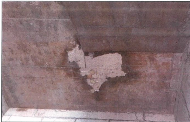
Figure 3.11 : Example of finishing Error.
