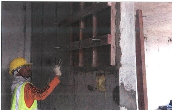
Figure 3.28: All the gap are sealed
