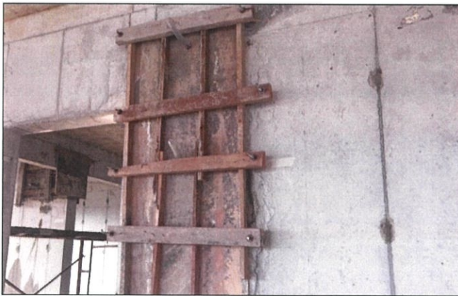
Figure 3.27: formwork is installed
