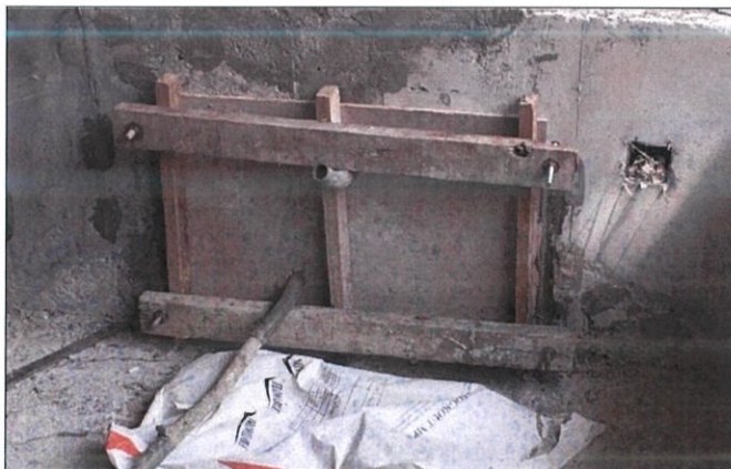
Figure 3.34: non-shrink grout is pumped into formwork
