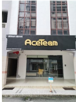
Figure 2: AceTeam Office at Damansara Intan
