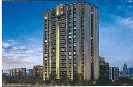
Figure 3.2: Aira Residence Tower B side view
