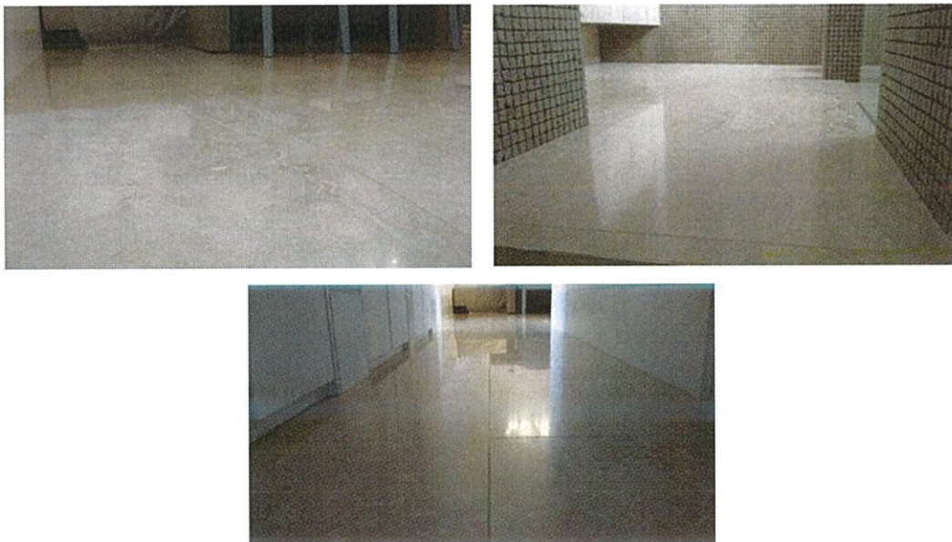
Figure 3.4: Marble floor finishes
