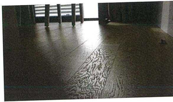
Figure 3.8: Engineered Timber Floor
