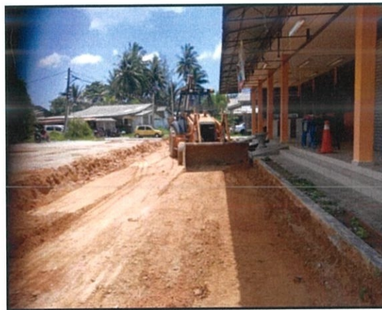
Figure 3.28: Remove and replace soil before lay the crusher run
