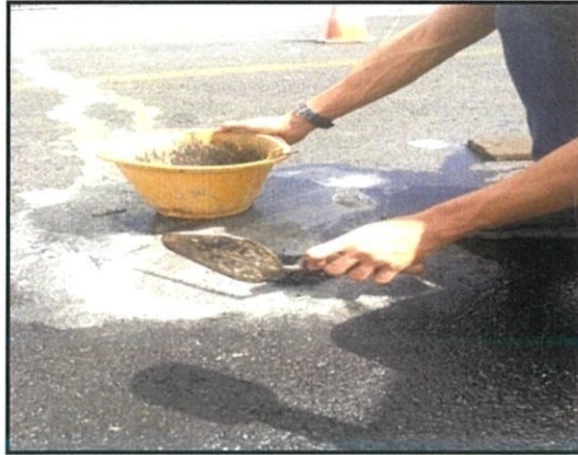
Figure 3.22: The core hole was restored by new asphalt
