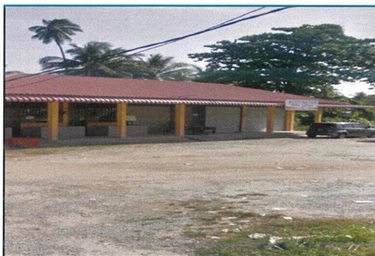
Figure 3.3: Location for road construction before starting the project
