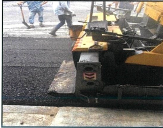
Figure 3.18: Process of laying asphalt concrete binder after prime coat
