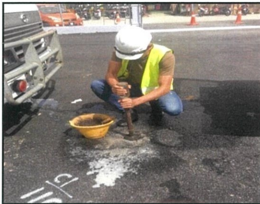
Figure 3.23: Compact the asphalt using hammer compactor at C1 point
