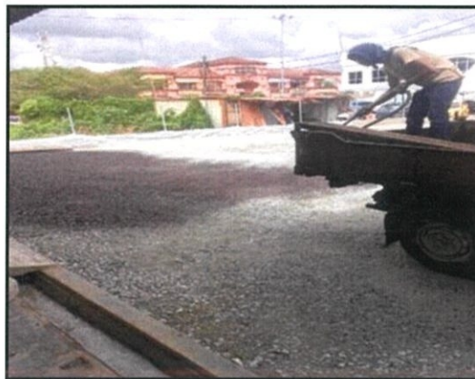
Figure 3.16: process of spraying bituminous prime coat on crusher run
