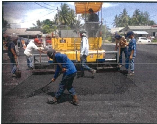
Figure 3.19: Process of laying asphaltic concrete wearing course
