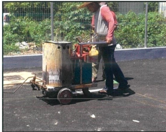
Figure 3.26: Process of road marking
