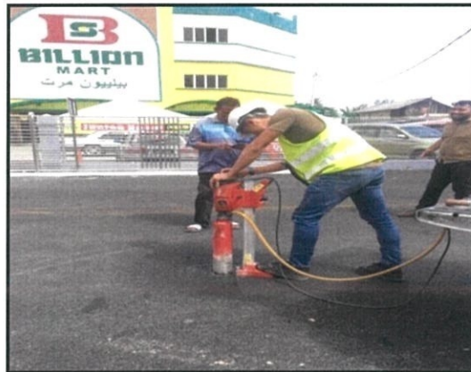
Figure 3.20: Core drilling machine was used during coring process
