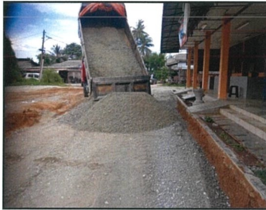
Figure 3.15: process of laying crusher run on the surface
