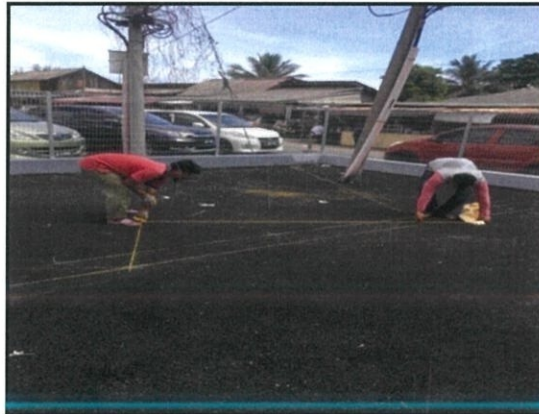
Figure 3.25: Workers locate and marks the line using yellow chalk
