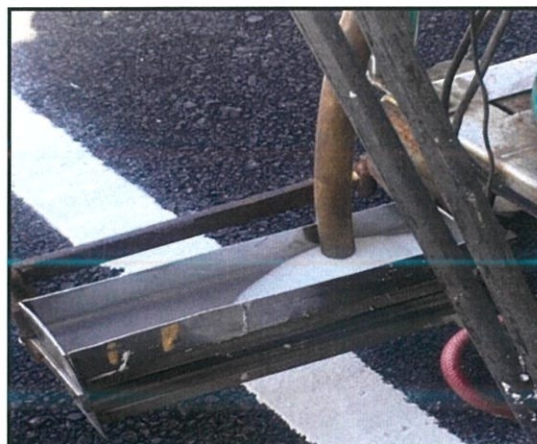
Figure 3.27: Glass powder is also sprinkled on the line
