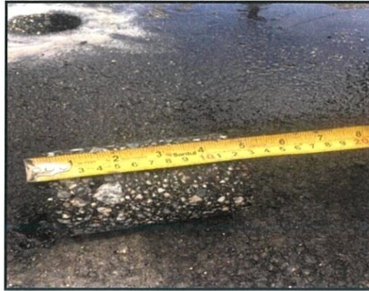
Figure 3.21: Measuring the thickness of asphaltic concrete
