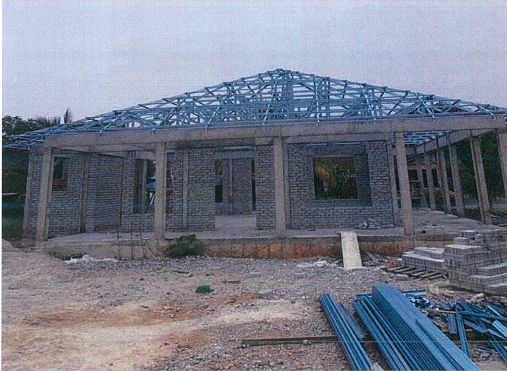
Figure 3.2 Current progress of the project (roofing)
