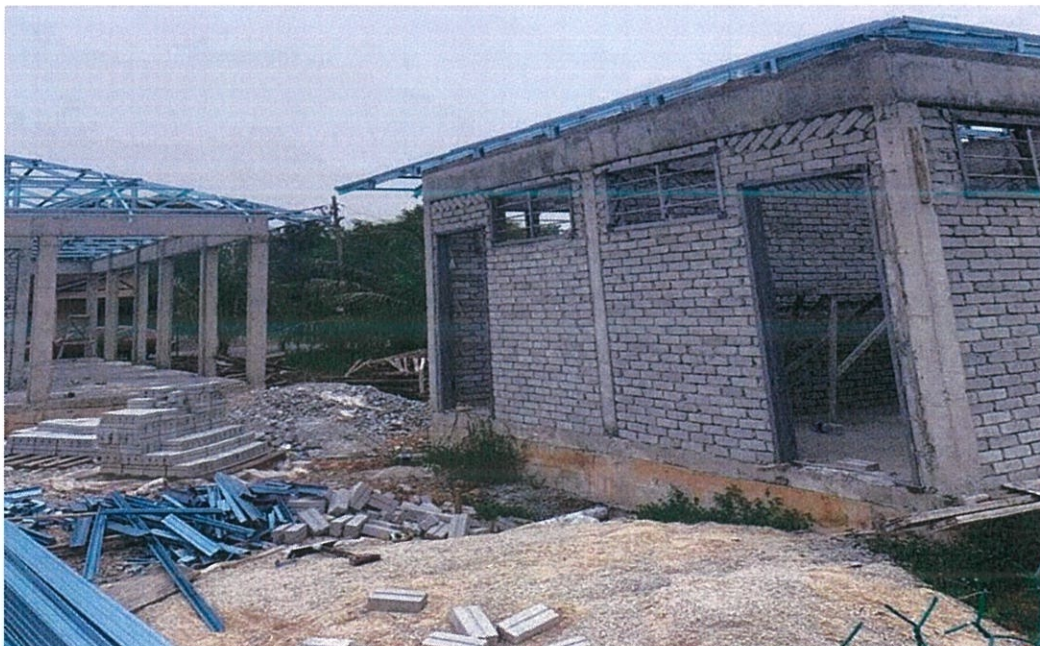
Figure 3.3 Current progress of the project (door and window)
