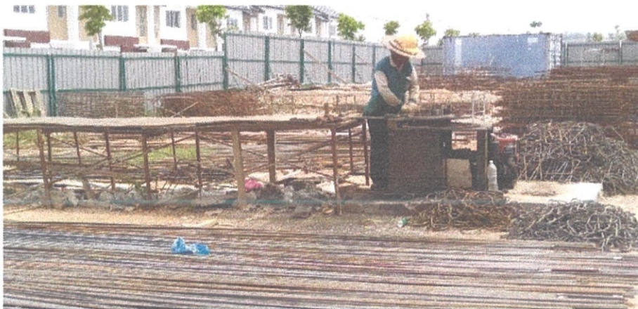
Figure 3.16 Preparation for steel bar
