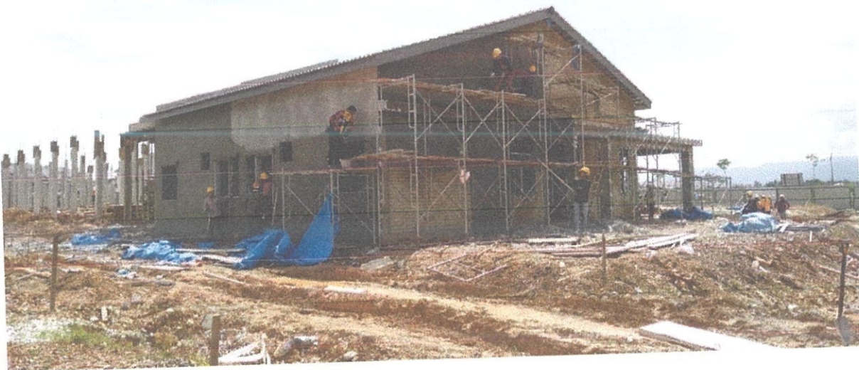
Rear view of 185-unit Single Storey Terrace House Phase 6 Figure 3.5
