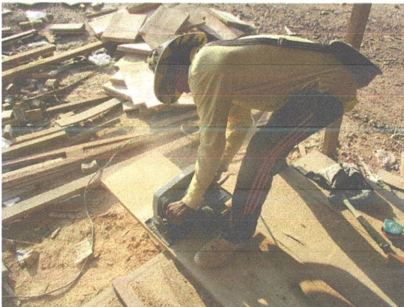
Figure 3.11 Preparation for formwork
