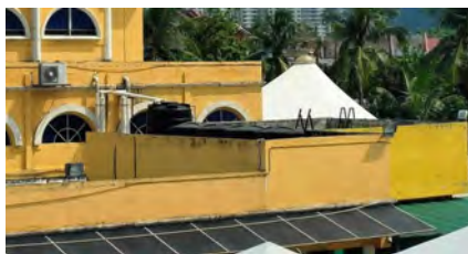
Figure 6: Rainwater Harvesting's Tank at Al-Muttaqin Mosque
