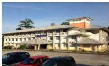
Figure 7: FSPU Annex 3 (BS)
