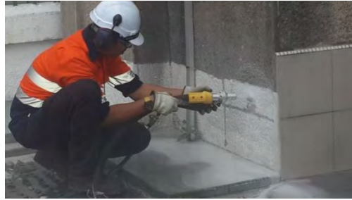
Figure 3: Process of cleaning the fair faced façade using armex soda.
