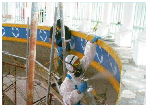
Figure 8: Process of applying the protective layer coating
