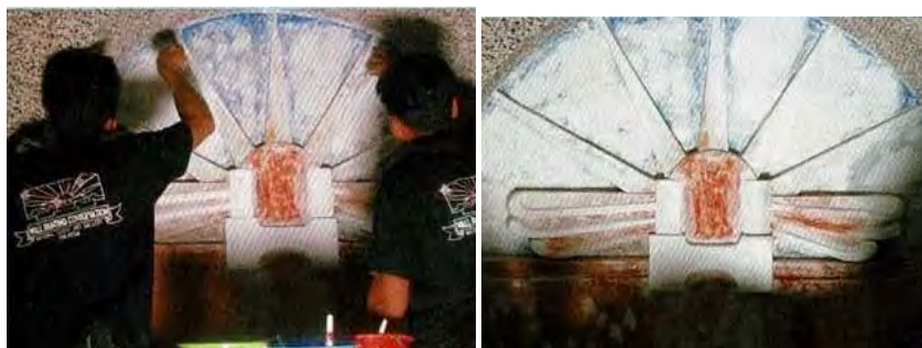
Figure 6: Process of applying the strengthening treatment
