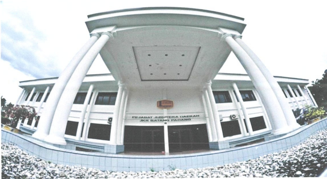
Figure 2.1 the office of JKR Batang Padang
