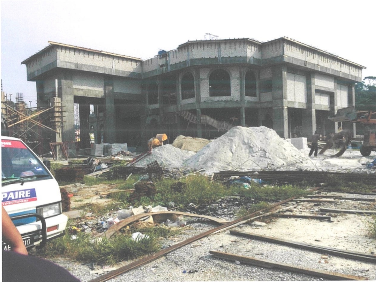
Figure 3.1: Image of Masjid Jamek Tapah in construction
