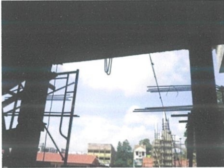
Photo 3.3 The placement of starter bars.
