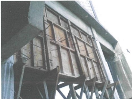
Photo 3.6 Another case of formworks for the concrete pouring.
