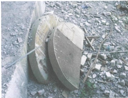
Photo 3.8 Took off the formworks.
