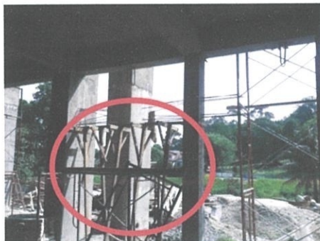
Photo 3.4 The stands being placed.
