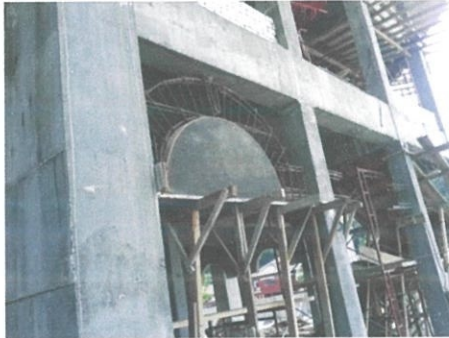
Photo 3.5 The reinforcement bars and formworks is place together.
