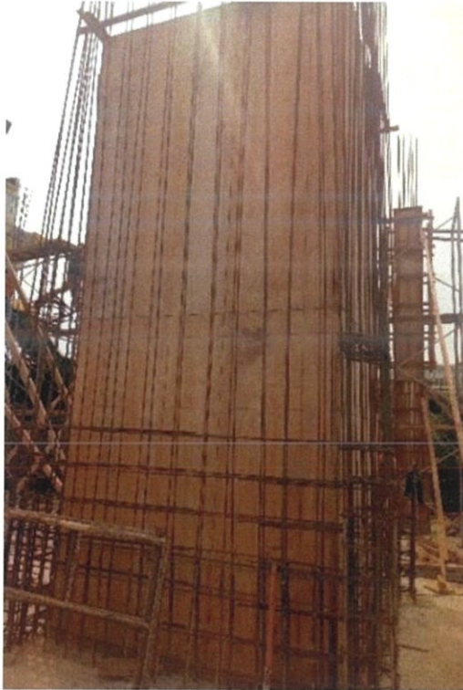
Figure 19: The starter bar for lift shaft
