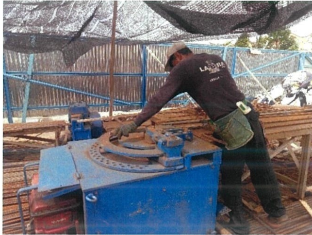
Figure 11: Forming the ground beam reinforcement bars using a bar bending machine
