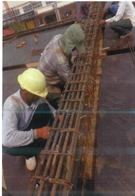
Figure 21: The workers tied the stirrups to the main bar
