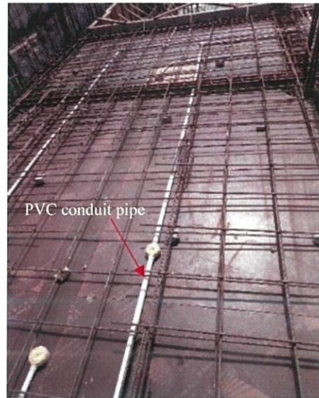
Figure 22: The BRC laid on first floor slab
