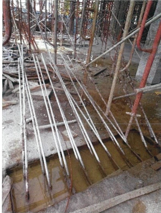
Figure 25: The starter bar for staircase
