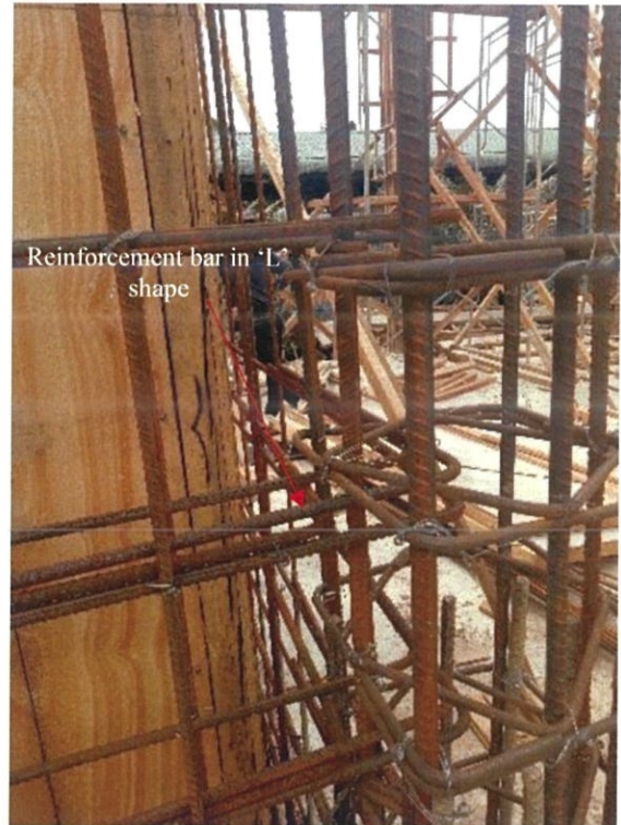
Figure 18: The reinforcement bar in 'L' shape
