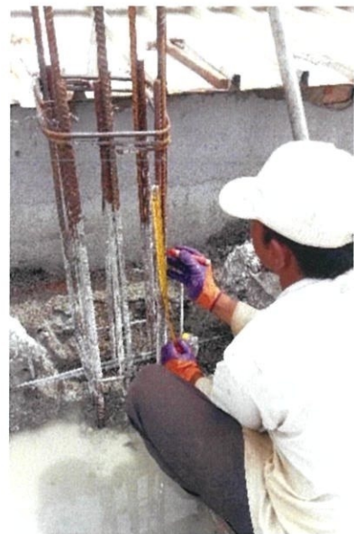
Figure 13: The worker marked the location of stirrup to the main bars
