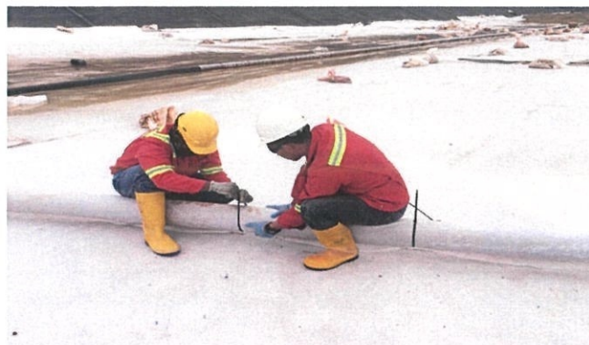
Figure 3.12: Pipe wrapped with geotextile and secured with cable ties
