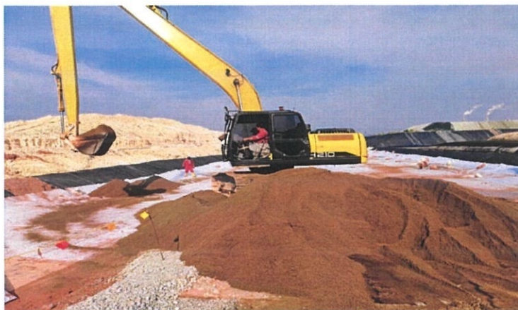
Figure 3.14: Coarse sand as drainage material
