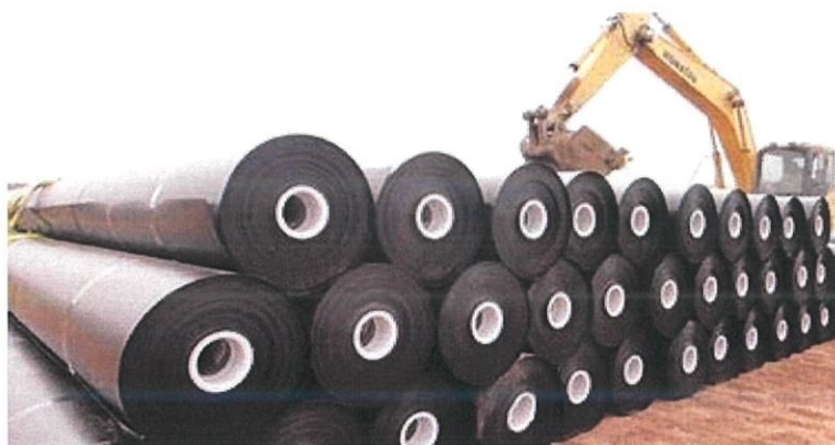
Figure 3.4: Stock pile of 2mm thick HDPE Liner Geomembrane in rolls
