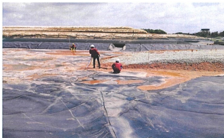
Figure 3.6: Marked cushion geotextile limit
