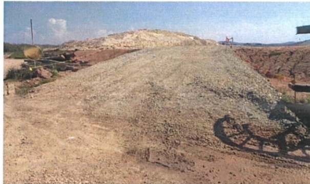
Figure 3.19: Reflector installed along access ramp
