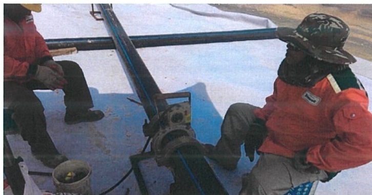
Figure 3.9: Welders weld pipe using butt fusion method
