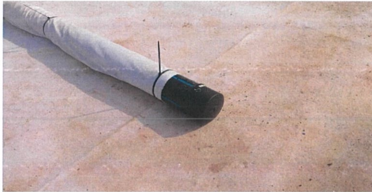
Figure 3.11: Install End Cap at every end of HDPE Pipe
