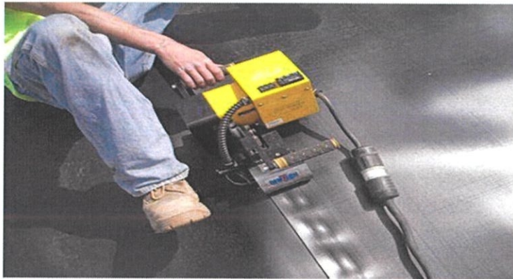
Figure 3.2: Weld HDPE Liner
