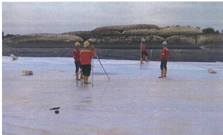
Figure 3.13: Sand level marked by survey team
