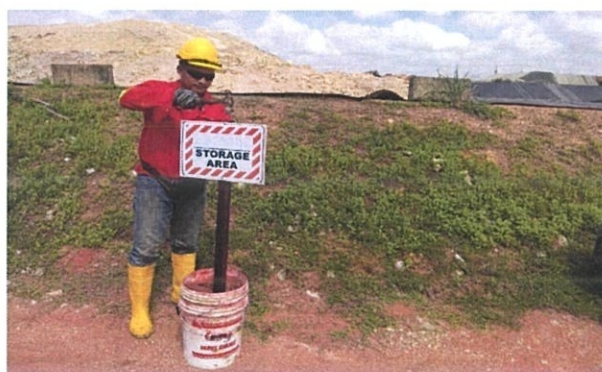
Figure 3.26: General worker set up signage at workplace
