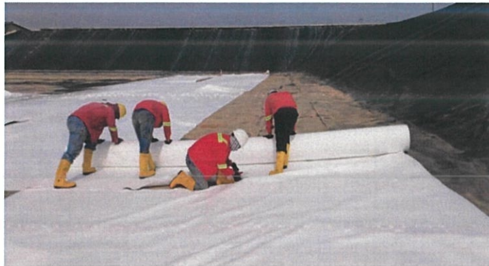
Figure 3.7: General Workers laid Cushion Geotextile on HDPE liner
