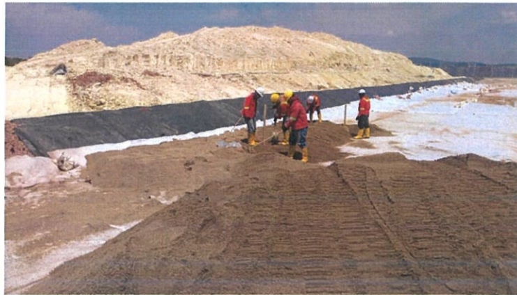
Figure 3.15: Sand manually levelled by general workers
