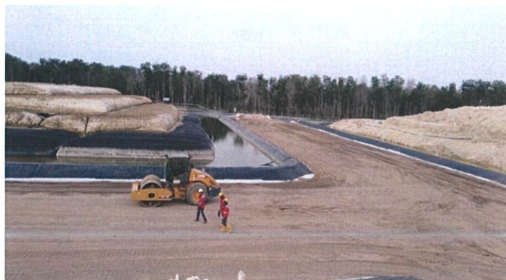
Figure 3.16: Sand compacted by Roller compactor
