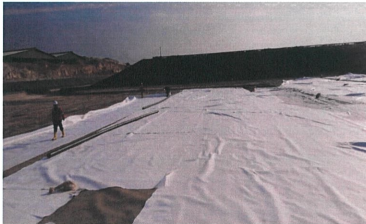
Figure 3.17: Laid separator geotextile
