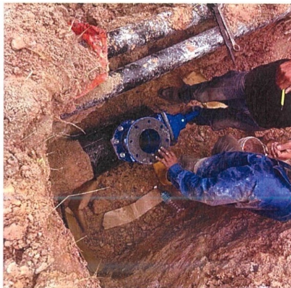
Figure 3.8: Sluice Valve installation
