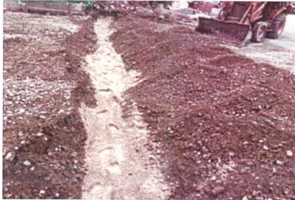
Figure 3.18: HDPE pipe backfilled with crushed run and sand
