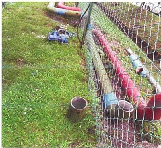
Figure 3.21: MSCL pipe installation process
