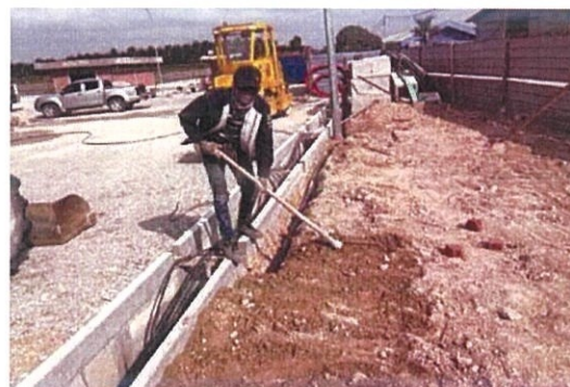
Figure 3.15: HDPE Polyethylene pipe installation
