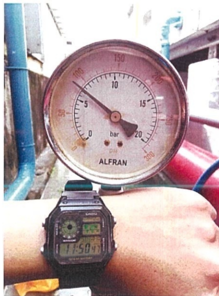
Figure 3.26: MSCL pipe water pressure test
