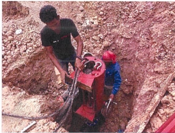
Figure 3.9: Drilling SAJ pipeline using Hot Tapping Machines
