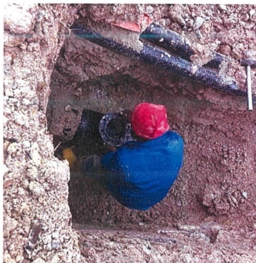
Figure 3.6: Steel Flanged Tee installation
