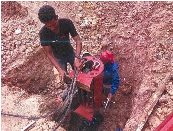
Figure 3.3: Hot tapping operation
