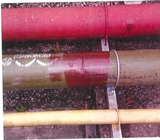
Figure 3.24: Steel bracket installation
