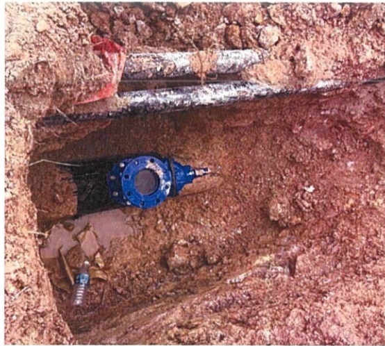
Figure 3.11: Sluice Valve fully installation
