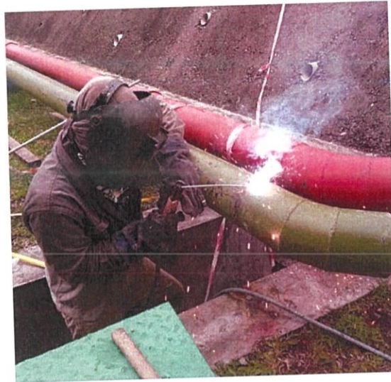
Figure 3.22: Jointing of MSCL pipe fitting
