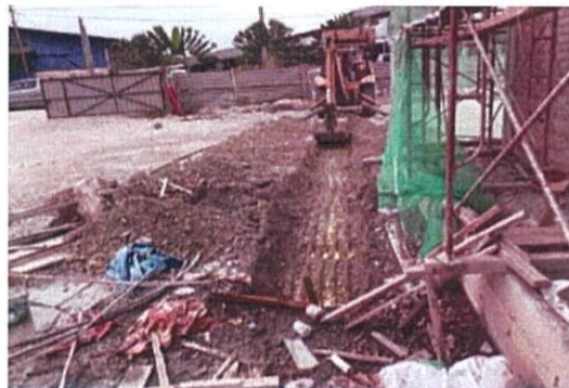
Figure 3.14: HDPE pipeline excavation
