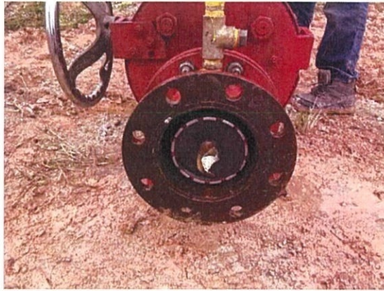
Figure 3.10: SAJ pipeline steel coupon
