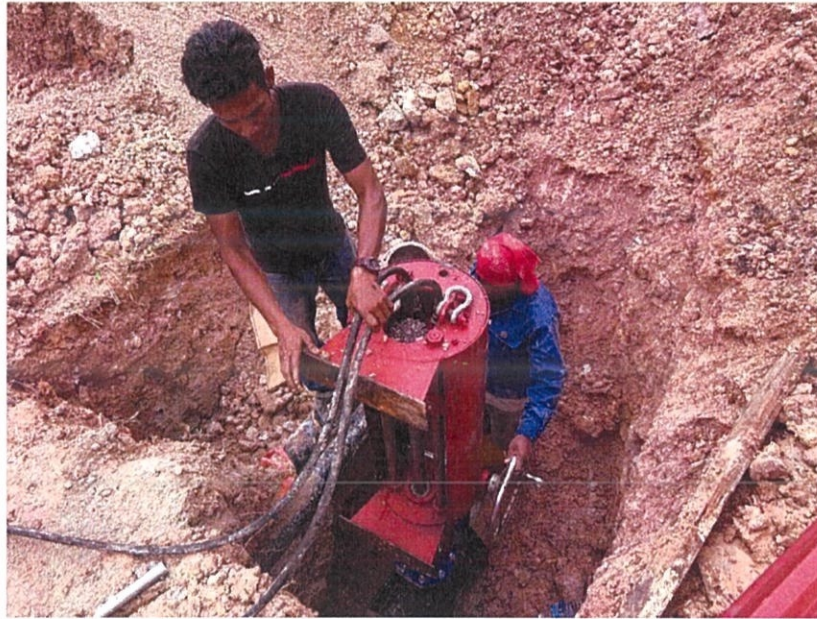
Figure 1.1 : Hot Tapping Equipment
