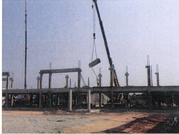
Figure 3.11 Installation Precast Beam
