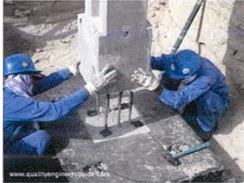
Figure 3.6 Installation precast column
