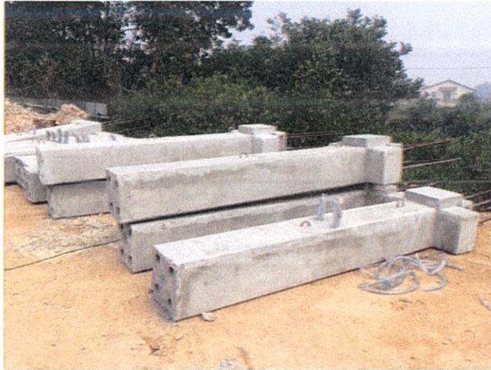
Figure 3.4 Precast Concrete Column
