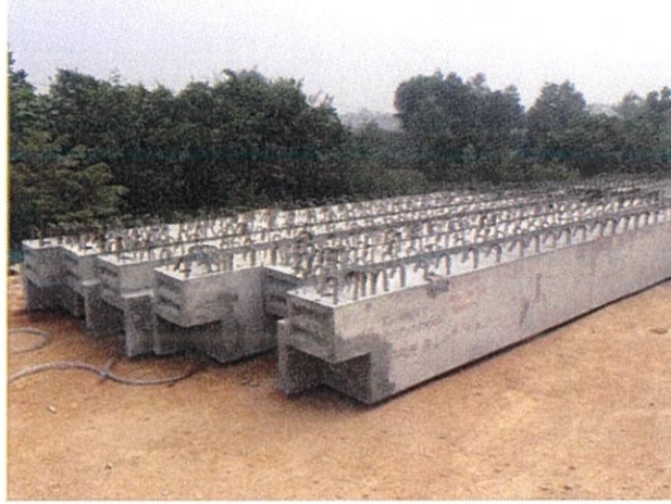
Figure 3.10 Precast Concrete Beam
