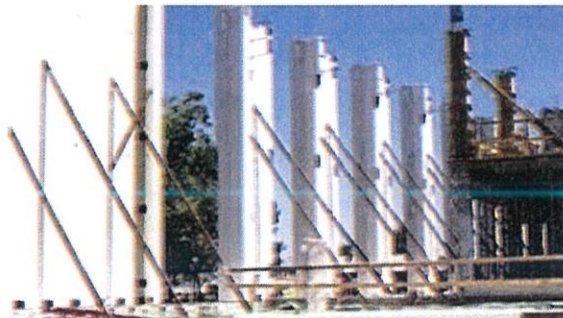
Figure 3.9 Props attach to the column
