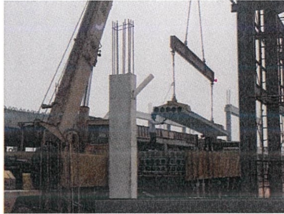
Figure 3.13 Lifting Hollow Core Slab
