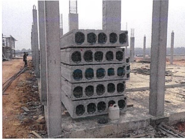
Figure 3.12 Precast Concrete Hollow Core Slab
