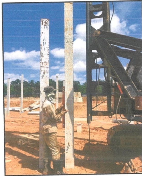
Figure 3.7: Vertically checked using spirit level
