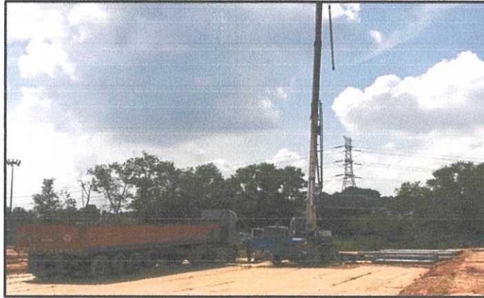
Figure 3.5: Unload RC pile from trailer
