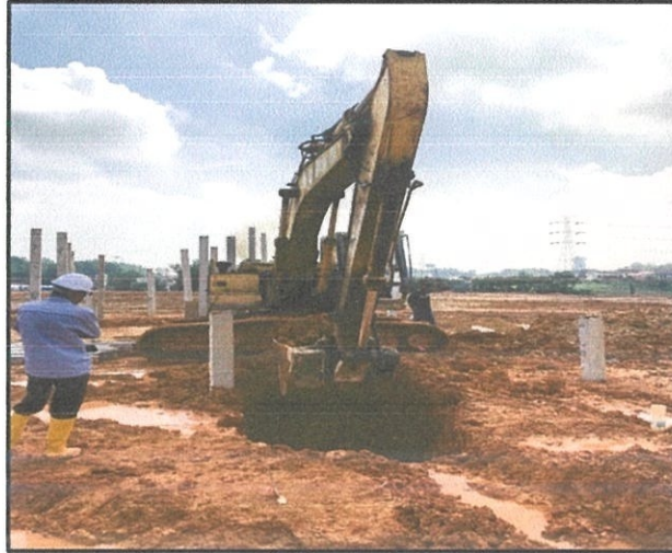
Figure 3.16: Excavator excavate 2m from ground level
