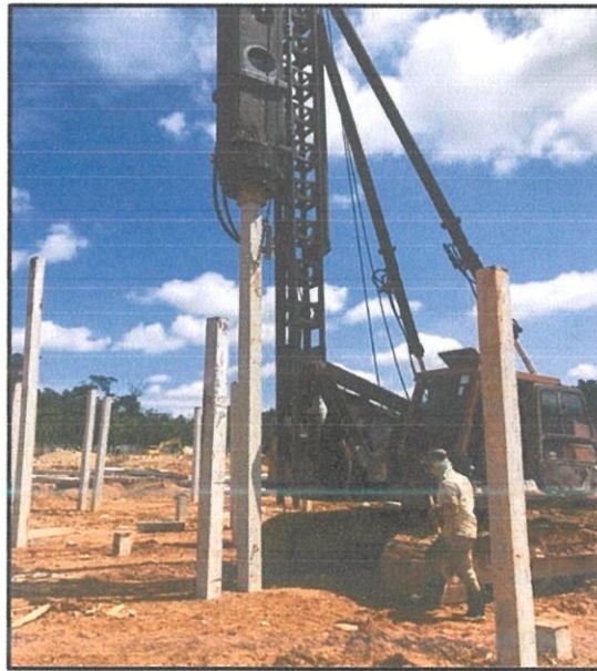
Figure 3.6: Pile is hoist up
