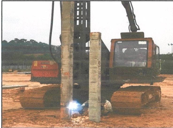
Figure 3.9: Show the worker is welding joint between two piles
