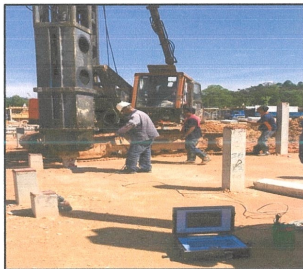
Figure 3.11: PDA test conduct by engineer at point number 61
