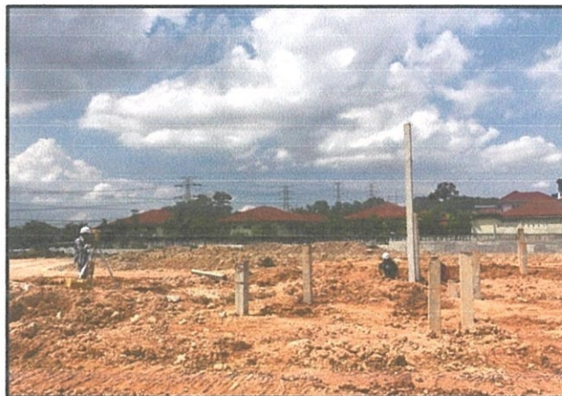
Figure 4: Pegging point by surveyor
