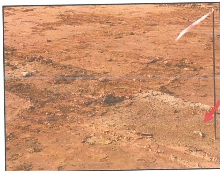
Figure 3.4: Peg that been peg by surveyor
