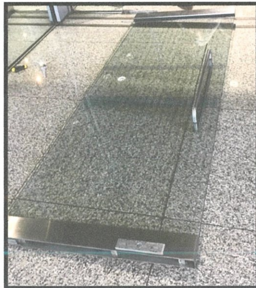
Figure 3.26 The Door Leaf was Remove
