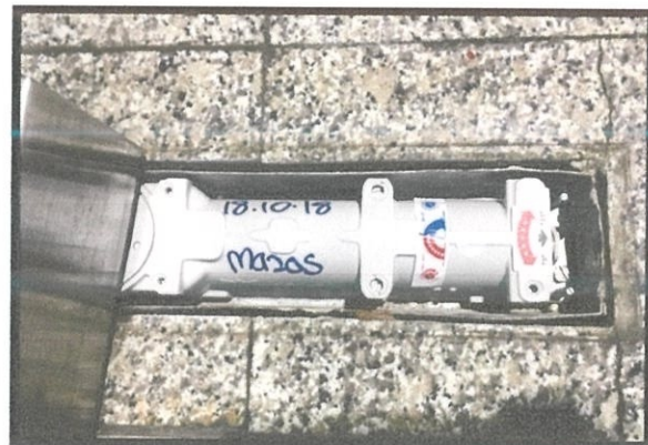
Figure 3.29 The Floor Spring is Replace
