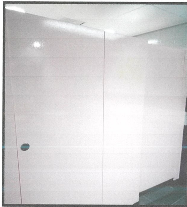
Figure 3.18 After Cubicle Paint
