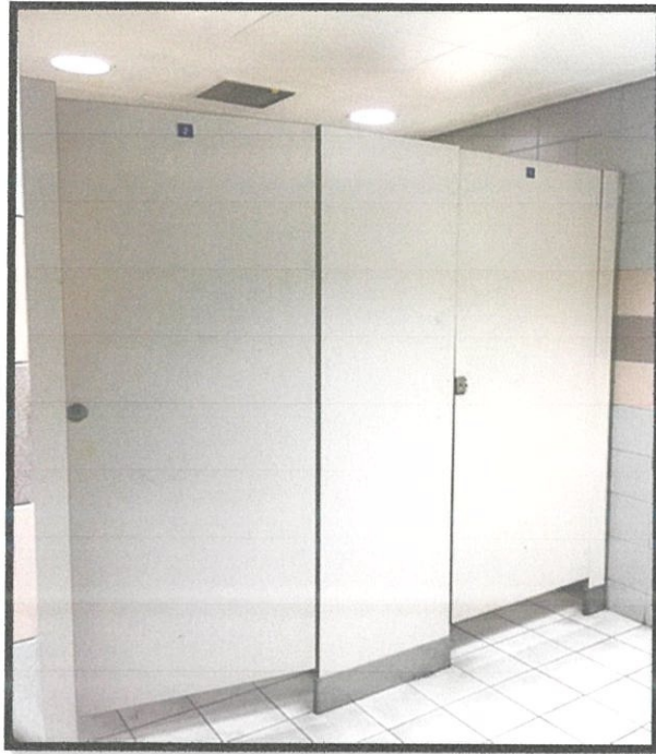
Figure 3.17 Before Cubicle Paint
