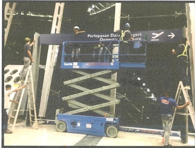
Figure 3.22 The Light Box Installation
