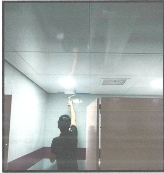
Figure 3.10 Painting the Ceiling
