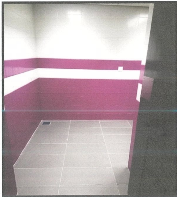
Figure 3.20 After Installing Tiles
