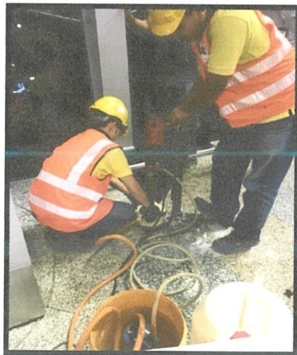
Figure 3.21 Coring Process
