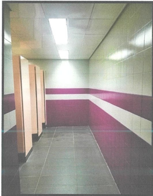
Figure 3.16 Final Layer of Paint
