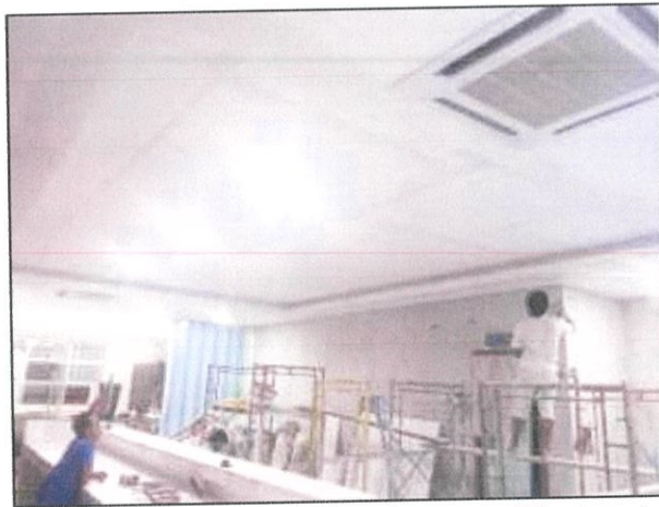
Figure 3.3.12: After completed filling the gap with stopping compound
