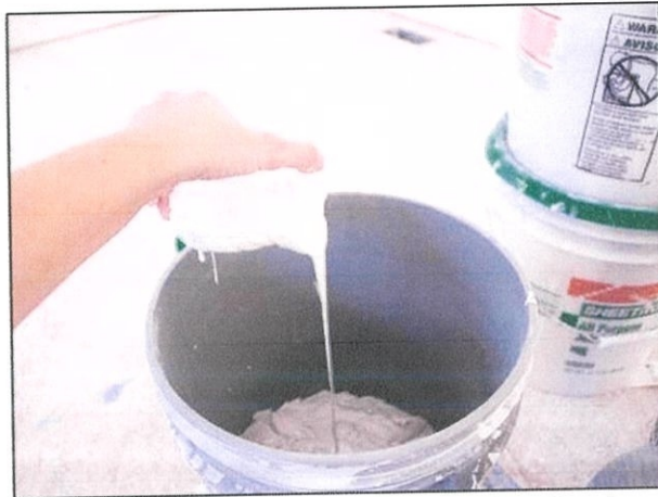
Figure 3.3.11: Mixing compound and water
