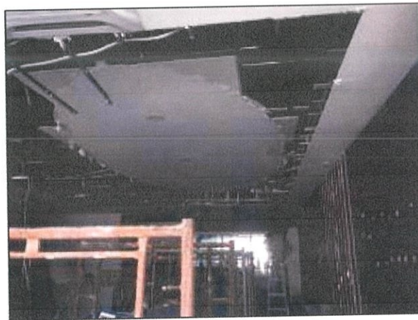
Figure 3.3.2: Dismantle existing plaster board
