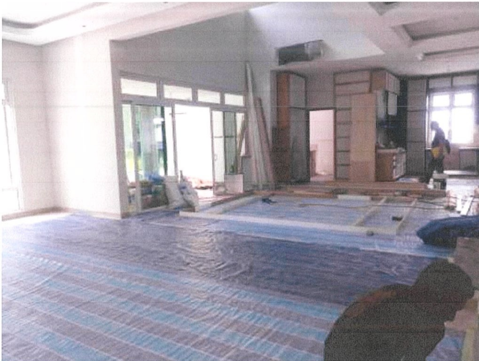
Figure 3.3.1: Floor covering process
