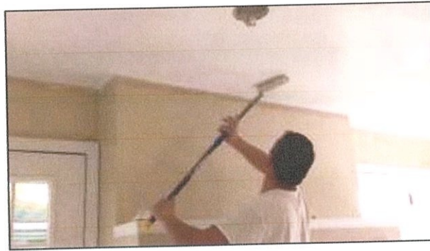
Figure 3.3.14: Applying paint on ceiling
