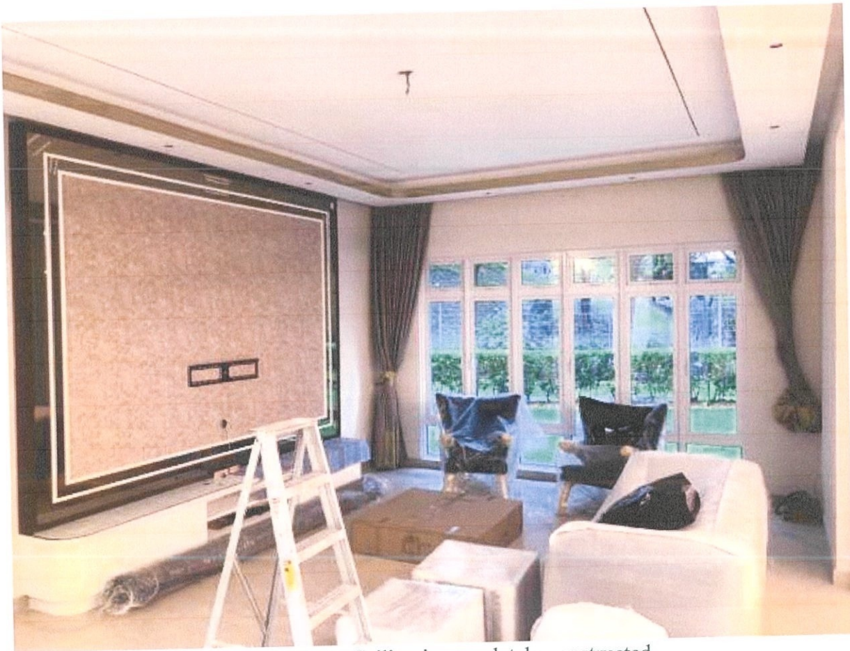
Figure 3.3.15: Ceiling is completely constructed
