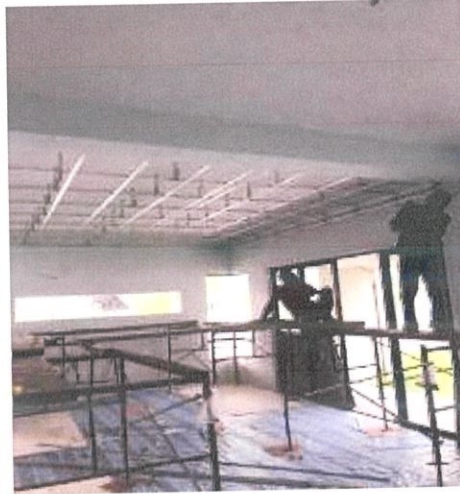
Figure 3.3.5: Ceiling framework
