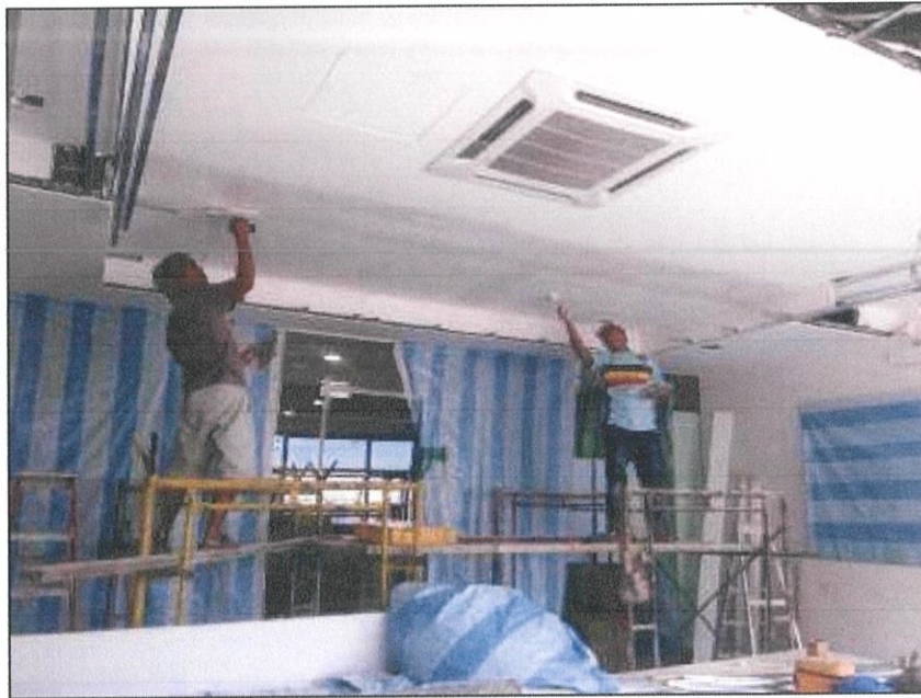
Figure 3.3.8: Installing plasterboard
