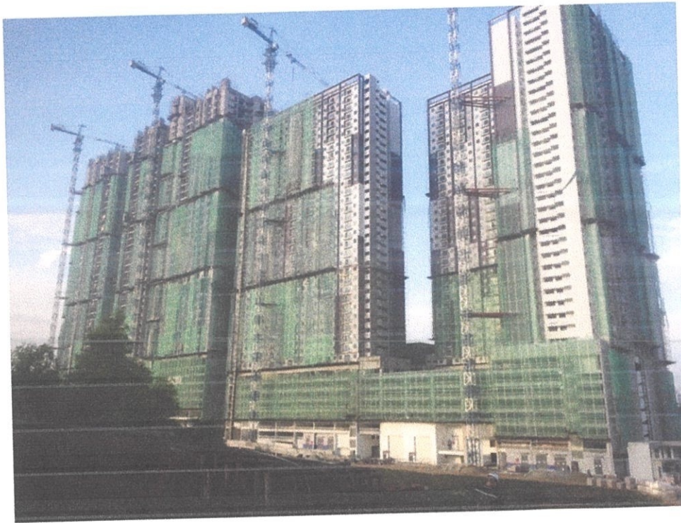
Figure 3.1 : THE HAVRE and JALIL EMAS under construction
