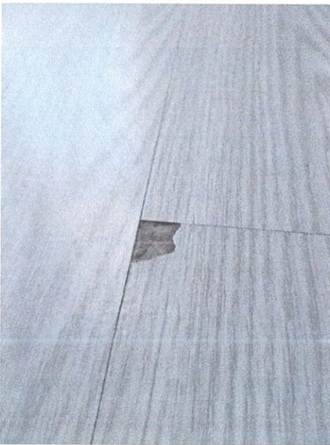
Figure 3.22 : 'Chipping' of laminated floor
