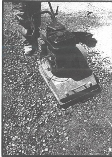
Figure 3.14 The worker is compacting the crusher run
