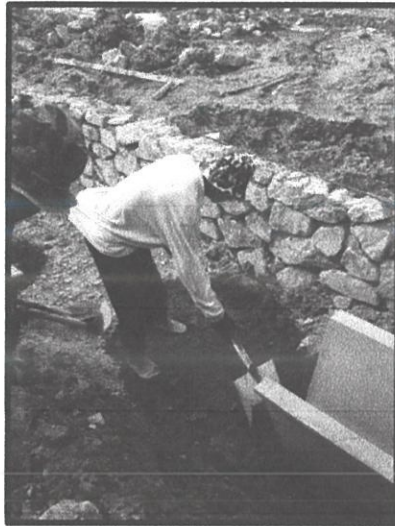
Figure 3.16 The worker is pouring and flattened the mortar
