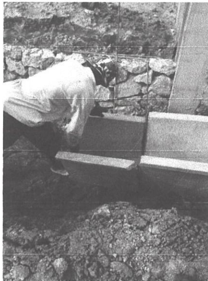
Figure 3.28 Pouring mortar
