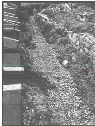
Figure 3.15 Crusher run that has been compacted and flattened
