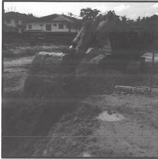
Figure 3.11 Worker using backhoe excavator to excavate the soil
