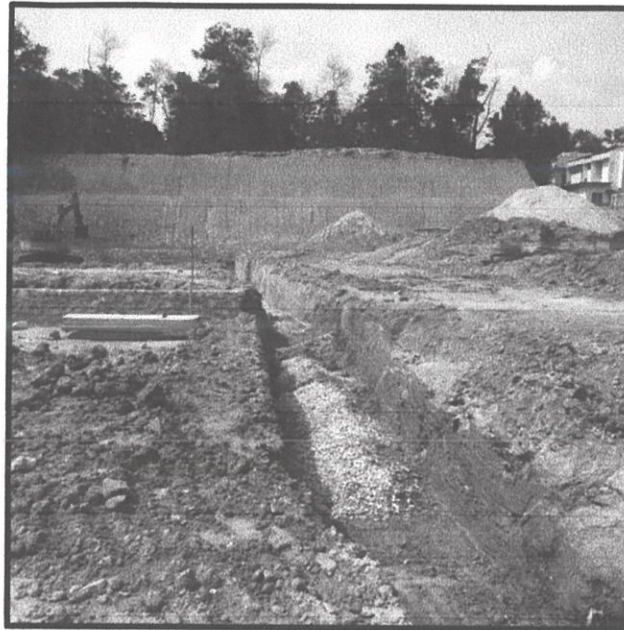
Figure 3.13 Crusher run were put onto the excavated soil
