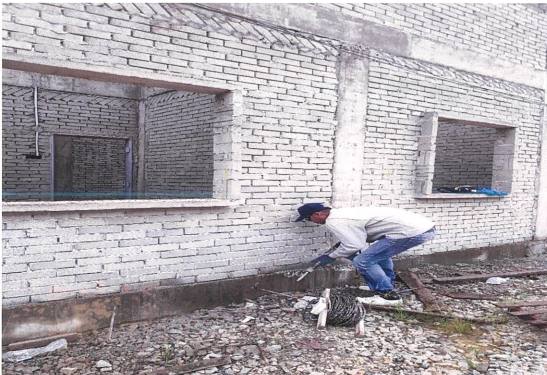
Figure 3.10 The worker hack the edge of beam.
