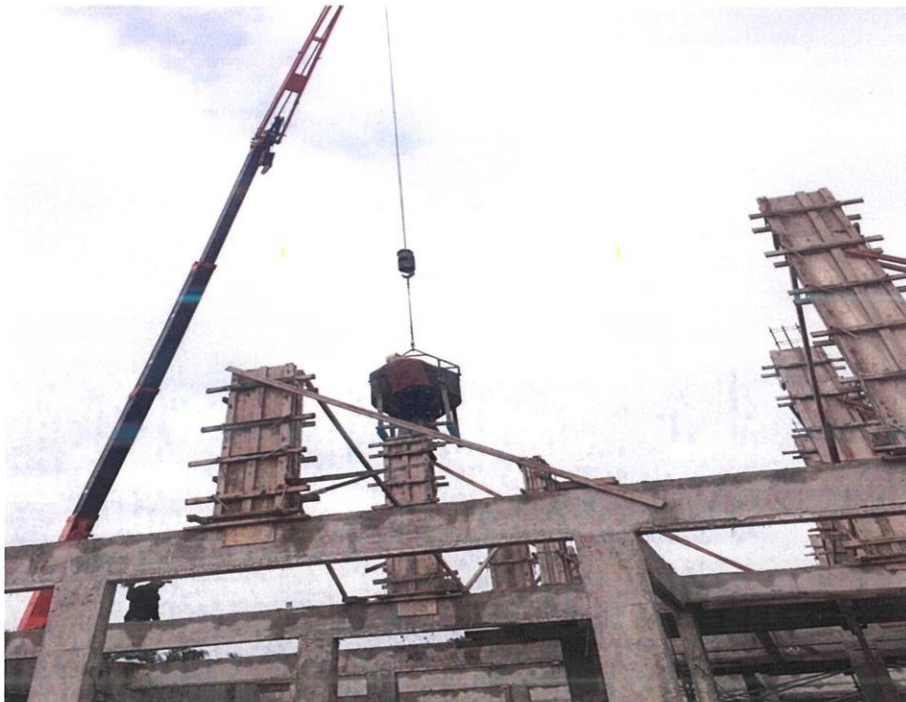
Figure 3.8 The worker is concreting the Beam.
