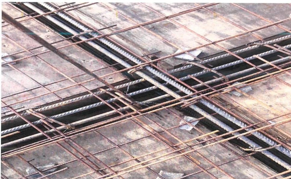
Figure 3.7 The BRC laid on the spacer block
