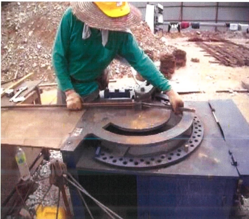
Figure 3.2 Bar bender bending the steel bar
