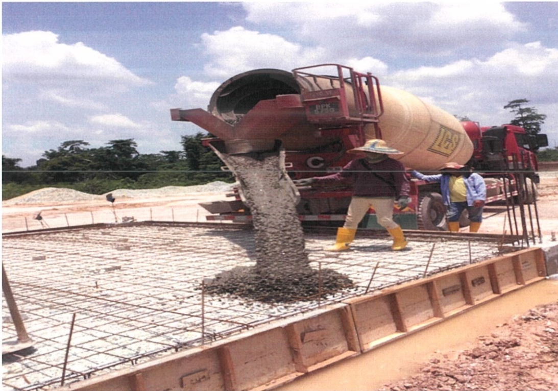
Figure 3.5 Concreting work of slabs
