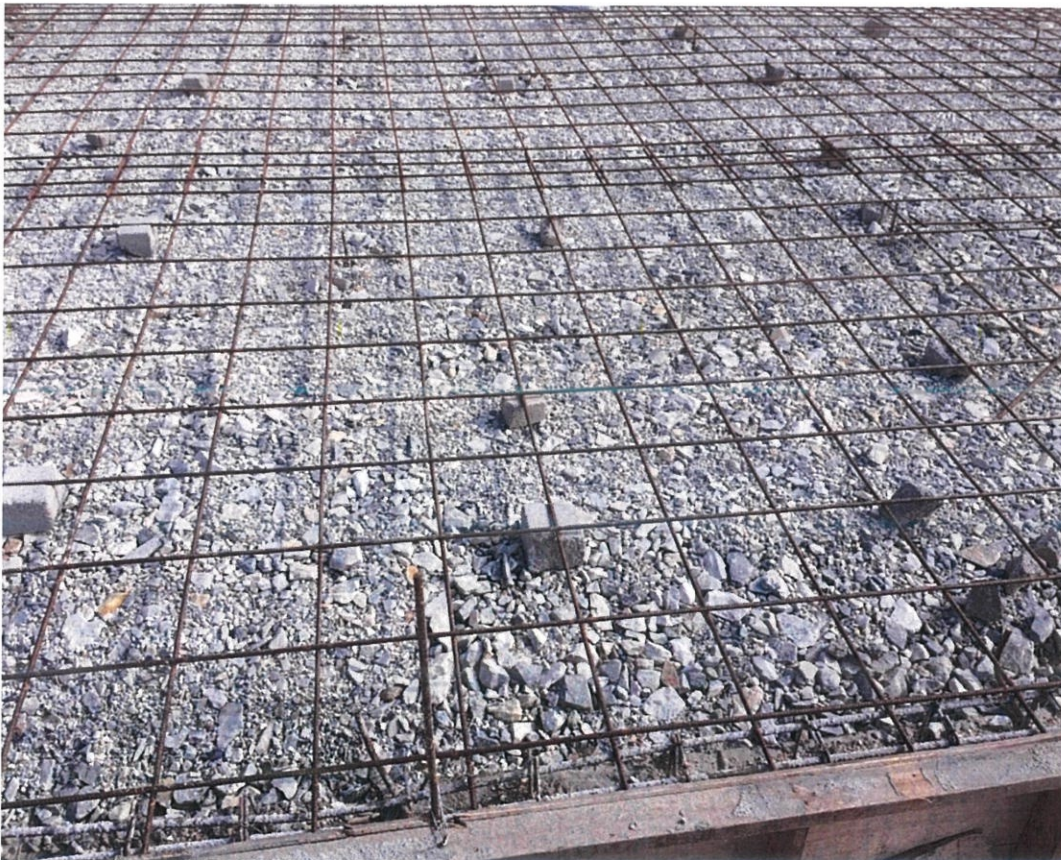
Figure 3.4 The BRC for floor slabs
