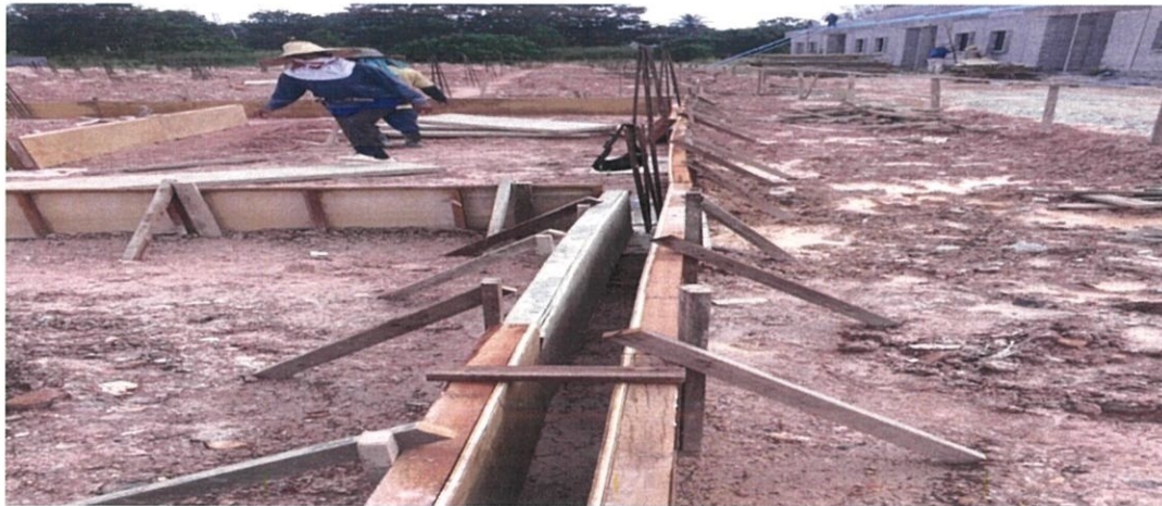
Figure 3.3 Formwork for the ground beams.
