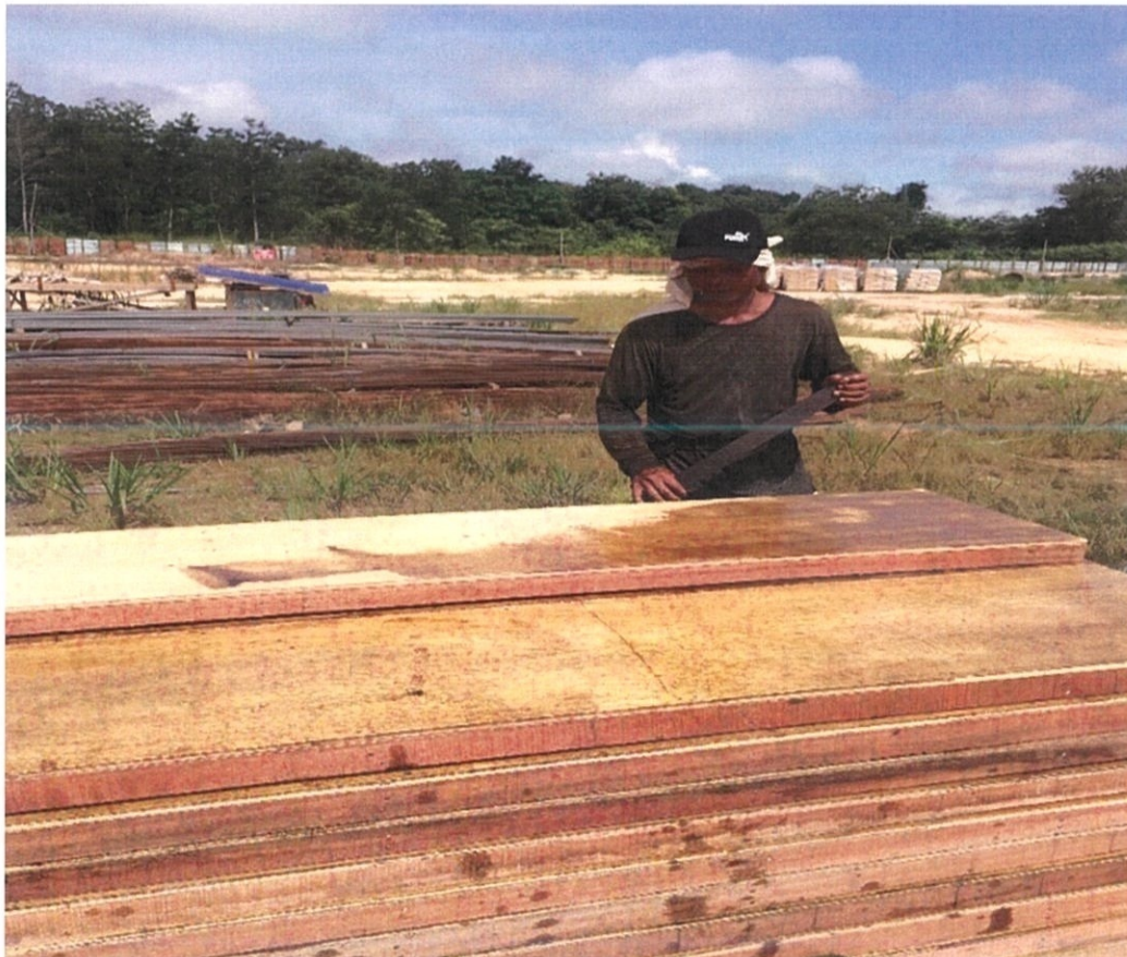
Figure 3.1 The worker is spreading the oil to the formworks.
