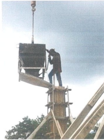
Figure 3.2.11: Pouring of concrete into column
