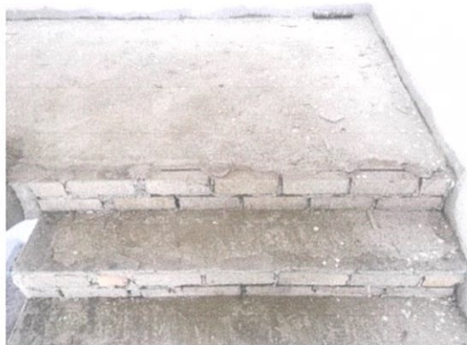
Figure 3.2.17: Install bricks to widen the landing
