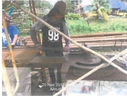
Figure 3.2.9: Cutting and bending reinforcement bar
