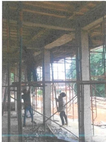
Figure 3.2.6: Remove formwork
