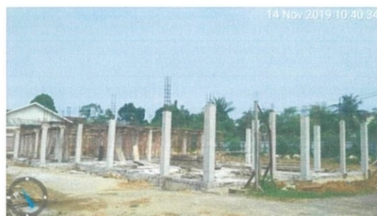
Figure 3.1.2 : Right side of the building
