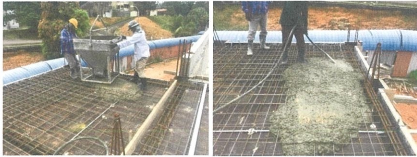
Figure 3.2.4: Pouring of concrete
