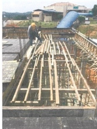
Figure 3.2.2: Installation of formwork for beam and slab
