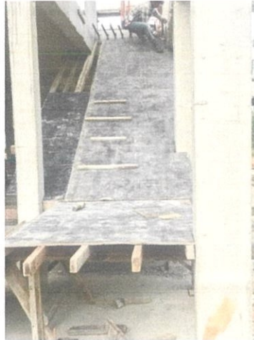
Figure 3.2.15: Installation of staircase formwork
