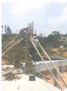
Figure 3.2.10: Installation of formwork
