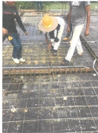
Figure 3.2.3: Installment of reinforcement bar attaches to BRC
