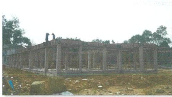
Figure 3.1.3 : Back side of the building
