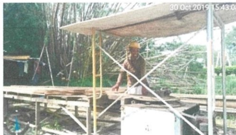
Figure 3.2.14: Bending and cutting reinforcement bar
