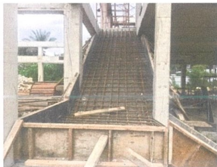
Figure 3.2.16: Reinforcement bar was installed horizontally and vertically
