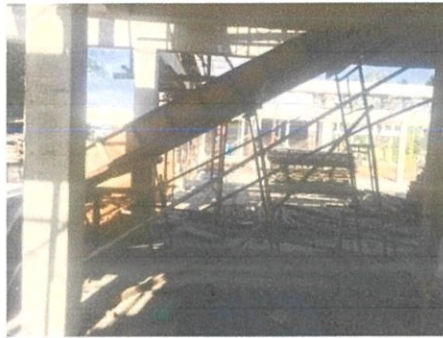
Figure 3.2.13: Installation of scaffold to withstand the stair's load
