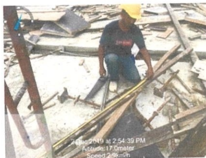
Figure 3.2.8: measure of formwork
