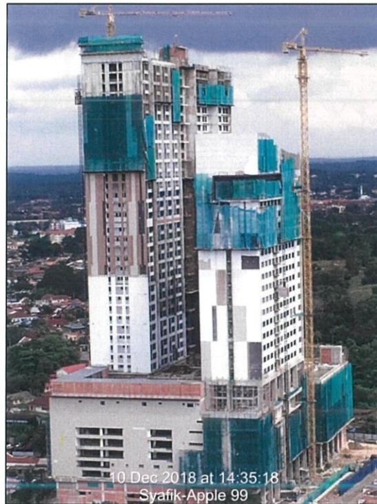
Figure 3.2: Condition of site on December 2018.
