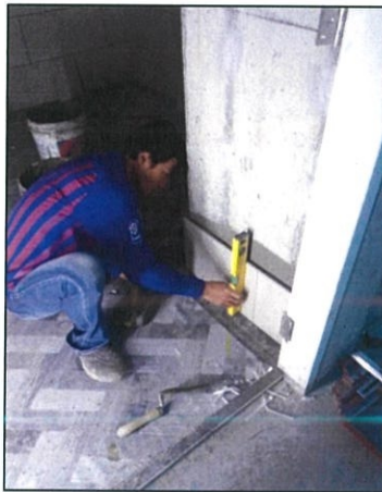
Figure 4.2: The workers make sure the verticality of tiles during installation.
