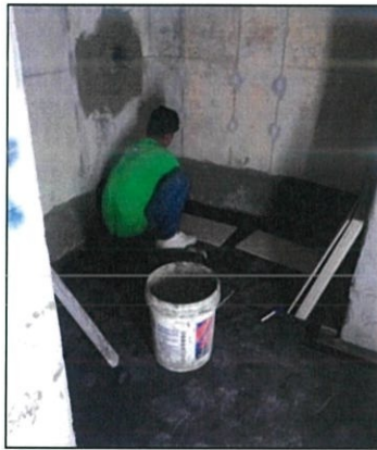
Figure 3.15: The tile layer prepares for install the wall tiles.
