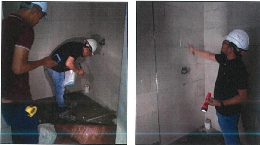
Figure 3.36 : Inspection with client representative.
