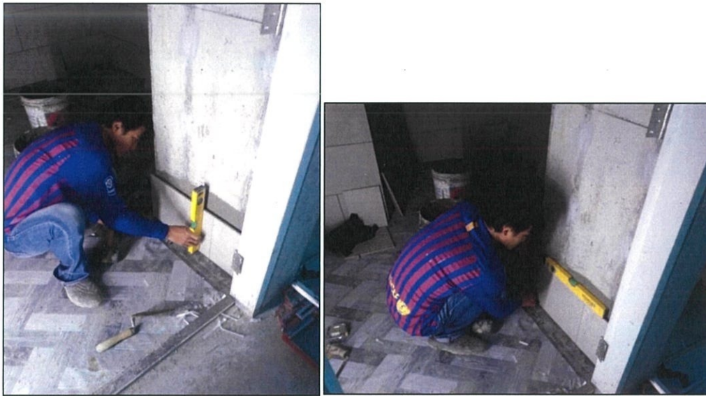
Figure 3.17 : The tile layer use spirit level to check the tiles are horizontal correctly.
