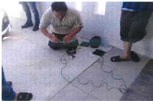
Figure 15 Earthing test for electrical failure
