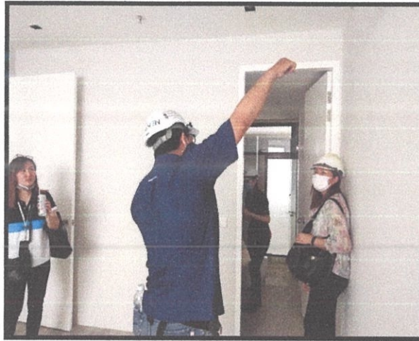
Figure 3.1.3 : Monitoring the work done with the client's representative
