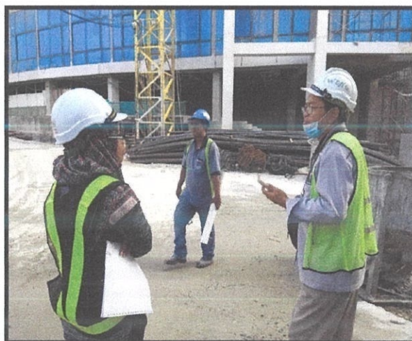
Figure 3.3.2(n) : QA/QC engineer checking the material with the logistic
