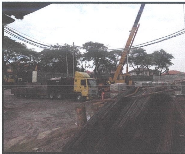
Figure 3.3.2(m) : The cement supplies deliver on site
