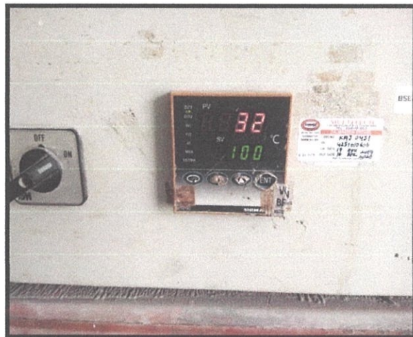
Figure 3.3.2(j) : Heating process after the rebar bend
