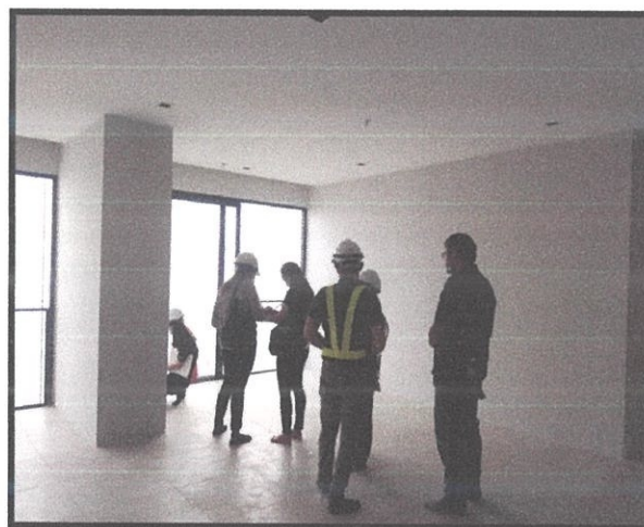
Figure 3.1.4 : Inspection of the outstanding work done in the unit area
