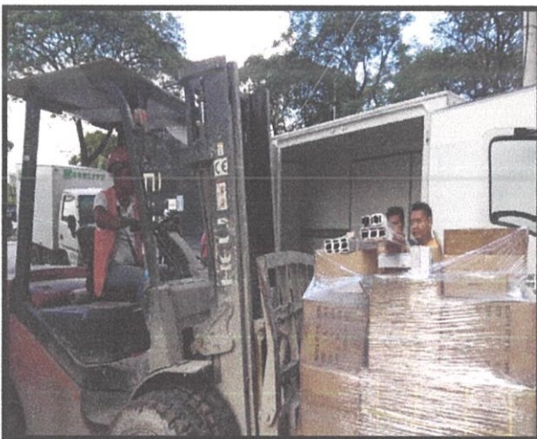
Figure 3.1.2(a) : The ironmongeries supplies, arrive on the construction site
