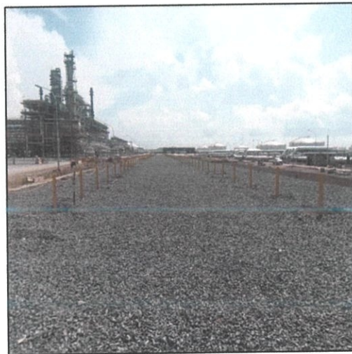
Photo 3.16: Chain Barrier Post has been set up at the site
