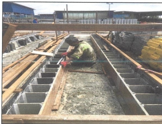
Photo 3.11: Formwork 200mm x 300mm x 12mm constructed
