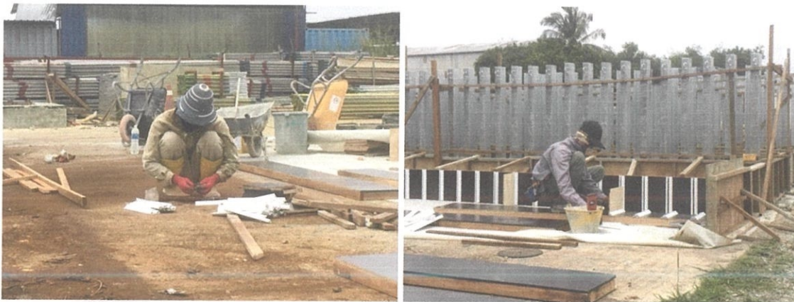
Photo 3.5: Construction of angle steel bar formwork
