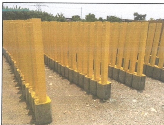
Photo 3.15: Topcoat paint of Angle Steel Pole
