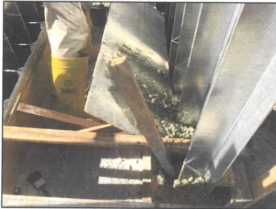
Photo 3.14: The concrete are poured and flattened
