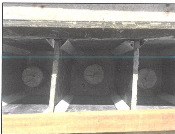
Photo 3.13: Concrete spacer are placed inside the formwork
