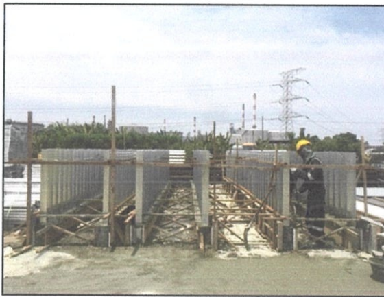
Photo 3.12: Angle Steel Pole are strengthen up before casting
