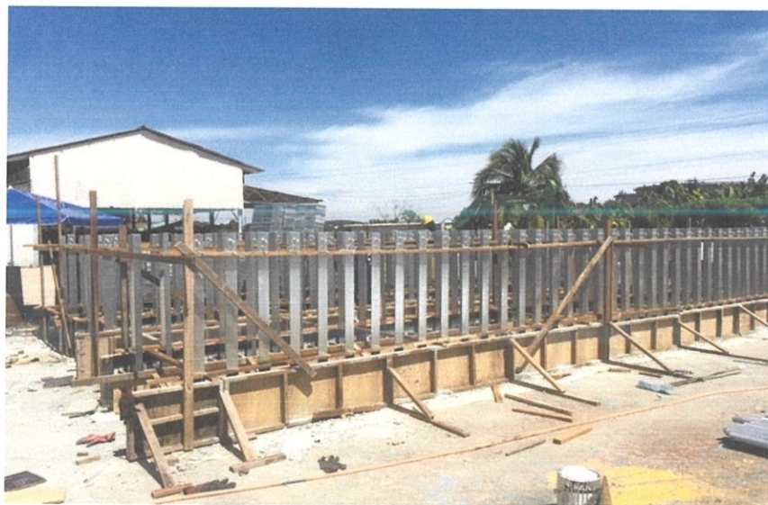
Photo 3.1: Construction of Chain Barrier Post in yard
