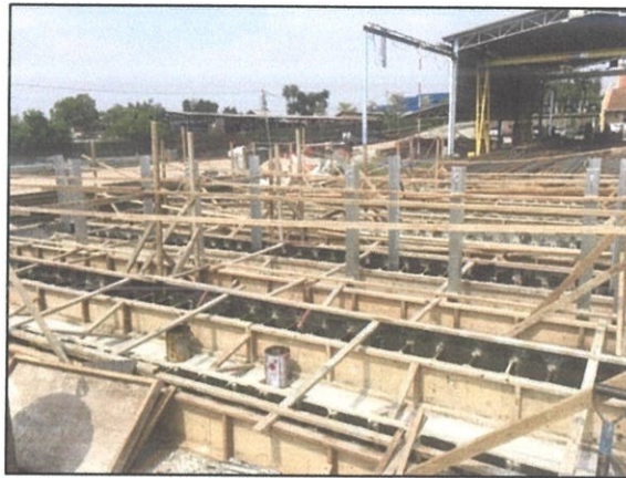
Photo 3.10 : Formwork Installation
