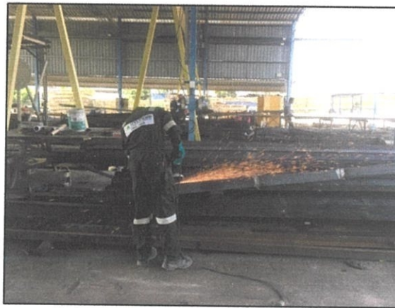
Photo 3.8: Grinding the end tail of each side of the angle bar
