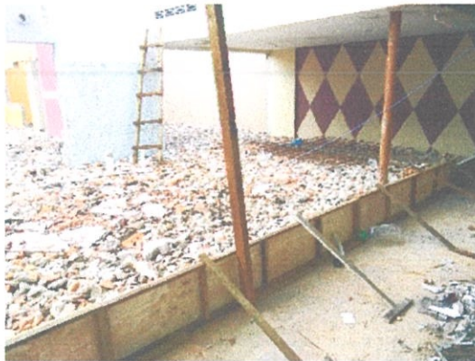
Figure 3.2.12 : Formwork for new floor
