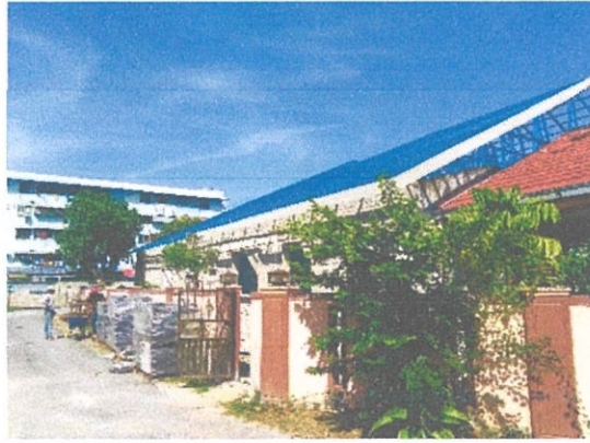
Figure 3.2.23 : The look after installing fascia board
