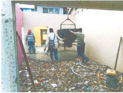
Figure 3.2.15 : Concrete pouring from bucket
