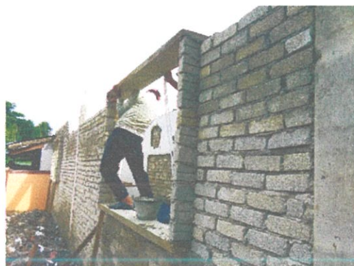
Figure 3.2.18 : Lintel for window
