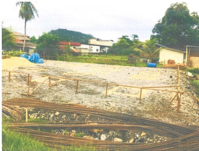
Figure 3.3.1.1 : Example of setting out for new house
