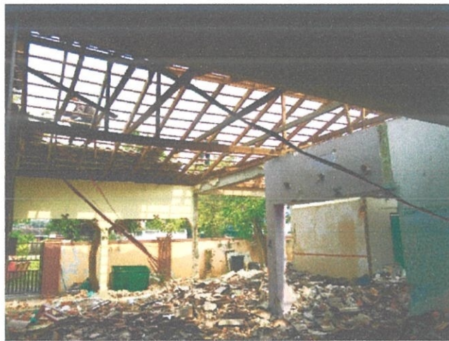
Figure 3.2.4 : Process of tear off the roof
