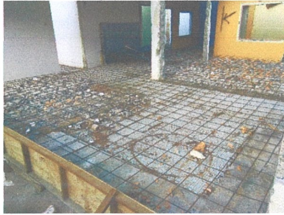
Figure 3.2.13 : BRC laying
