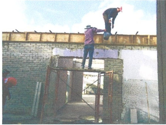
Figure 3.2.19 : Concrete pouring to the upper beam
