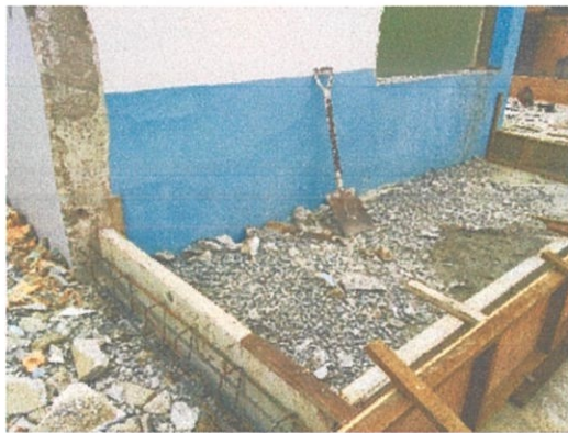
Figure 3.2.10 : Making of a new ground beam
