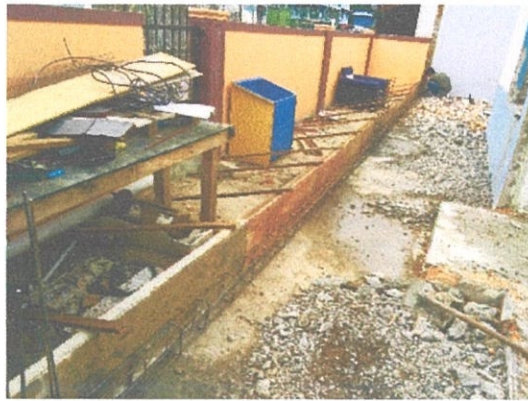
Figure 3.2.9 : Making of a new beam
