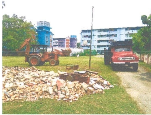
Figure 3.2.6 : Using excavator and lorry to remove the rubbish
