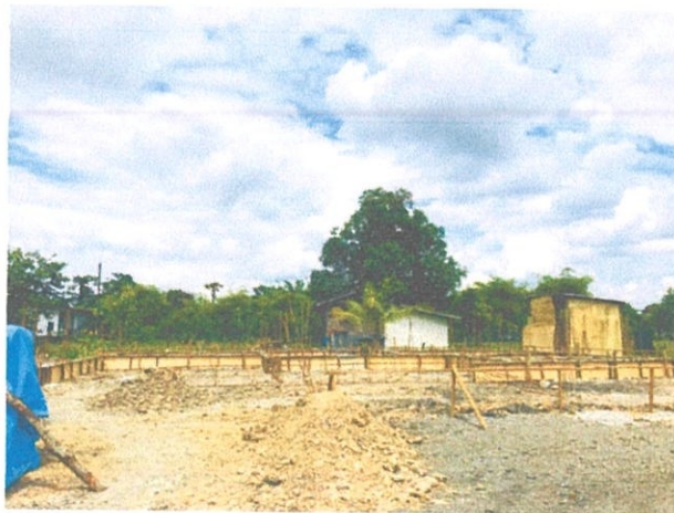
Figure 3.3.2.2 : Example of ground beam for new house.
