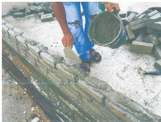
Figure 3.2.16 : Brick layering work
