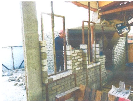
Figure 3.2.17 : Timber frame to make space for the actual window
