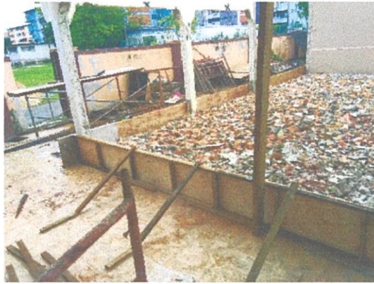
Figure 3.2.11 : Formwork for new floor
