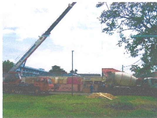
Figure 3.2.14 : Crane and concrete mixer
