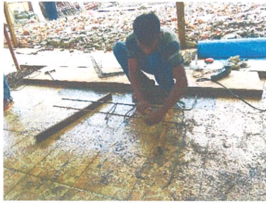
Figure 3.2.7 : Rebar for footing
