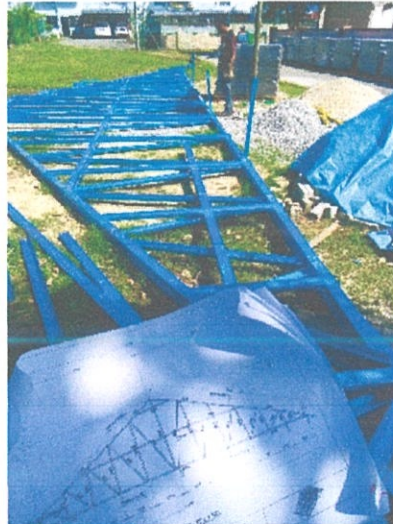
Figure 3.2.20 : Checking on the roof truss
