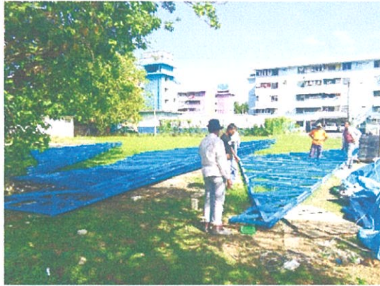
Figure 3.2.21 : Workers lifting the truss
