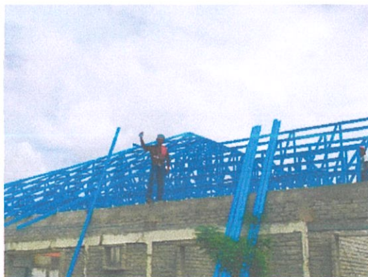
Figure 3.2.22 : Secure the position of the truss
