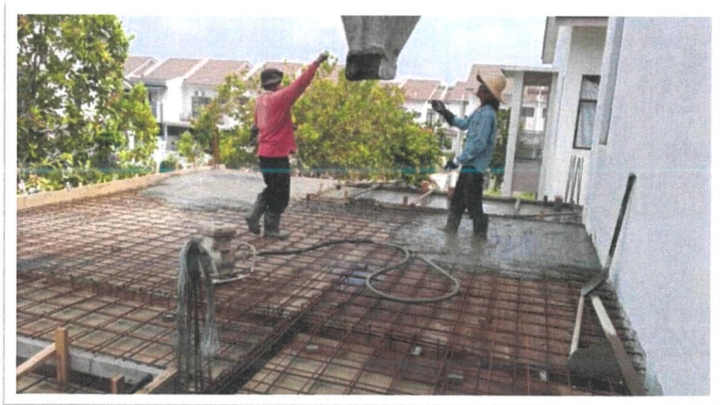
Figure 3.25 : Workers are handling the concrete bucket.
