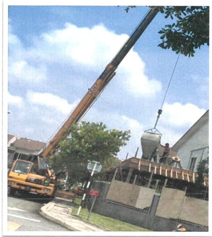
Figure 114 : Concrete poured on the slab.
