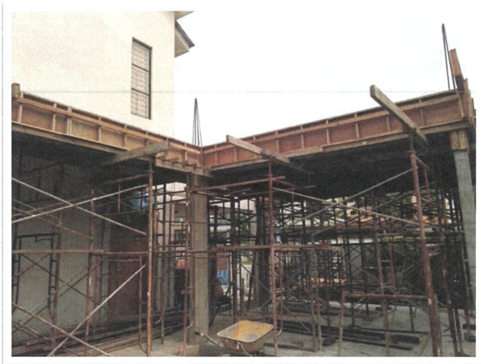
Figure 3.19 : First floor beam formwork
