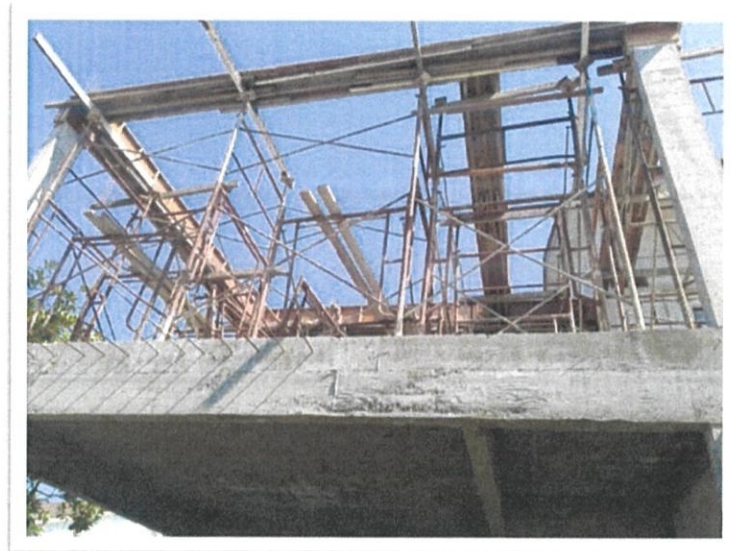
Figure 13 : Roof beam formwork on progress
