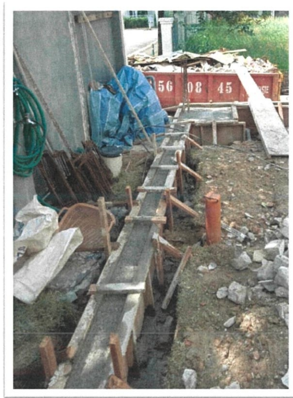
Figure 3.13 : Ground beam formwork filled with concrete
