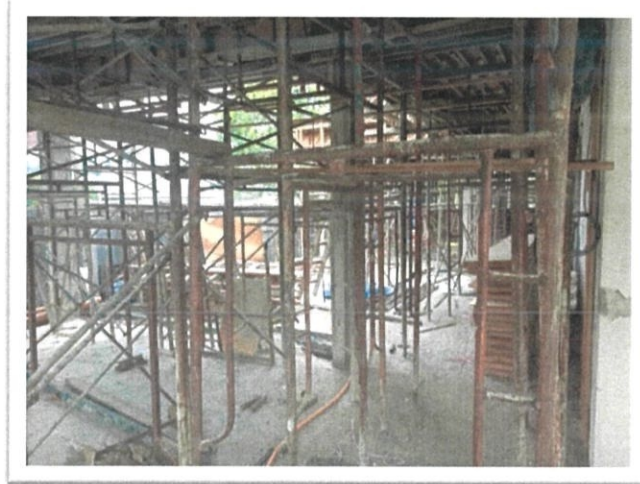
Figure 3.22 : Temporary supporters for first floor slab.
