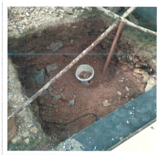
Figure 3.8 : Excavated soil for foundation
