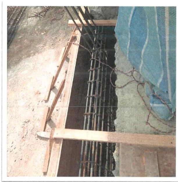
Figure 8 : Reinforcement bars placed in formwork
