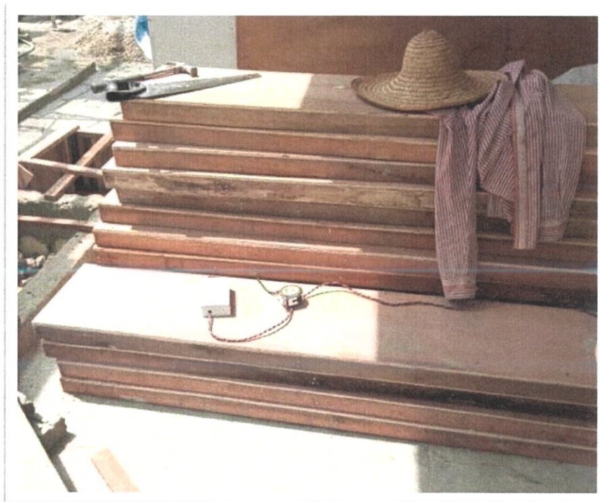
Figure 3.33 : Plywood formwork
