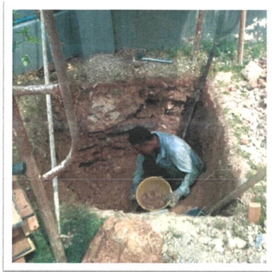
Figure 3.7 : Worker excavating the foundation
