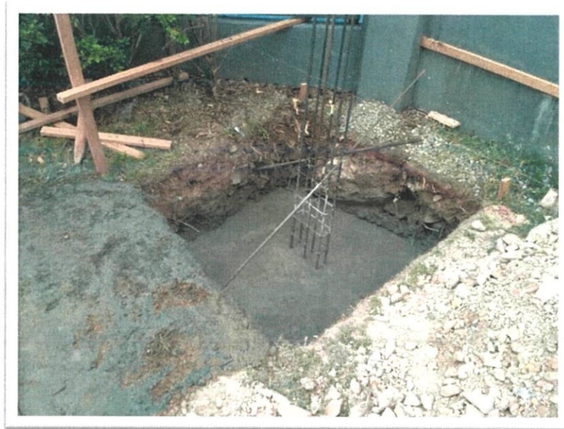
Figure 3.9 : Foundation filled with concrete
