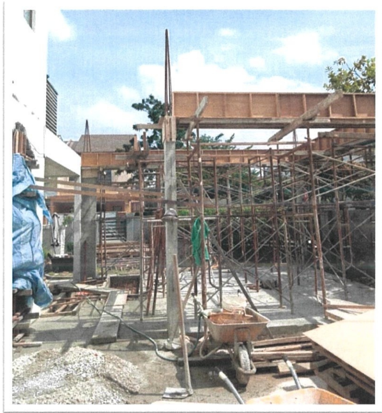
Figure 3.20 : First floor beam formwork
