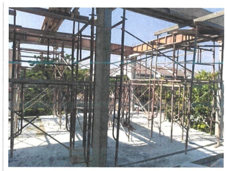
Figure 14 : Roof beam formwork on progress
