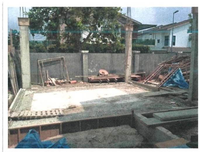
Figure 3.18 : Completed slab and column formwork dismantled
