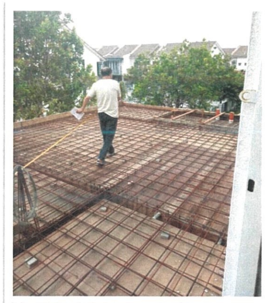
Figure 3.23 : First floor slab on progress.
