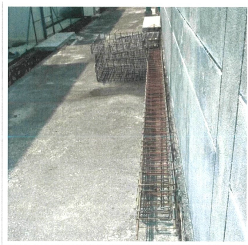
Figure 3.35 : Steel structure for beam
