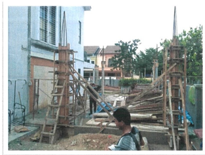
Figure 3.17 : Column formwork
