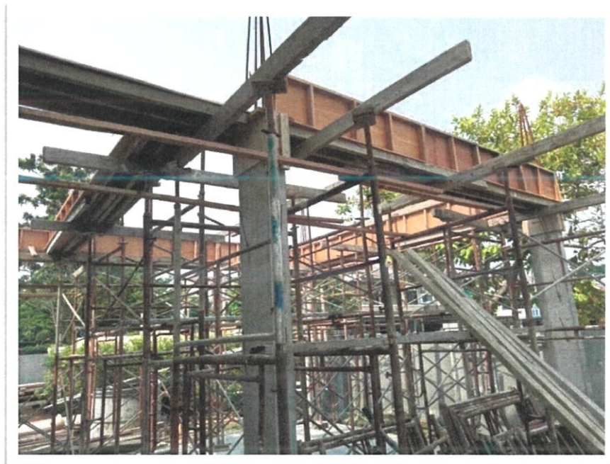
Figure 10 : First floor beam formwork
