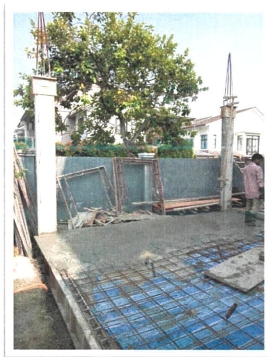
Figure 3.16 : Ground floor slab on progress
