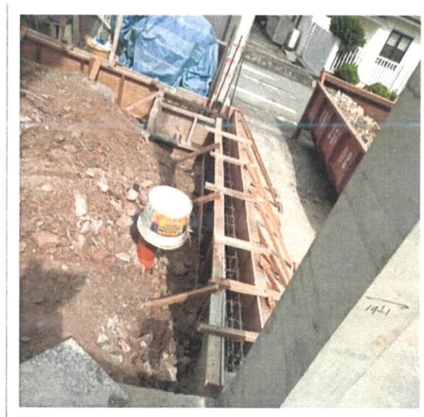
Figure 3.12 : Ground beam formwork
