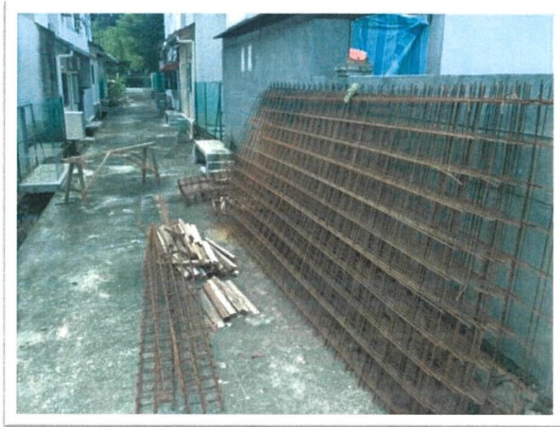
Figure 3.34 : Steel structure for slab
