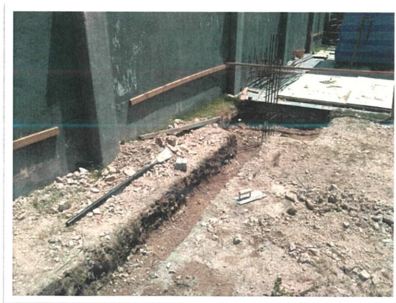
Figure 3.10 : Excavated ground beam.
