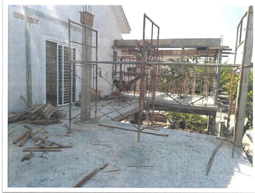
Figure 12 : First floor column formwork dismantled.
