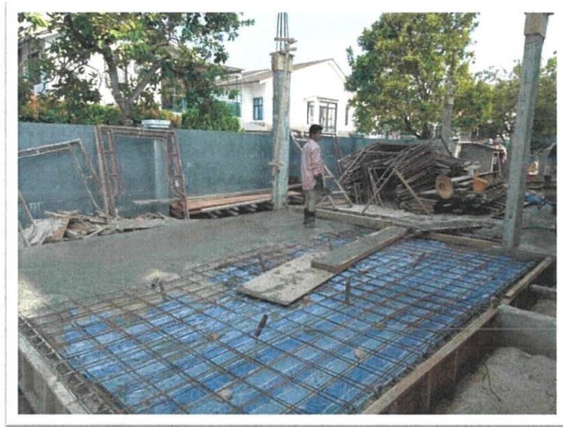
Figure 3.15 : Ground floor slab on progress
