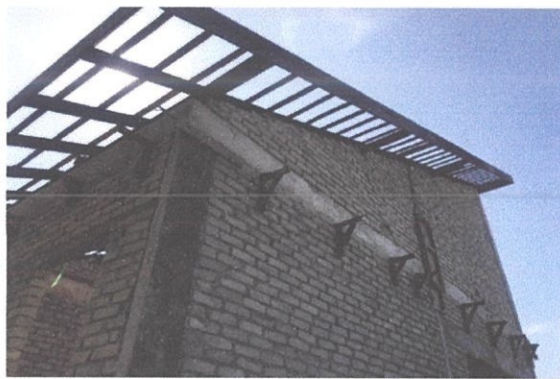
Photo 3.3: Determine the roof angle and shape
