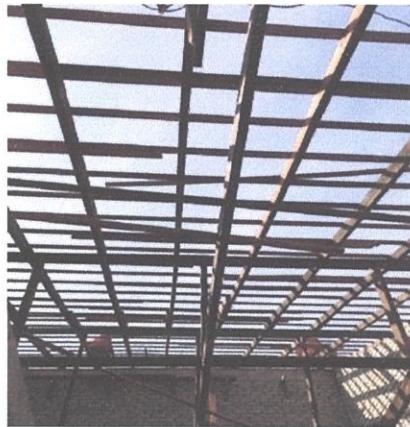
Photo 3.2: Install the rafter
