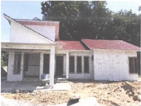
Photo 3.4: Installation of roof tiles
