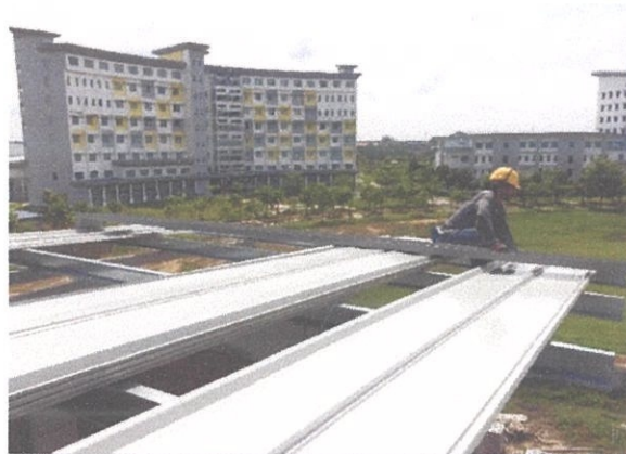
Figure 3.66: Flashing installation
