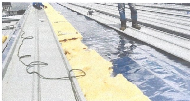
Figure 3.63: Lay the aluminium foil and glass fibre
