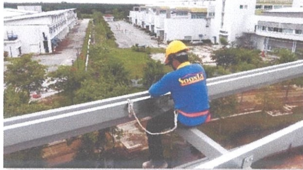
Figure 3.61: Installation of fascia
