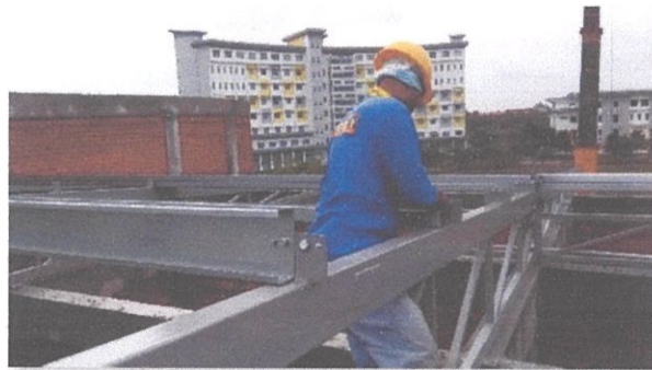
Figure 3.62: Purlin installation
