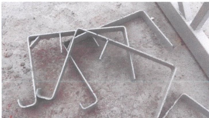
Figure 3.13: Bracket gutter
