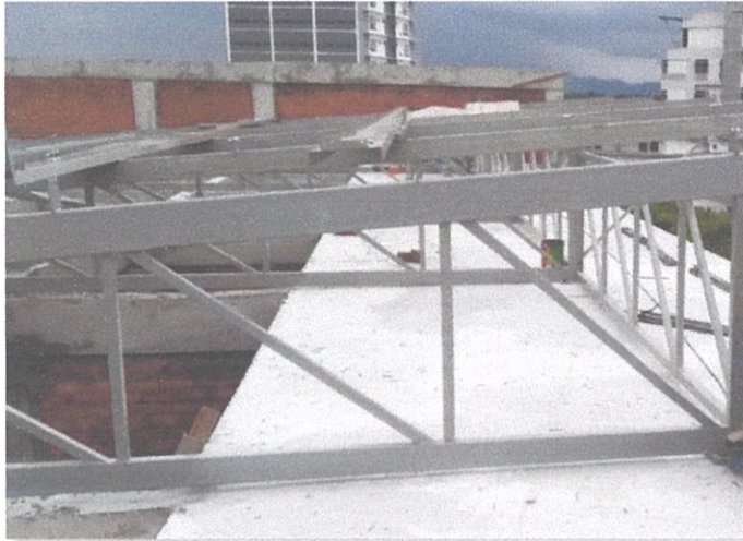
Figure 3.8: Web members in a steel trusses
