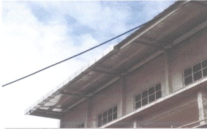
Figure 3.14: Gutter on roof
