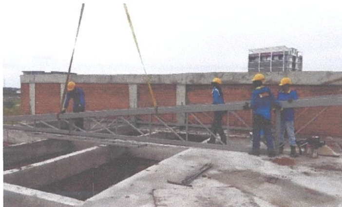
Figure 3.51: Placing T1 trusses
