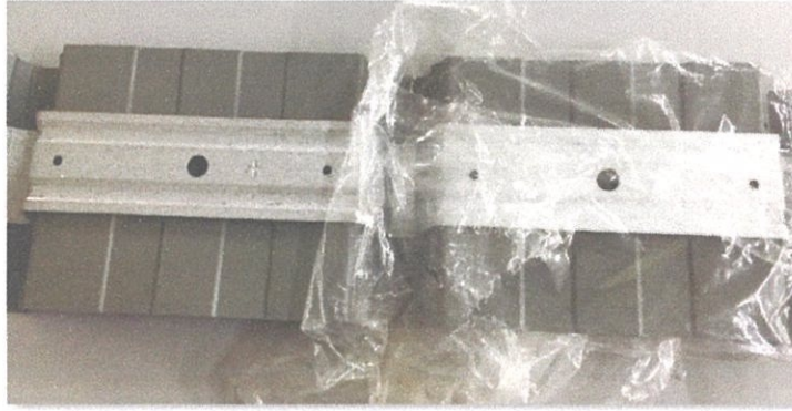
Figure 3.12: Back of metal deck
