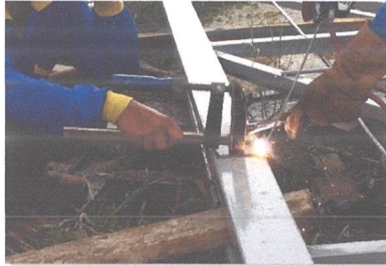
Figure 3.28: Welding on site
