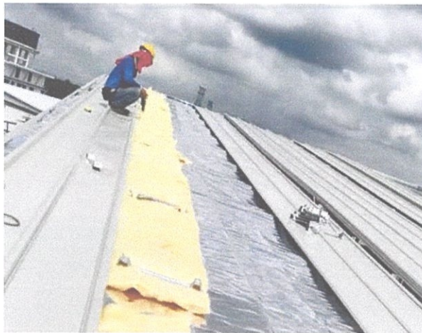
Figure 3.65: Metal deck installation
