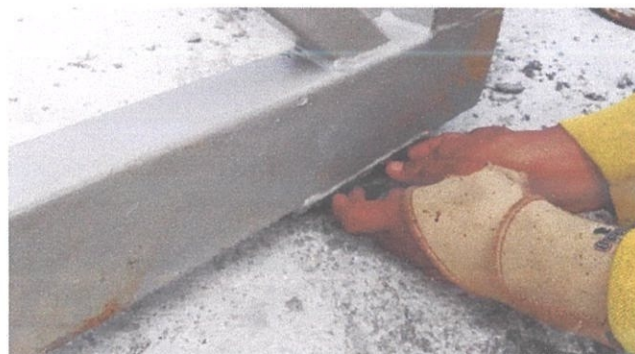
Figure 3.60: Insert washer
