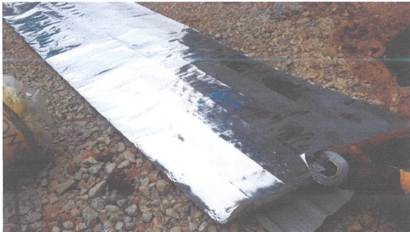
Figure 3.9: Aluminium foil being lay on the ground
