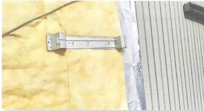
Figure 3.64: Clipping the wool with aluminium foil
