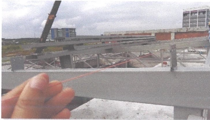
Figure 3.55: Guide thread
