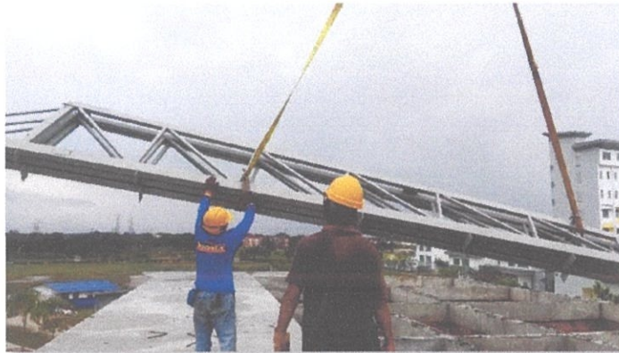
Figure 3.50: Lifting trusses
