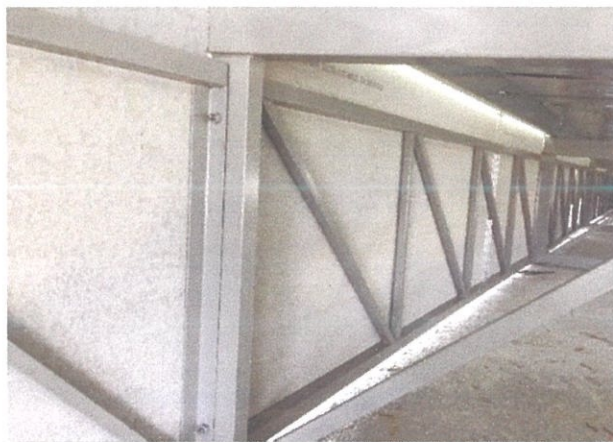
Figure 3.17: Cement board attached to trusses
