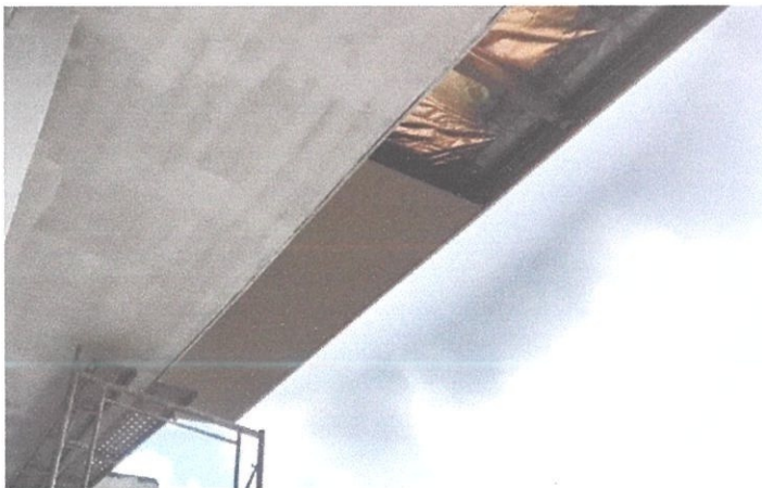
Figure 3.19: Strip ceiling attached to trusses
