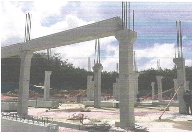
Photo 3.4: Precast beams on site
