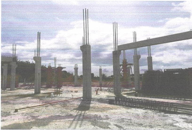
Photo 3.2: Precast columns on site
