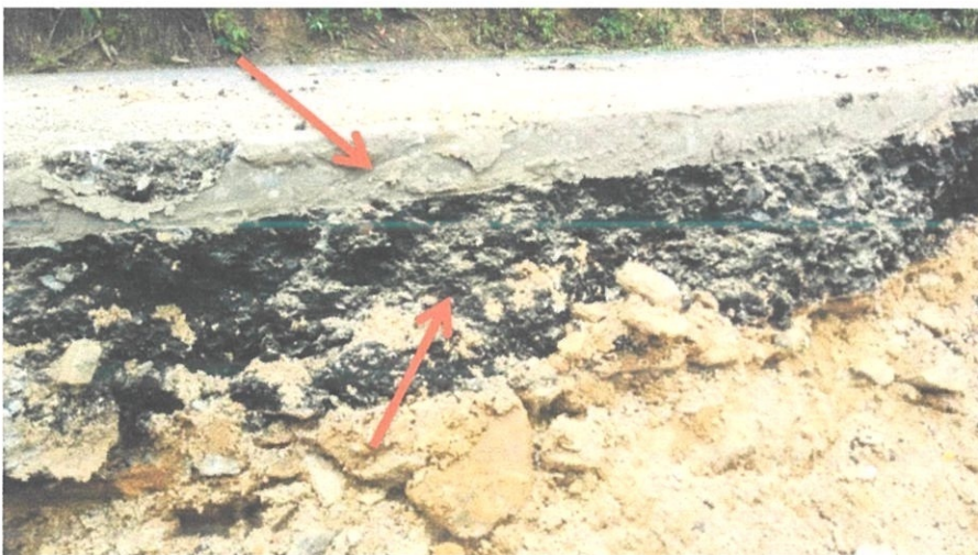
Figure 3.18: The wearing course and binder course layer
