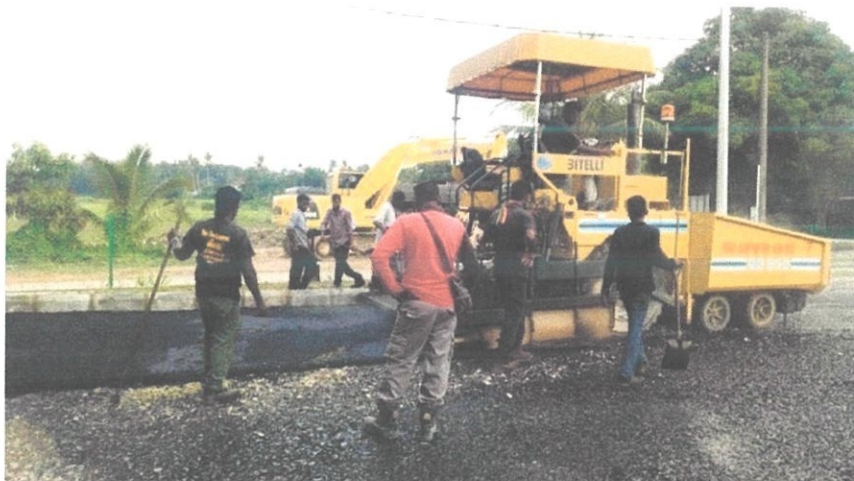
Figure 3.10: Premix binder course is laid onto the ground by pavers
