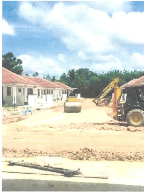
Figure 3.5: Compacting sand bedding process using steel roller
