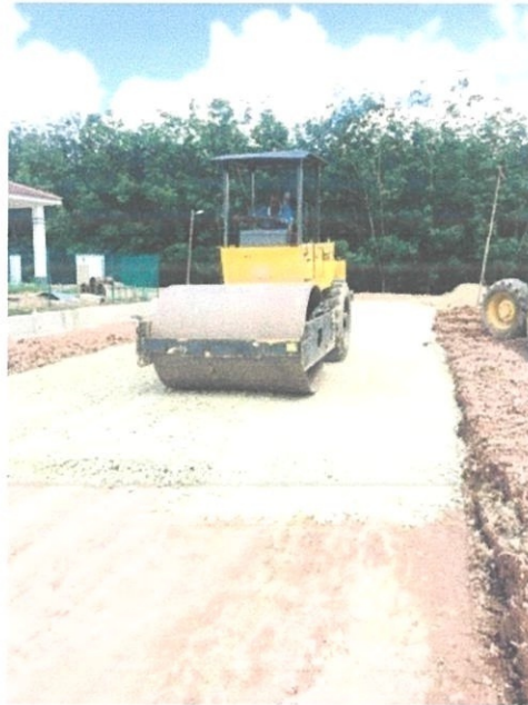
Figure 3.6: Compacting crusher run material using steel roller
