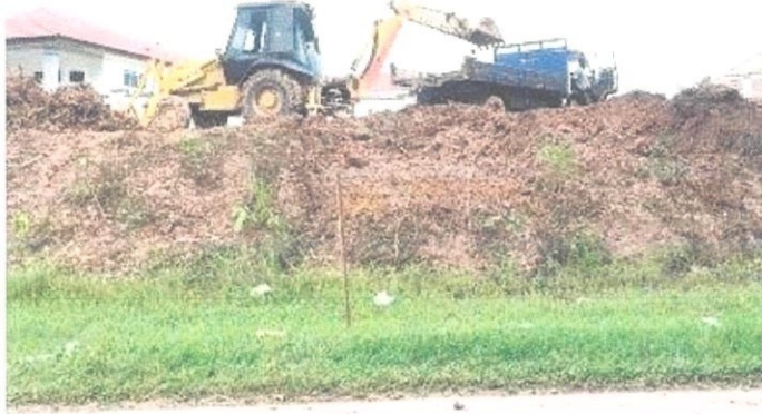
Figure 3.3: Excavation for slope
