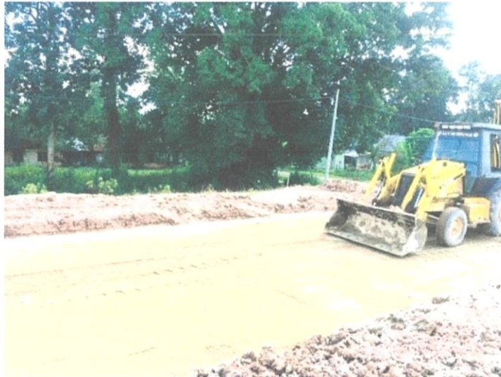
Figure 3.4: Sand bedding laying process
