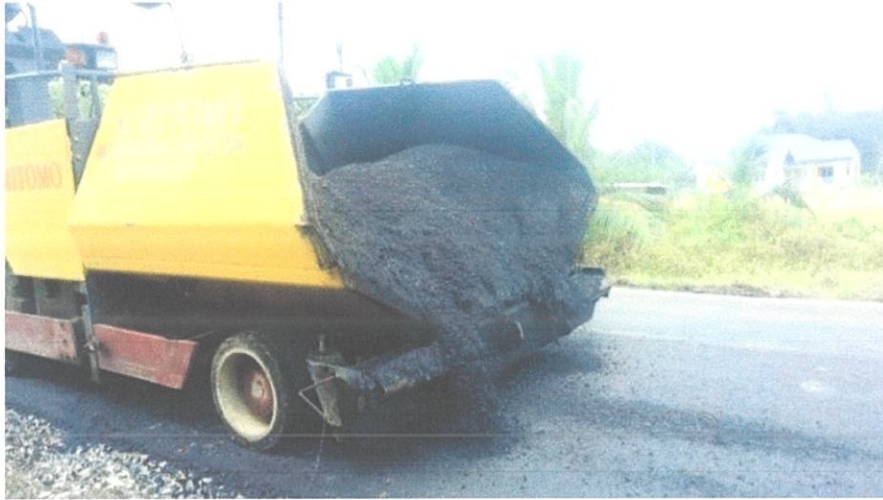
Figure 3.11: Premix wearing course is laid onto the ground by asphalt paver
