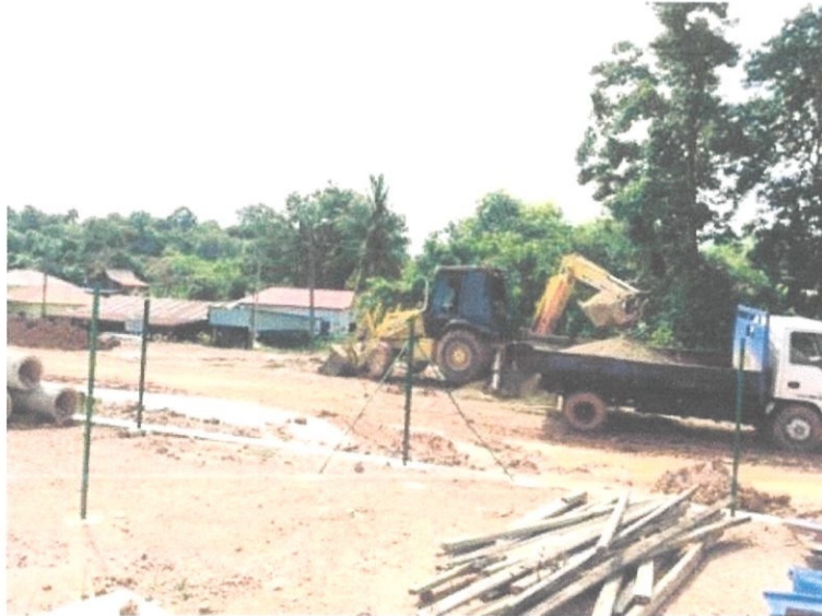
Figure 3.2: Excavation to remove undergrowth roots
