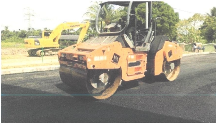
Figure 3.12: Compacting the premix wearing course using steel roller.
