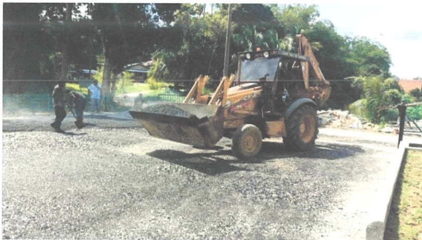
Figure 3.9: Process of laying premix on the ground
