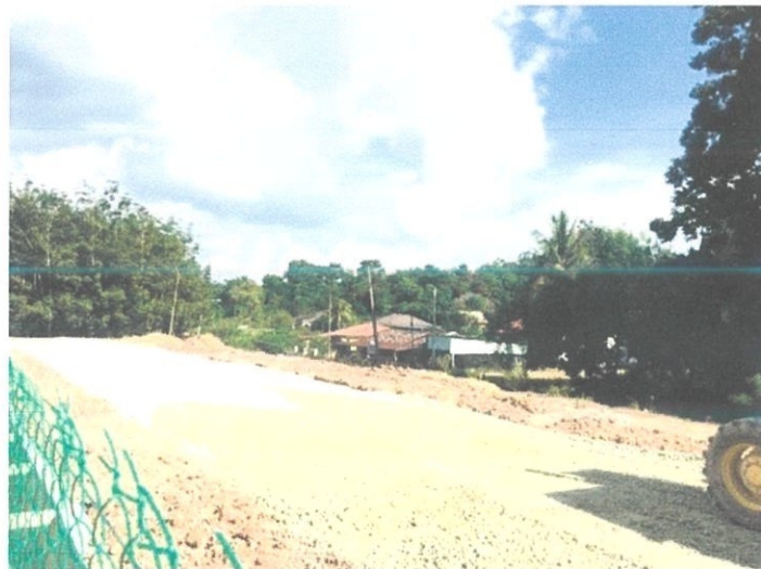
Figure 3.7: Crusher run that have been compacted
