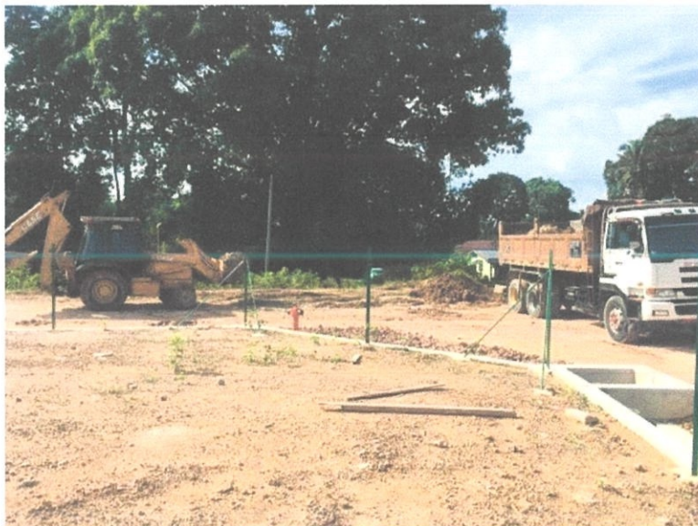
Figure 3.1: Site clearance process
