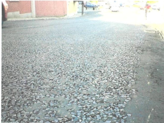
Figure 3.19: The road base layer
