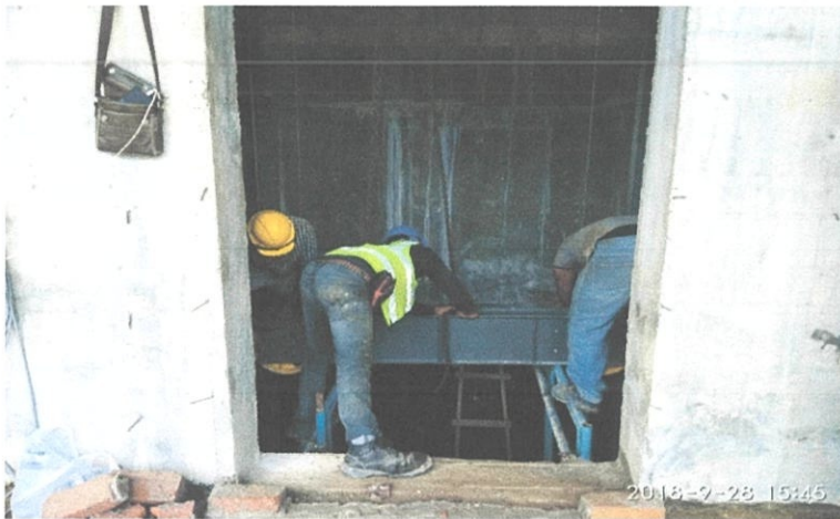
Photo 3.1: Counterweight frame and Guide rail center
