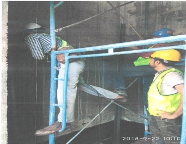
Photo 2.9: Mounting main bracket and counterweight rail process
