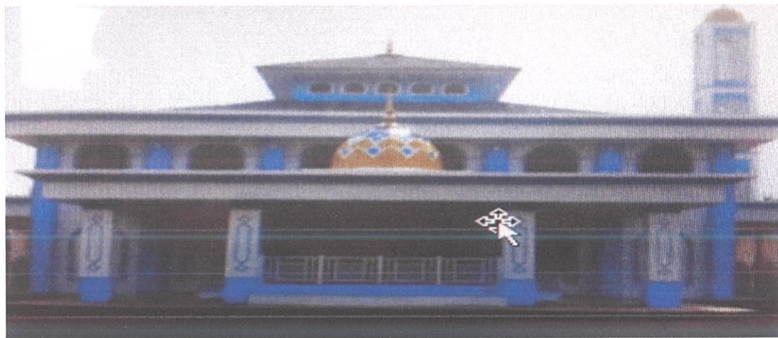
Figure 3.1 : The completed of Kampung Murni Jaya Mosque, Kulaijaya
