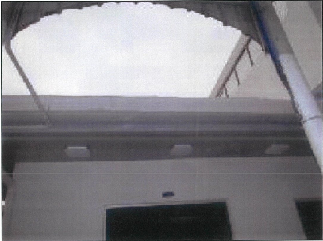
Figure 3.10: Re-Painted Gutter Brackets
