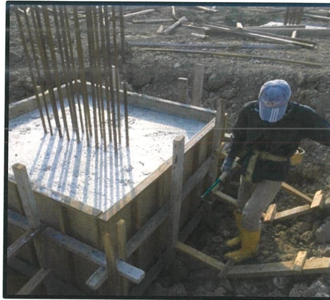
Figure 3.16: The removal of pile cap formwork
