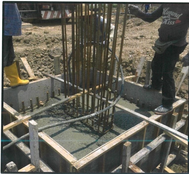
Figure 3.15: Concreting and vibrating works
