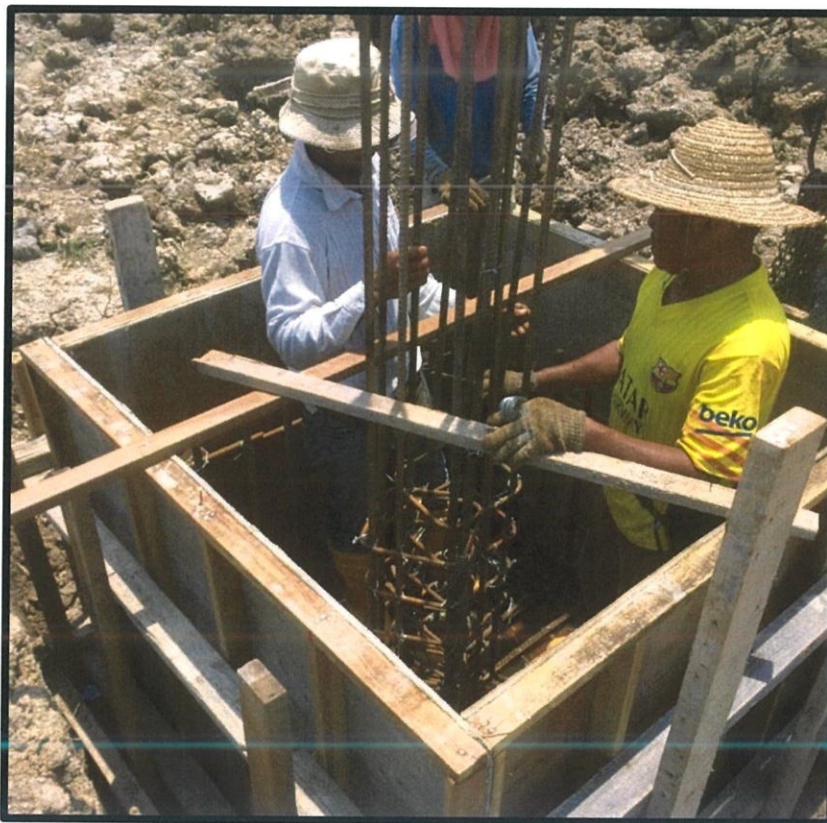
Figure 3.14: Installation of reinforcement bar for pile cap
