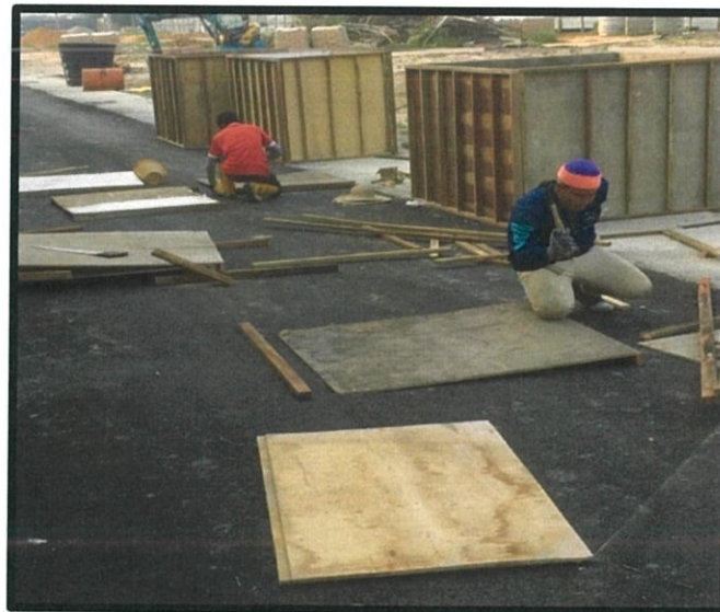
Figure 3.12: The workers are doing the pile cap formwork
