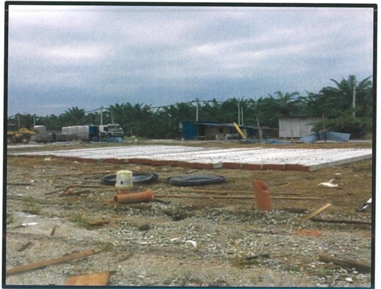
Figure 3.8: The reinforced concrete of piles
