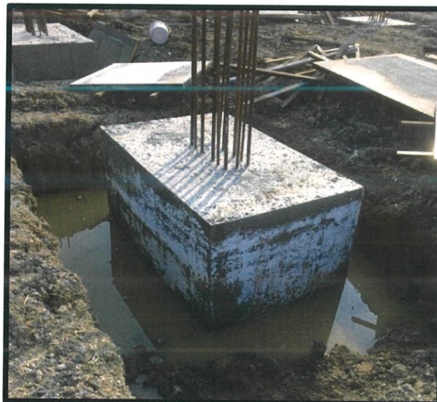
Figure 3.17: Curing process for pile cap
