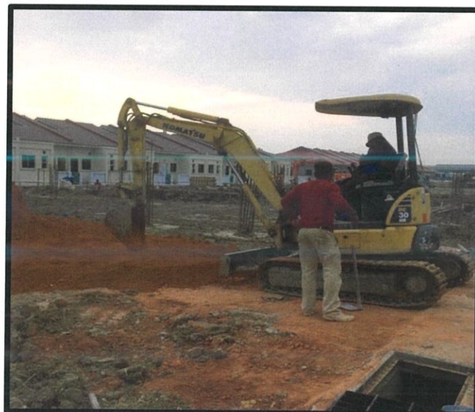
Figure 3.18: The backfilling process of pile cap
