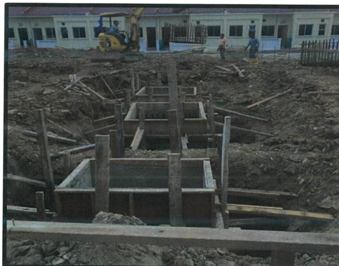
Figure 3.13: Installation of pile cap formwork
