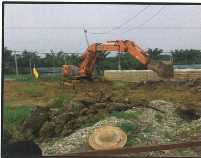
Figure 3.10: Excavation work into the ground
