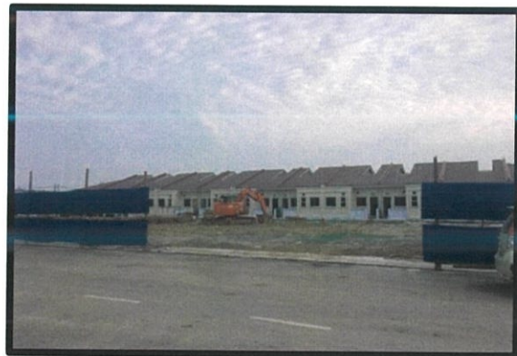
Figure 3.2: The construction site for three-storey shophouse at Taman Emas
