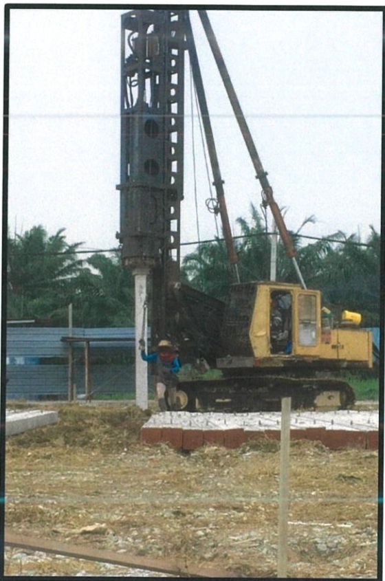
Figure 3.7: Hammering process of piles
