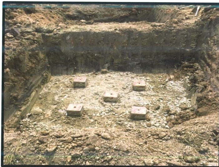
Figure 3.11: Excavation works done with the piles driven into the ground
