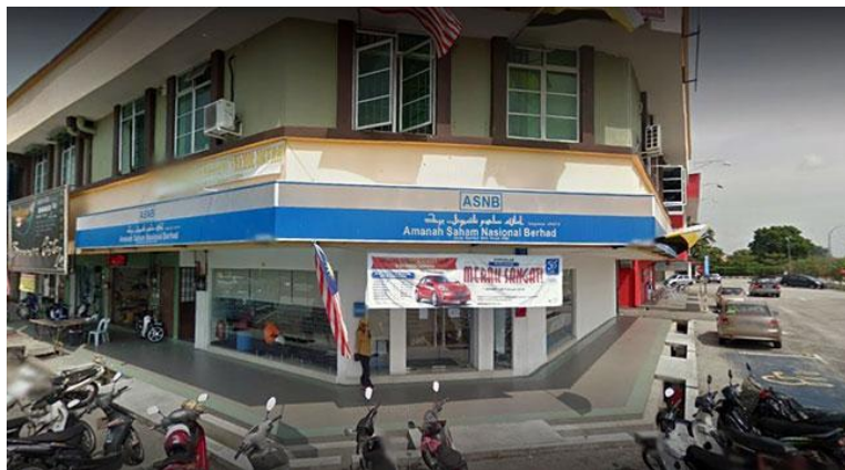
View of ASNB Teluk Intan
