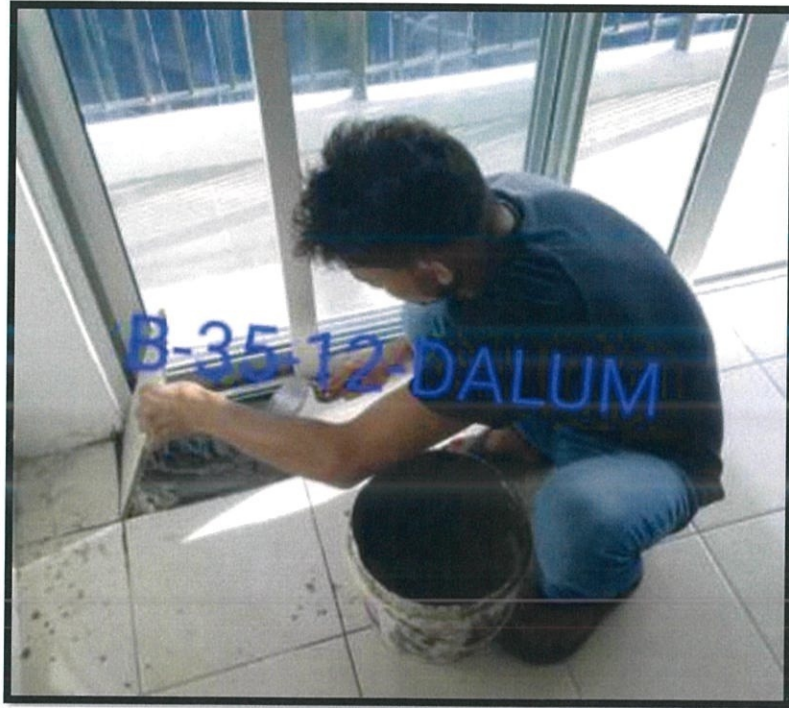
Figure 22 Applying mortar on floor and tile
