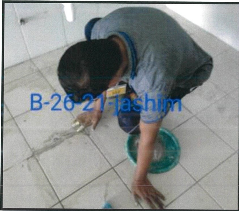
Figure 26 Apply grout on tiles
