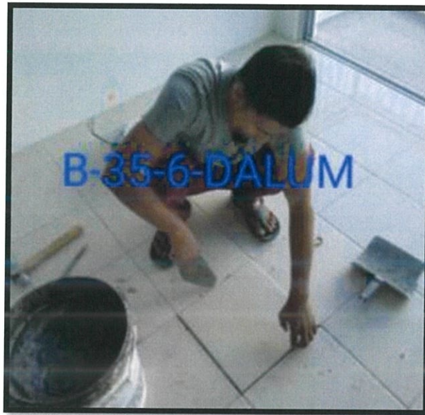
Figure 23 Placing tiles
