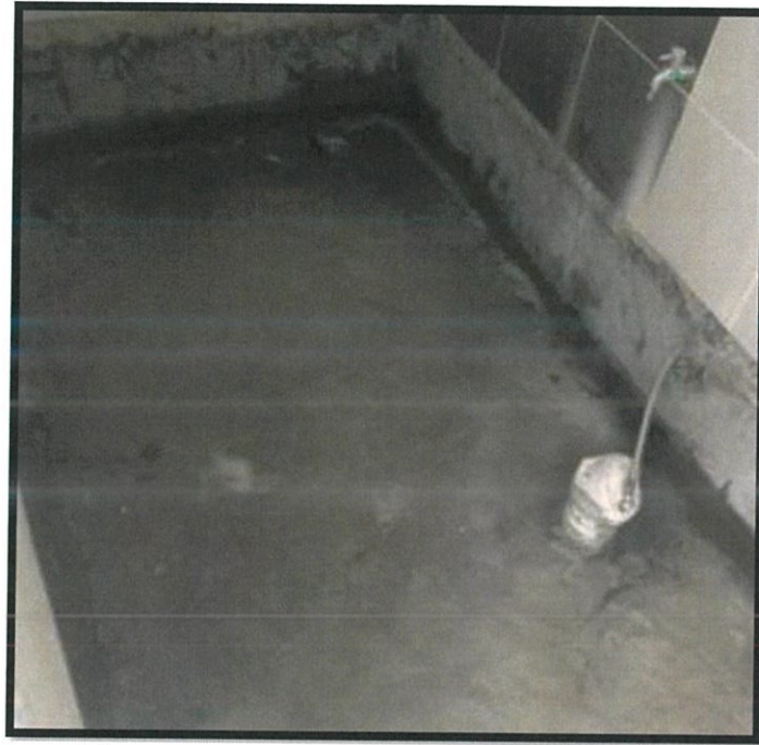
Figure 18 Apply water proofing membrane
