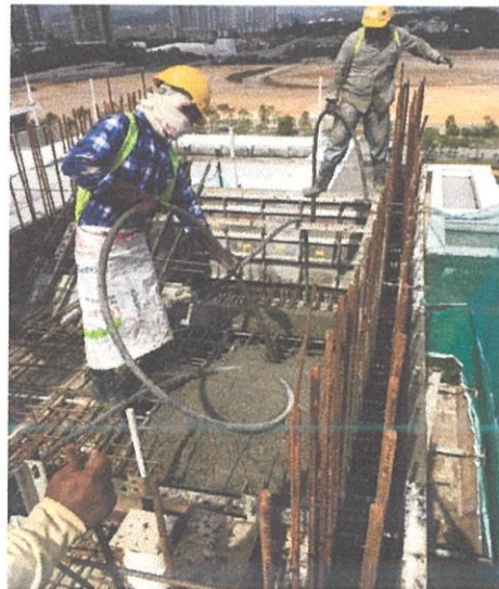
Photos 3.11 : Concreting work at staircase
