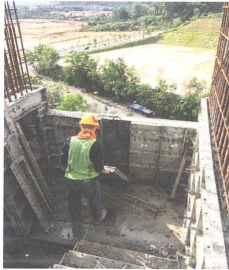
Photos 3.13 : Work of opening the formwork at staircase
