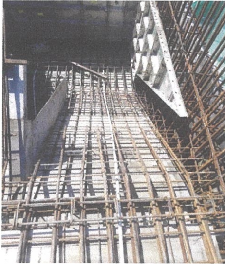
Photos 3.8 : The installtion of wall panel
