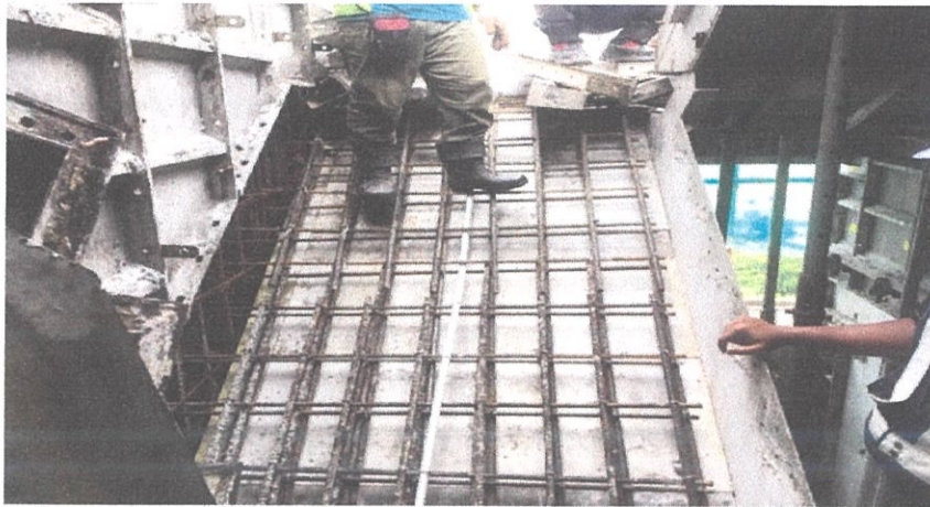
Photos 3.7 : Rebar and electrical pipe that has been installed at staircase.
