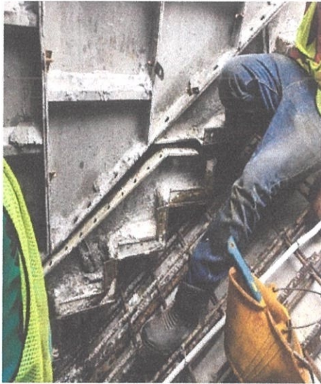
Photos 3.9 : The installation of gun panel
