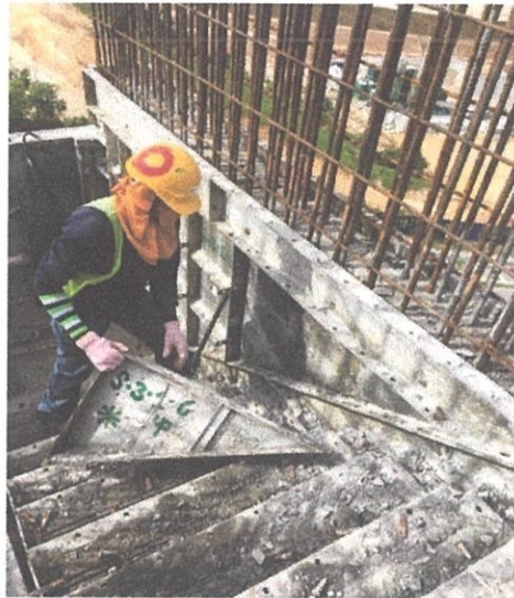
Photos 3.14 : Work of opening formwork at staircase
