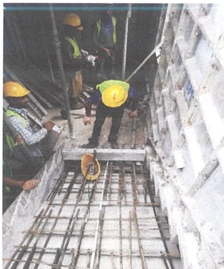
Photos 3.10 : The installation of step panel
