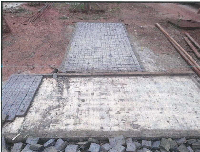
Photo 3.3 : Shows the concrete blocks prepared for reinforcement bar
