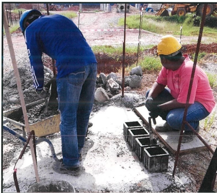
Photo 3.4 : Shows the making of concrete cube for concrete Grade 35
