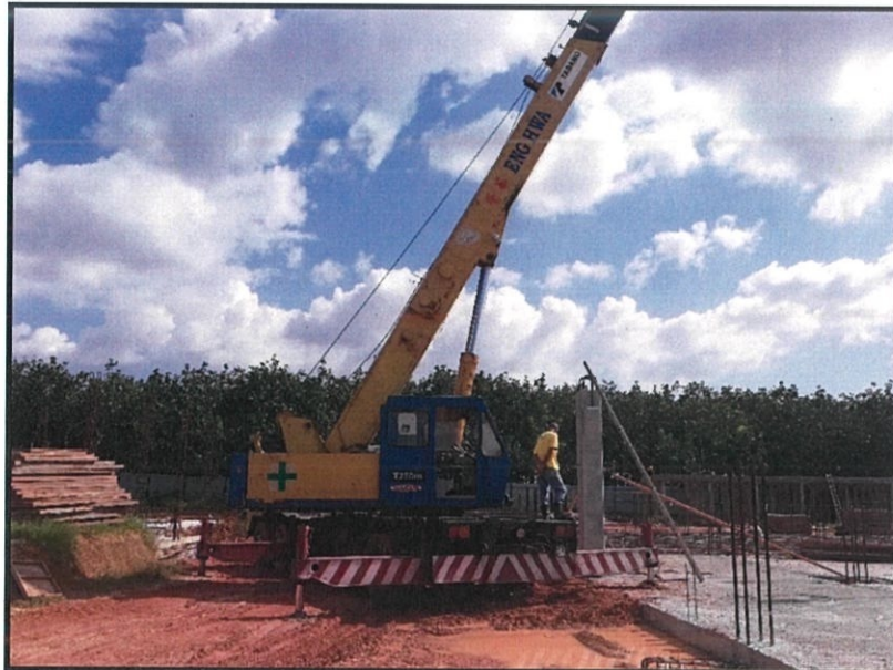
Photo 3.11 : Shows the crane used at the construction site
