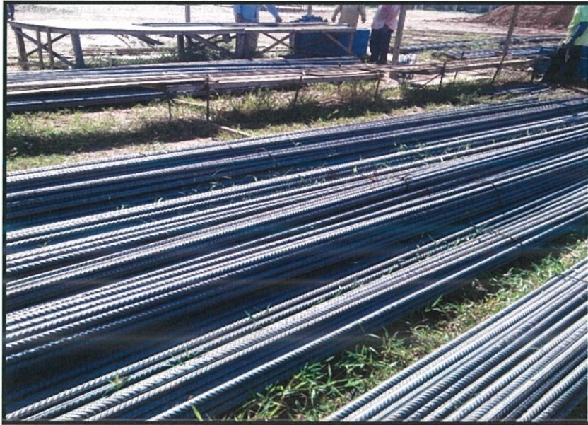
Photo 3.2 : Shows the steel bar prepared to be cut
