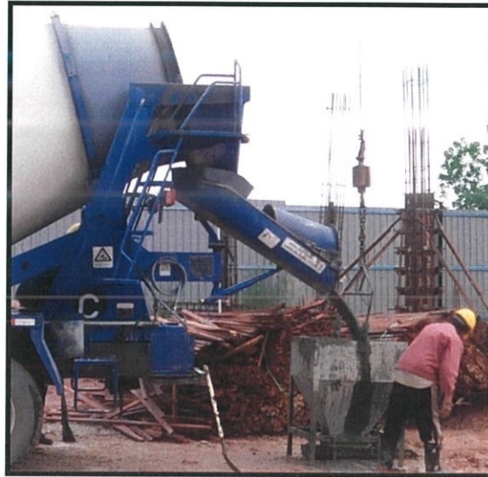
Photo 3.12 : Shows the concrete mixer truck pouring concrete into the bucket
