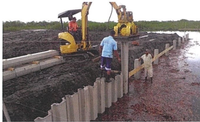
Figure 1.2: Sheet pile. Source: Doug Ingersoll (2012).
