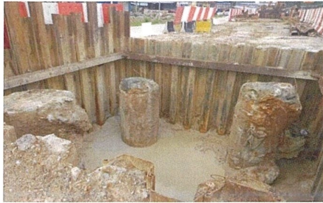
Figure 1.1: Bore pile. Source: Abdul Rohman (2015).
