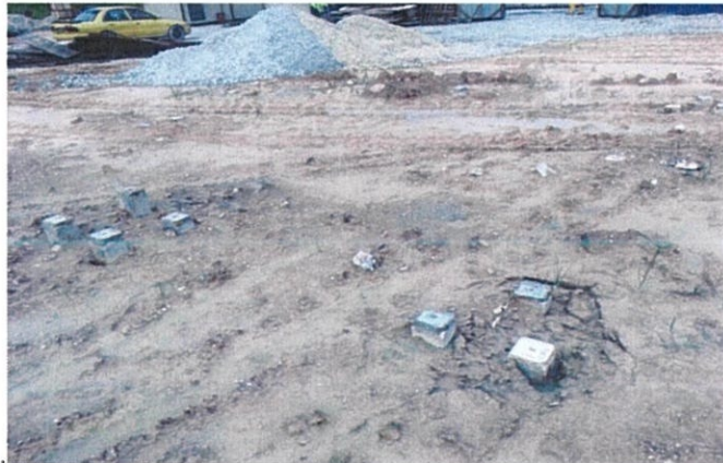
Photo 3.6: The piling points at Water Tank area.
