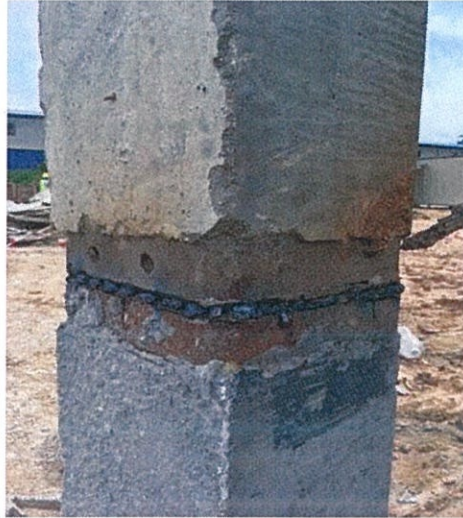
Photo 3.14: Pile joints are completed.
