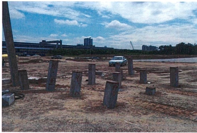
Photo 3.9: The piling points at Toll Canopy area.
