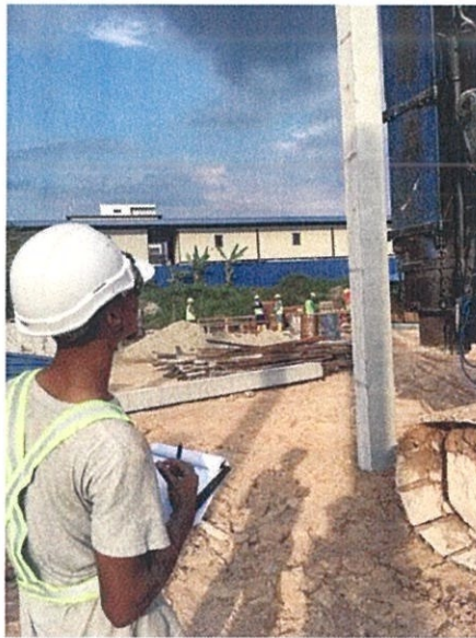
Photo 3.16: A worker was recorded the pile reading.
