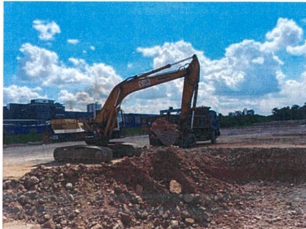
Photo 3.3: Excavator are used to excavate soil at the OSD area.
