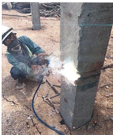
Photo 3.13: Welding process is in process.
