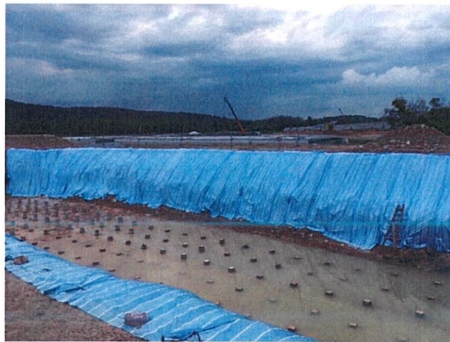
Photo 3.10: The piling points at OSD Tank 1.
