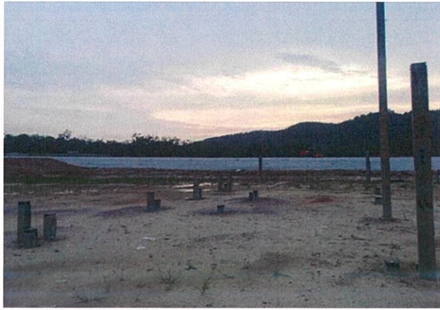
Photo 3.7: The piling points at TNB Substation area.
