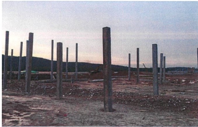
Photo 3.8: The piling points at Maintenance Depot Building area.
