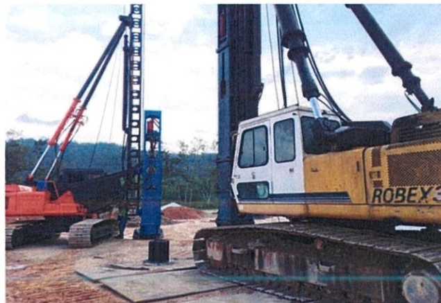
Photo 3.2: Hydraulic piling machine.
