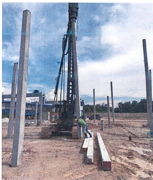
Photo 3.11: A worker was handling the pile.
