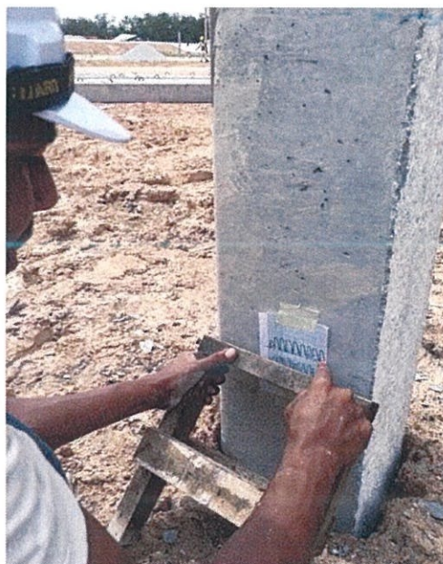
Photo 3.15: A worker was take the blows of set using a graph paper
